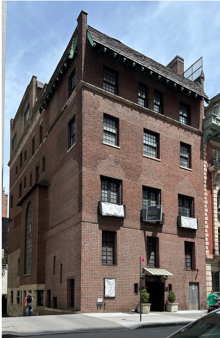
existing facade photo - modified 1926
