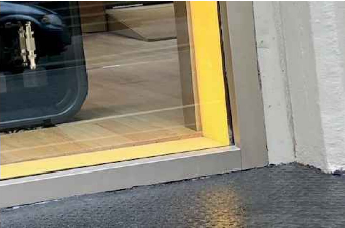
WINDOW FRAMES SILL FROM EXTERIOR
