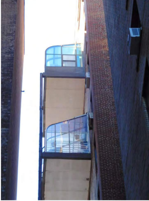
Existing Conditions 11B
