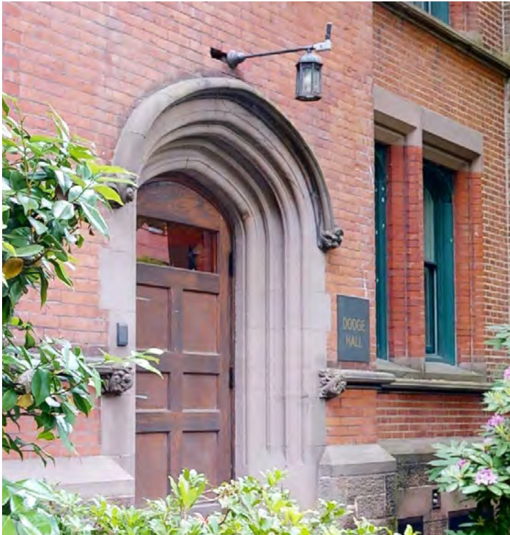
TYPICAL RESIDENTIAL FIXTURE TO BE RESTORED, ARM RETURNED TO HISTORIC CONDITION
