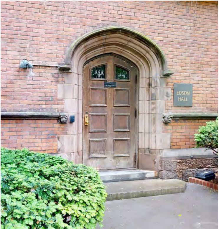
MANY DOORS DO NOT HAVE ANY HISTORIC FIXTURES & NEED TO MEET CODE REQUIRED LIGHT LEVELS - NEW FIXTURE TO MIMIC HISTORIC RESIDENTIAL FIXTURE
