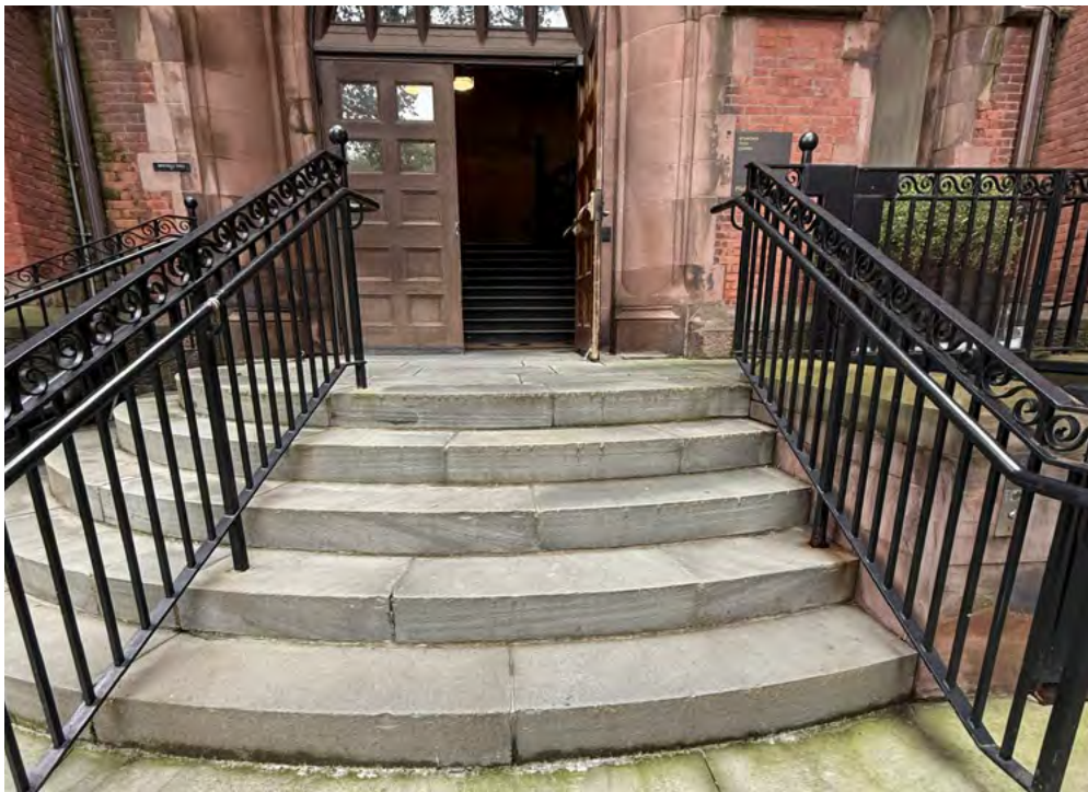
REBUILT STOOP AND GUARDRAILS, HOFFMAN HALL
