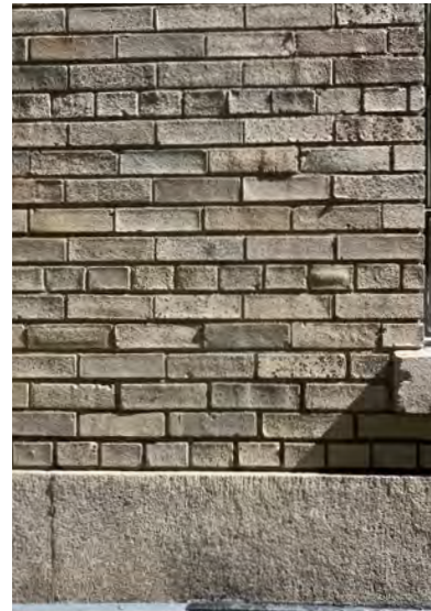
2. Brick and Granite water table
