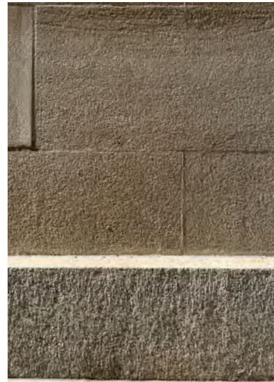
2. Brick and Granite water table
