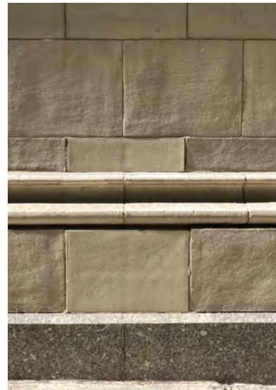
2. Brick and Granite water table
