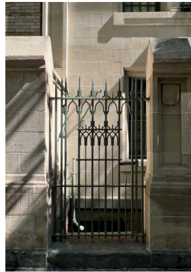
2. Metal Gate and Granite water table
