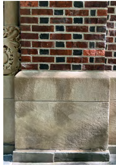
2. Brick and Granite water table
