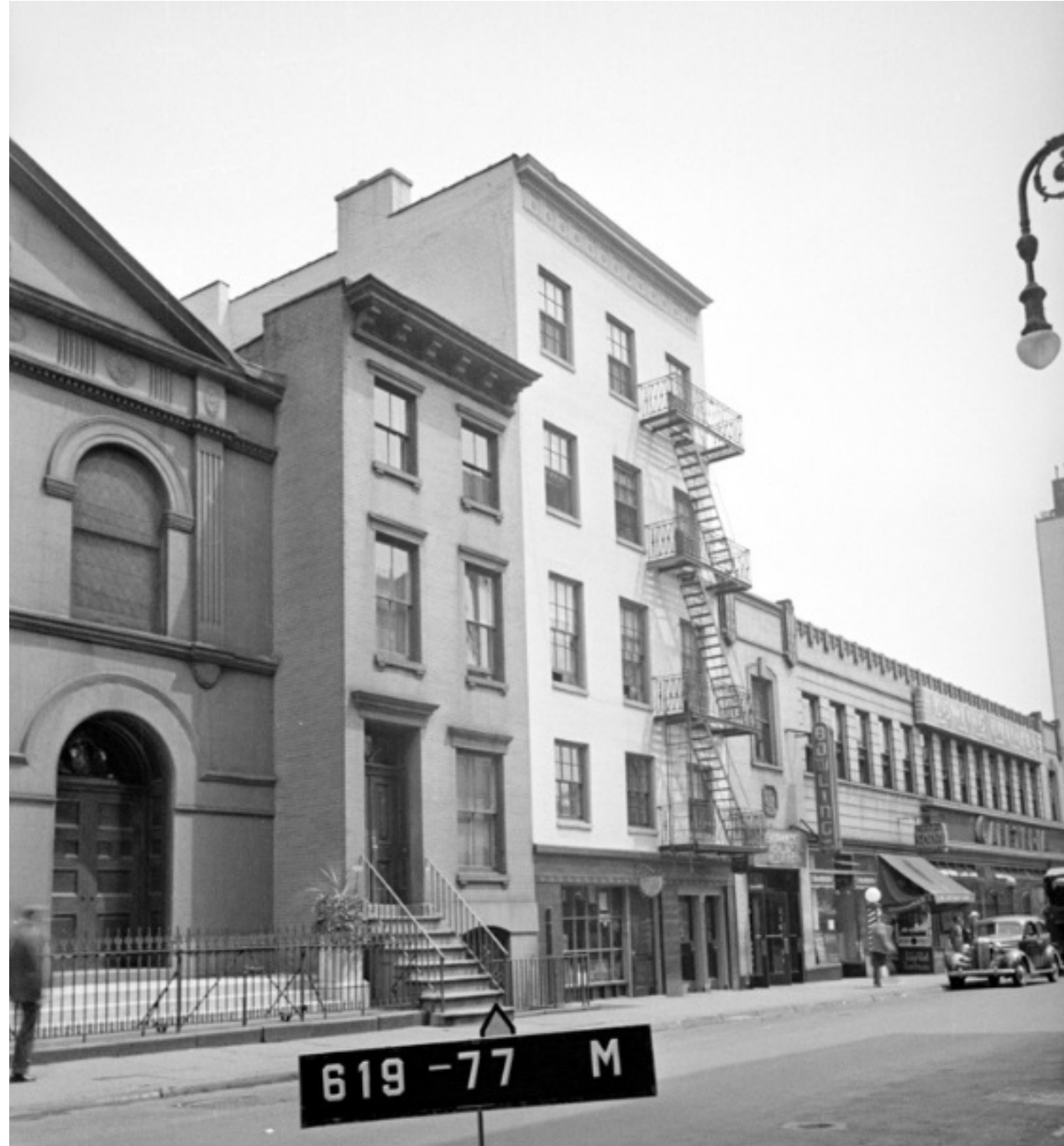
CHRISTOPHER STREET VIEW - BUILDING FRONT (c1940)
