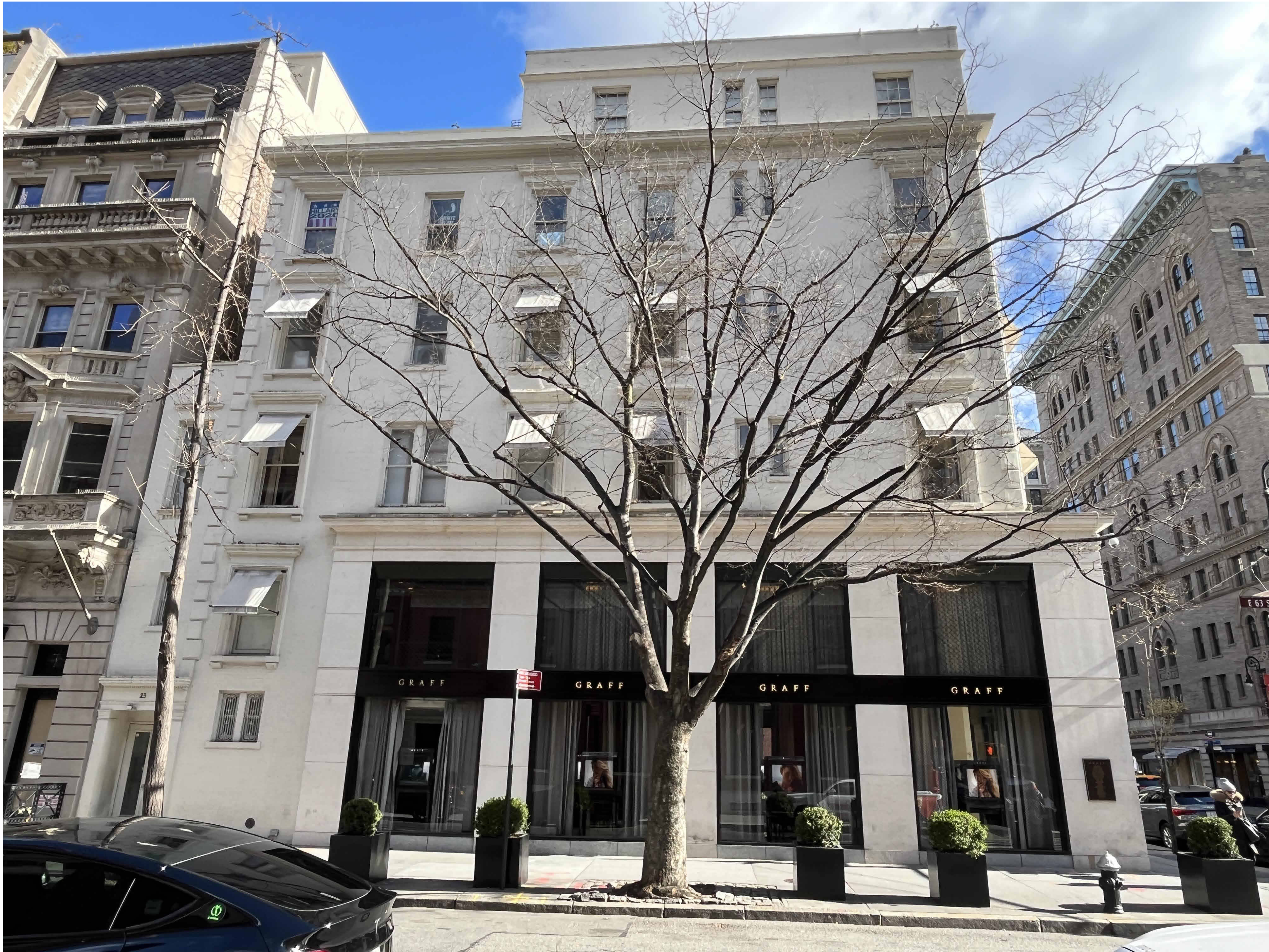
View of East 63rd Street elevation.
