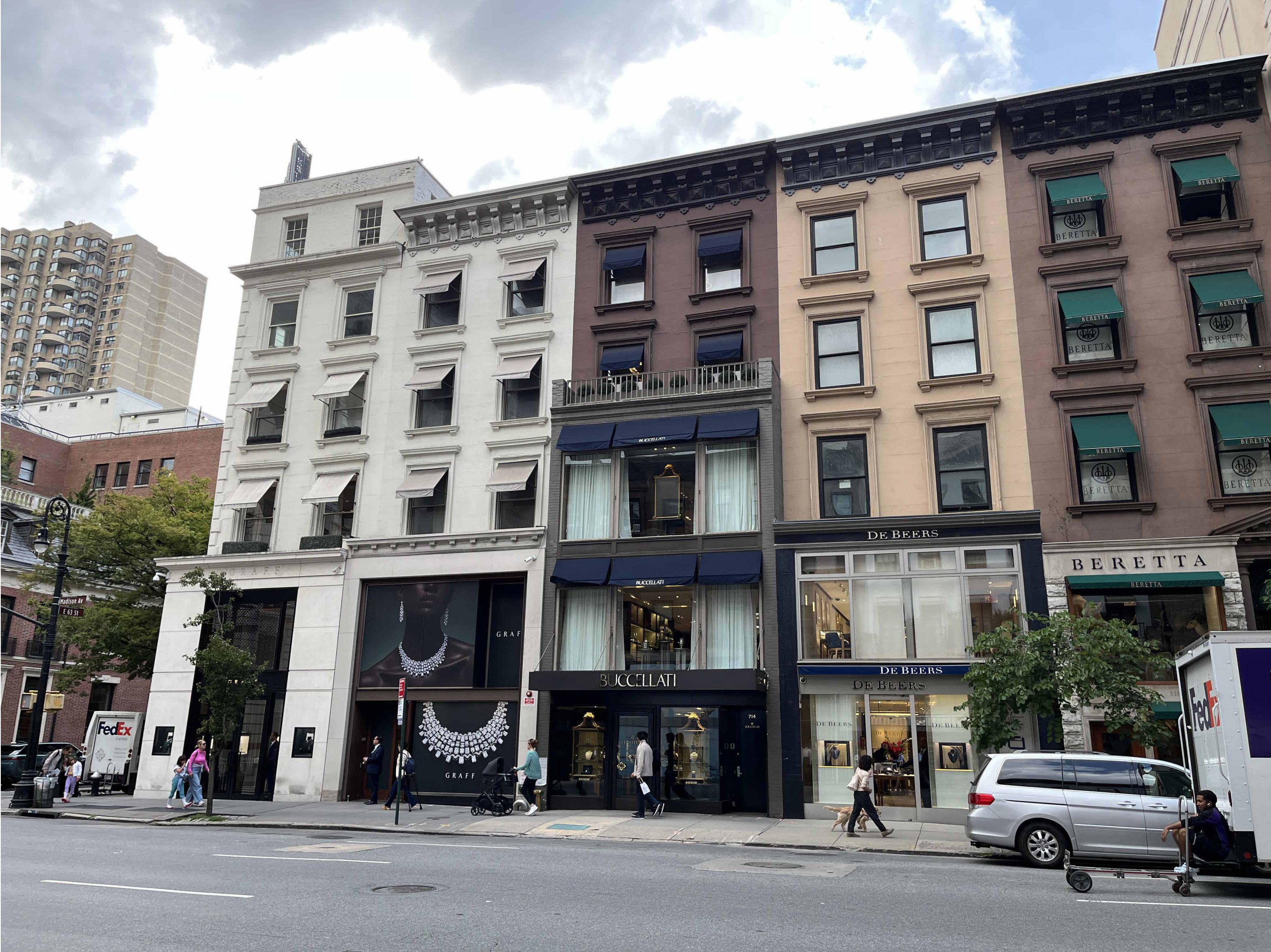
View of blockfront, looking southwest.
