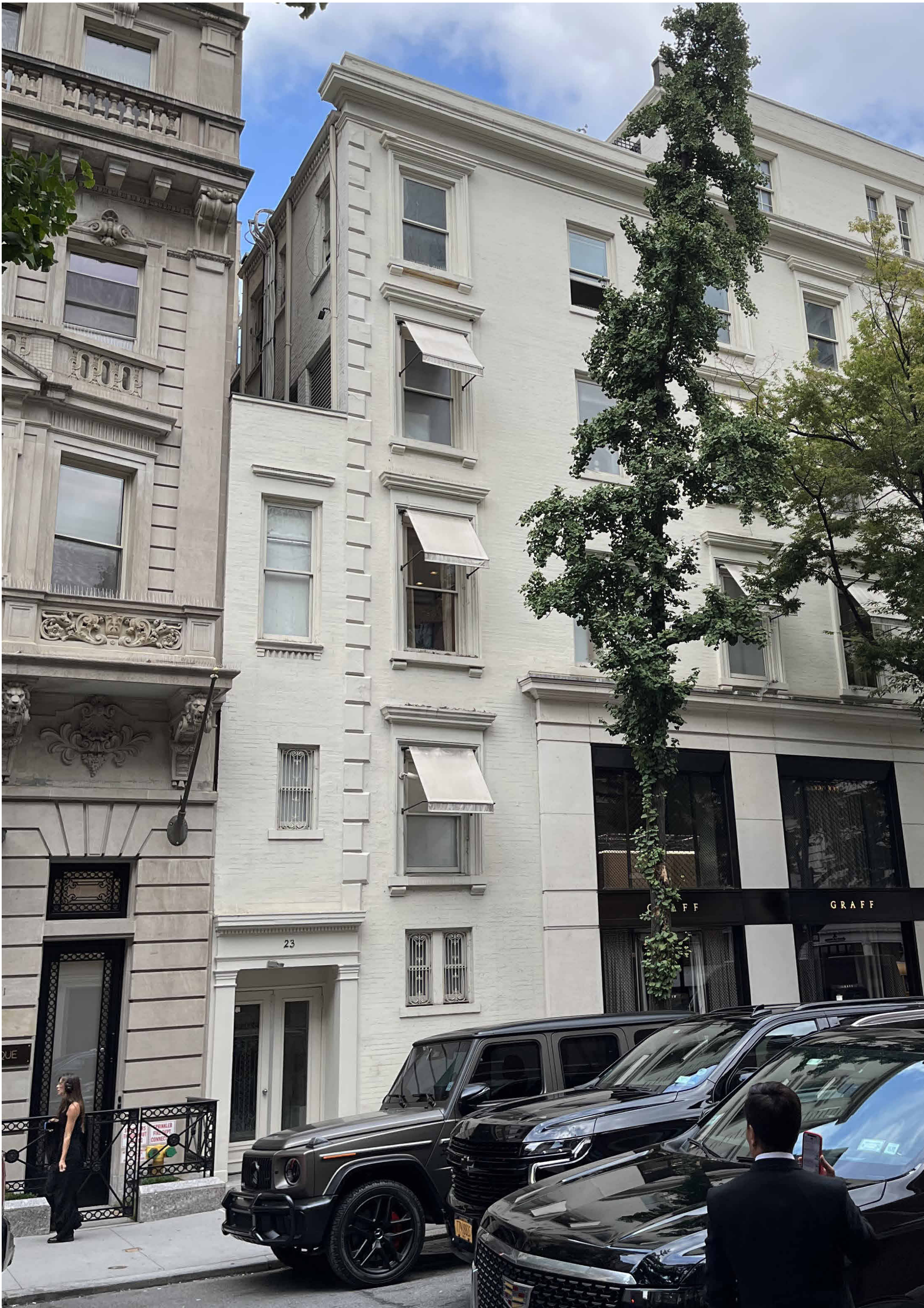
View to partially visible rear of 710 Madison Ave. Rear of 712 is not visible.
