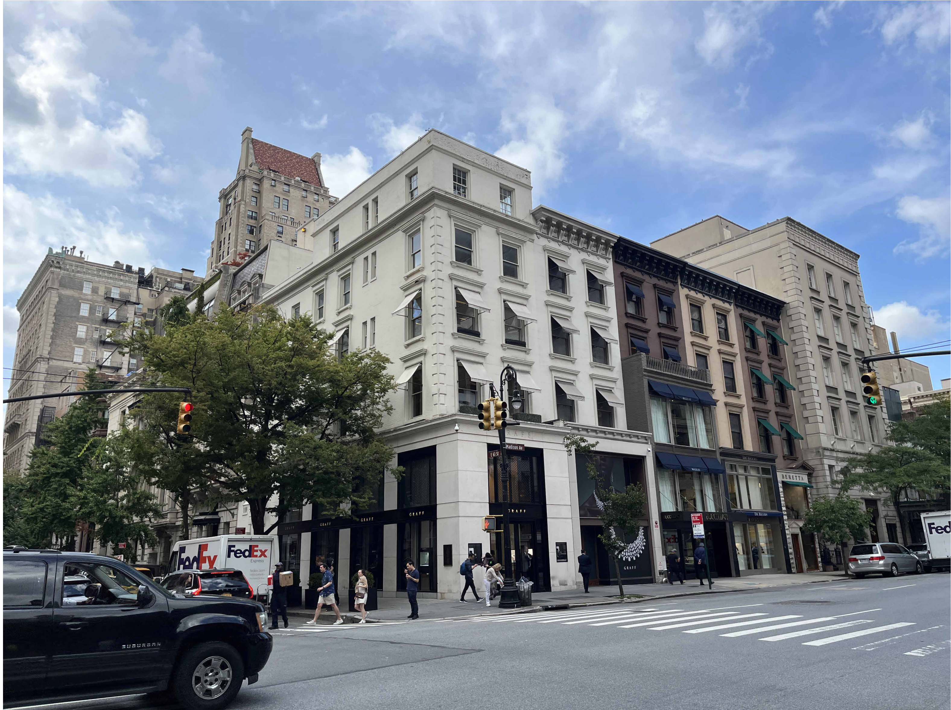
View of blockfront, looking northwest.
