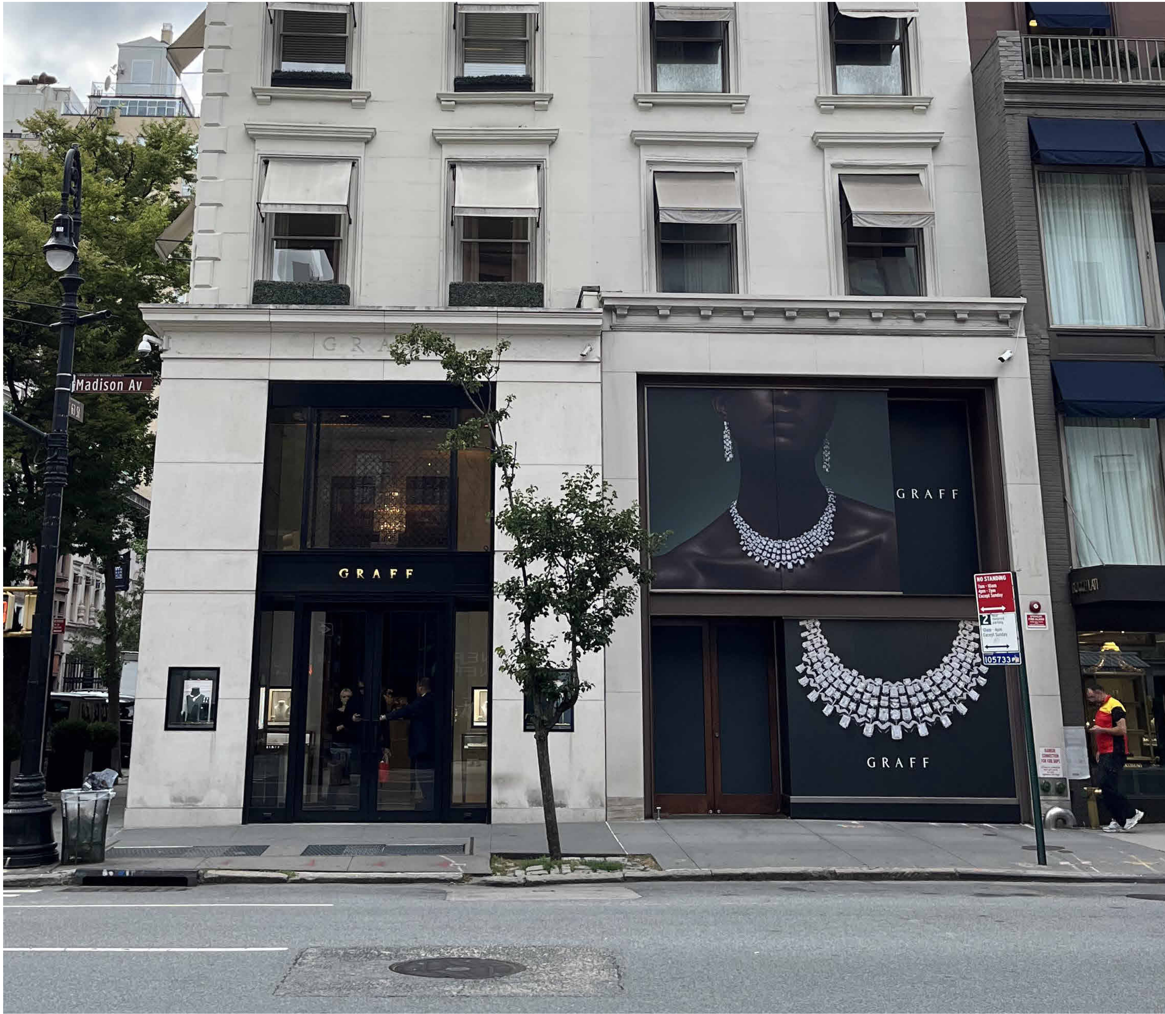
Overall view of 710 and 712 Madison Avenue two-story storefronts.
