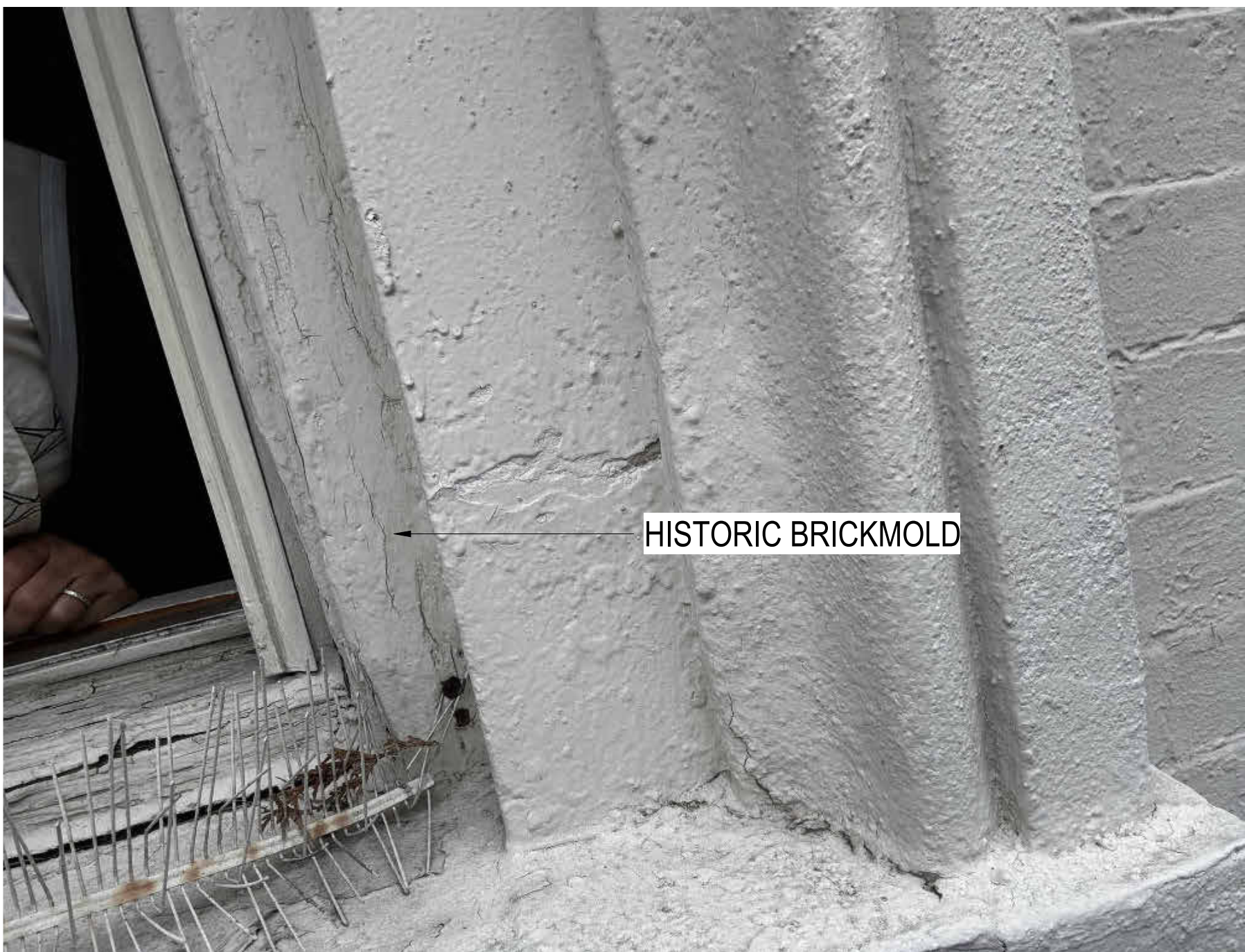
EXISTING CONDITIONS PHOTOGRAPH SHOWING BRICKMOLD
