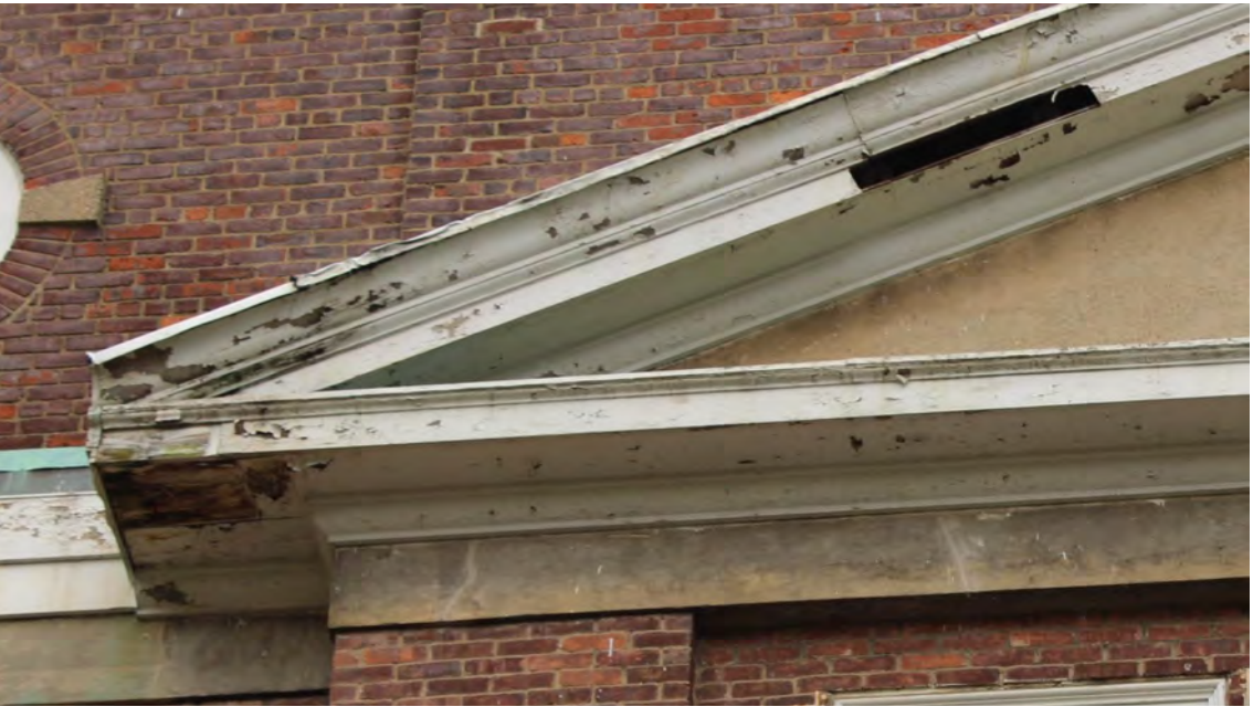
REPLACED MISSING AND DETERIORATED WOOD ELEMENTS
