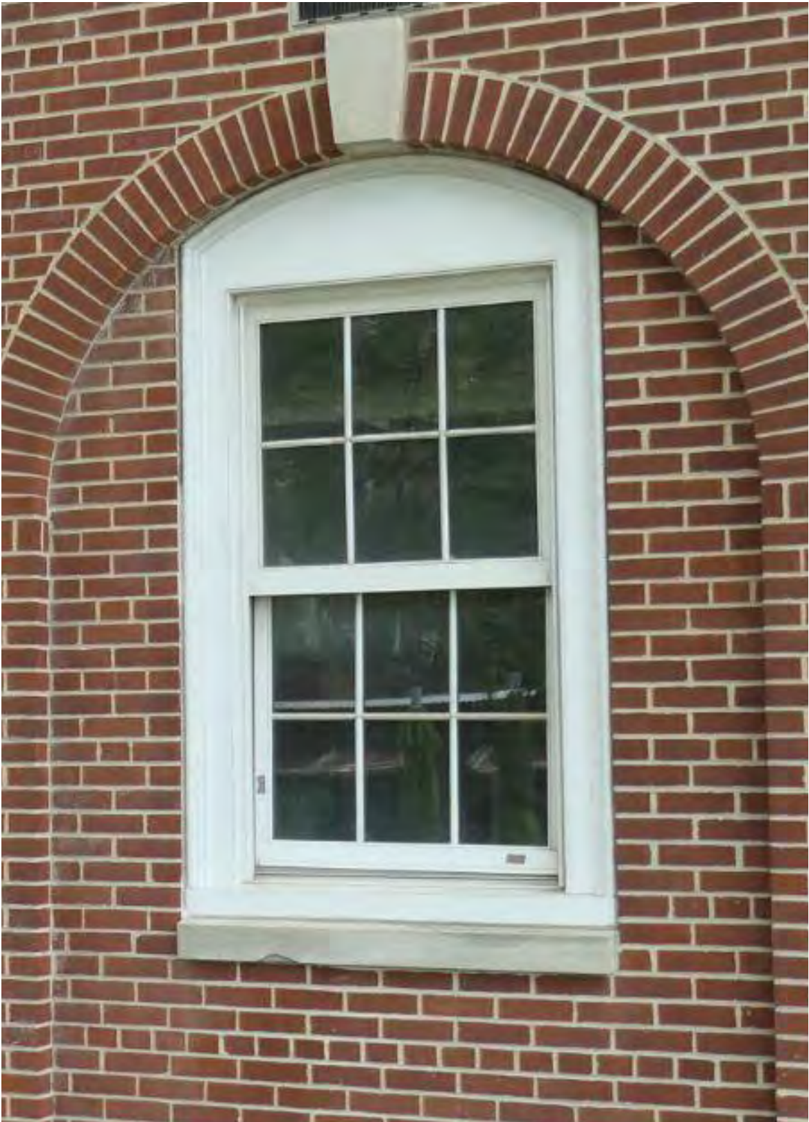
EXISTING - SQUARE-HEADED WINDOW WITHIN ARCHED OPENING
