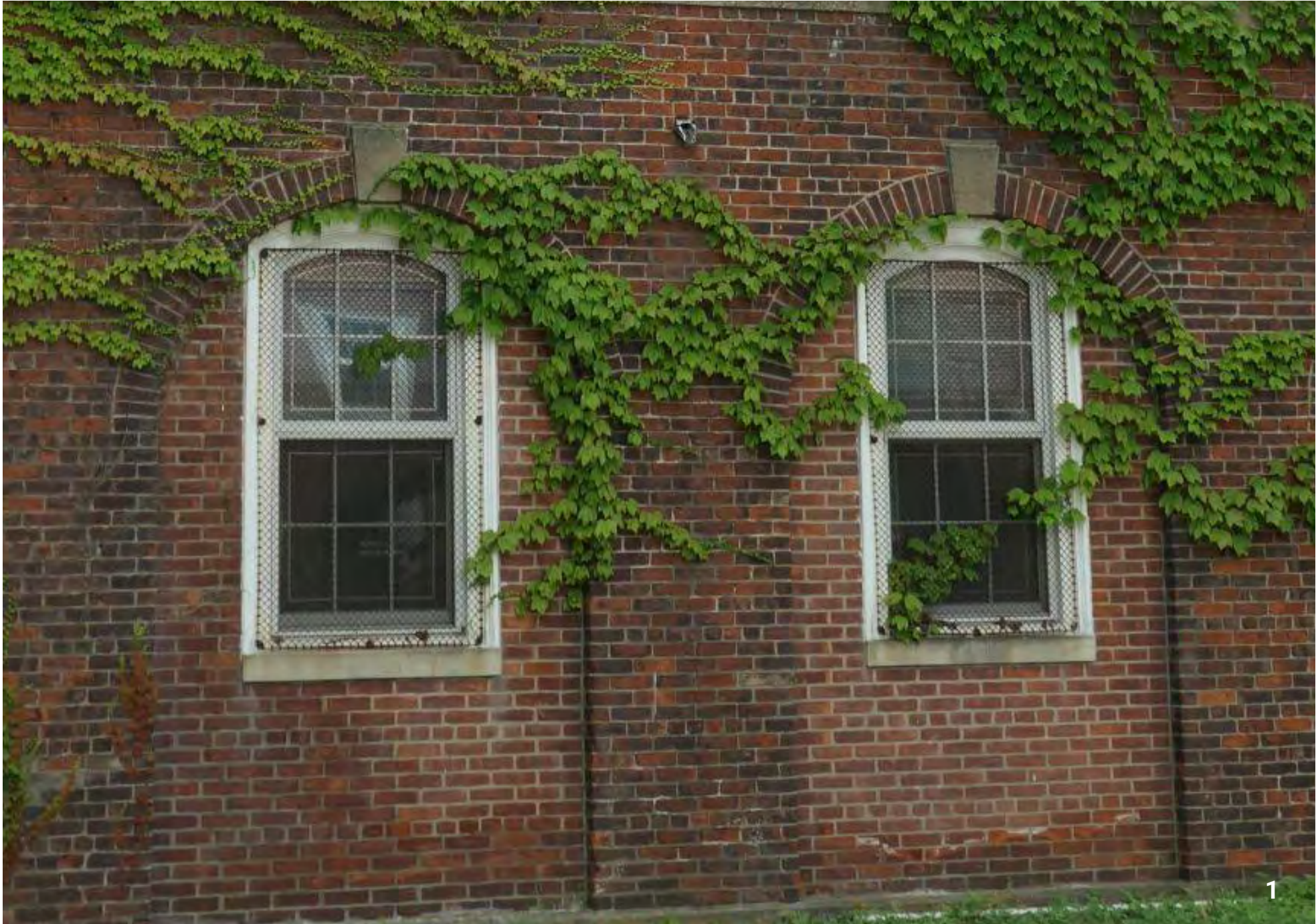
DETAIL OF NON-HISTORIC BRICK AND WINDOWS IN INFILLED ARCADE
