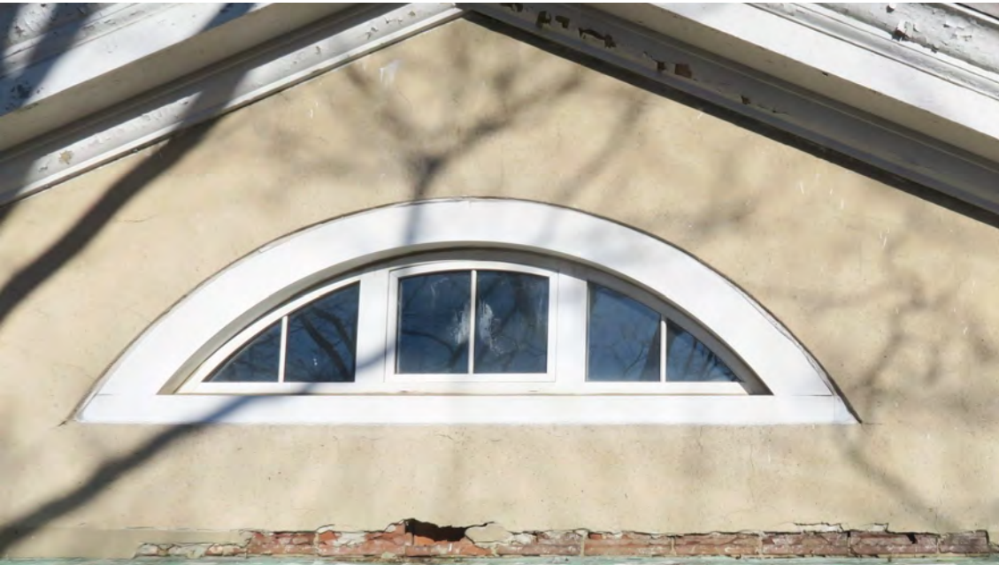
REPLACE DETERIORATED STUCCO TO MATCH EXISTING
