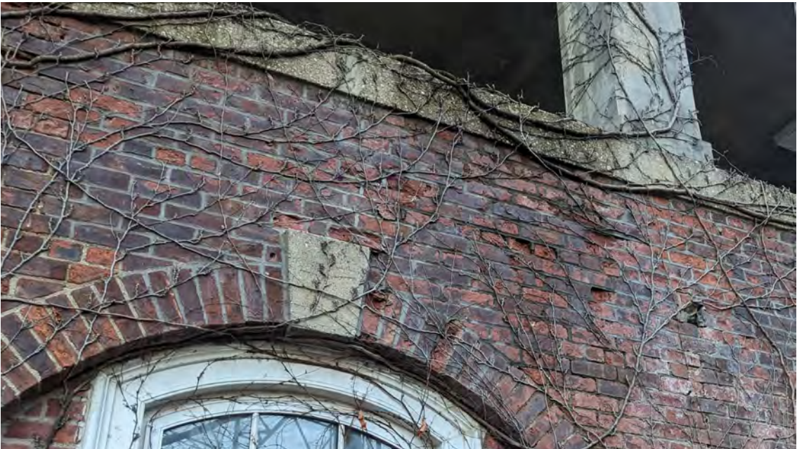
REPLACE DETERIORATED BRICK WITH NEW BRICK TO MATCH EXISTING
