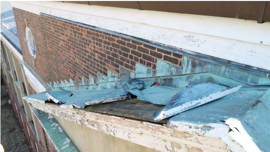
REPLACE DETERIORATED FLASHING TO MATCH EXISTING
