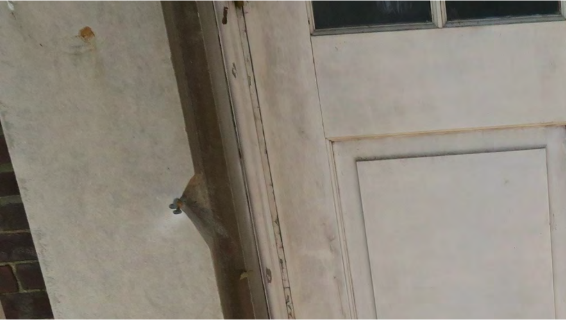
REPAIR SPALLED STONE WITH STONE DUTCHMAN REPAIRS
