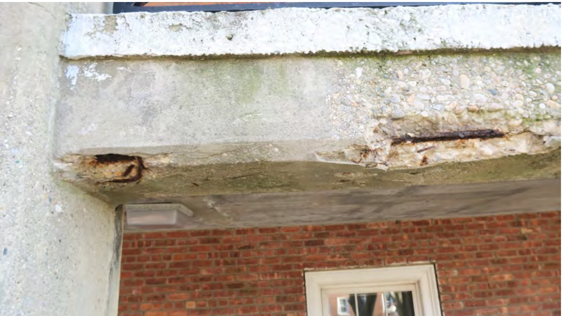
PATCH SPALLED CONCRETE
