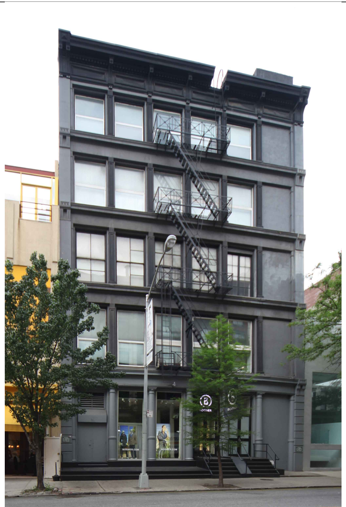
03 2010 LPC DESIGNATION PHOTO NTS
