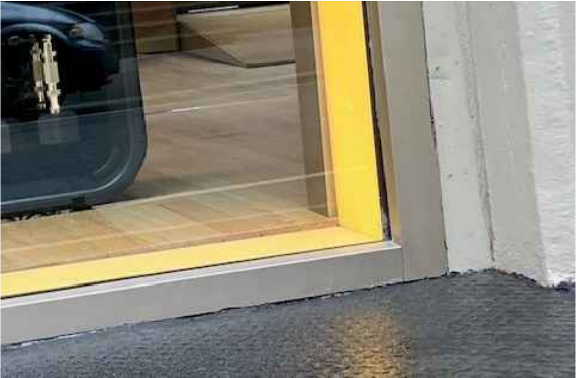
WINDOW FRAMES SILL FROM EXTERIOR
