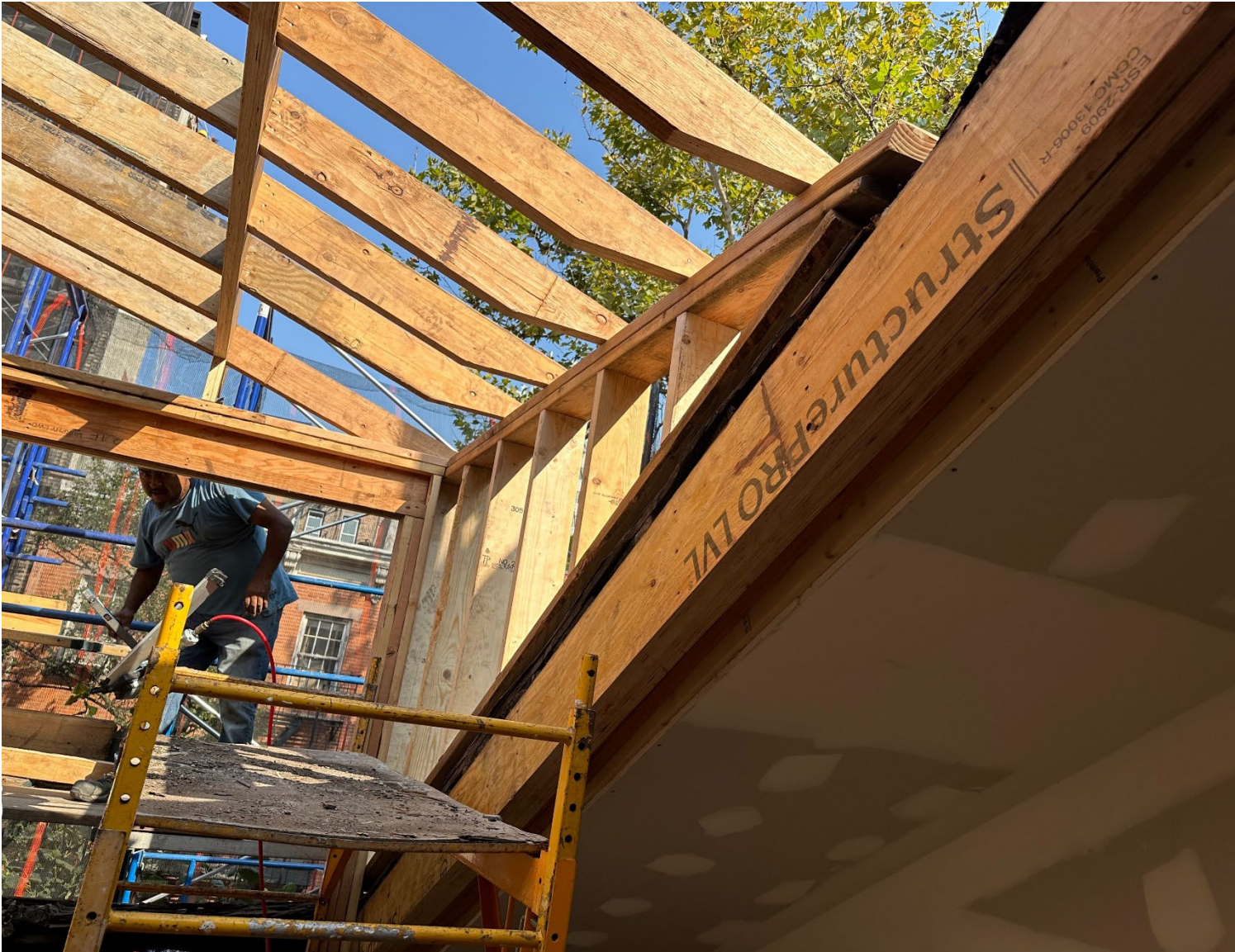
Reconstruction of dormer Sides of dormers are placed on the structural headers
