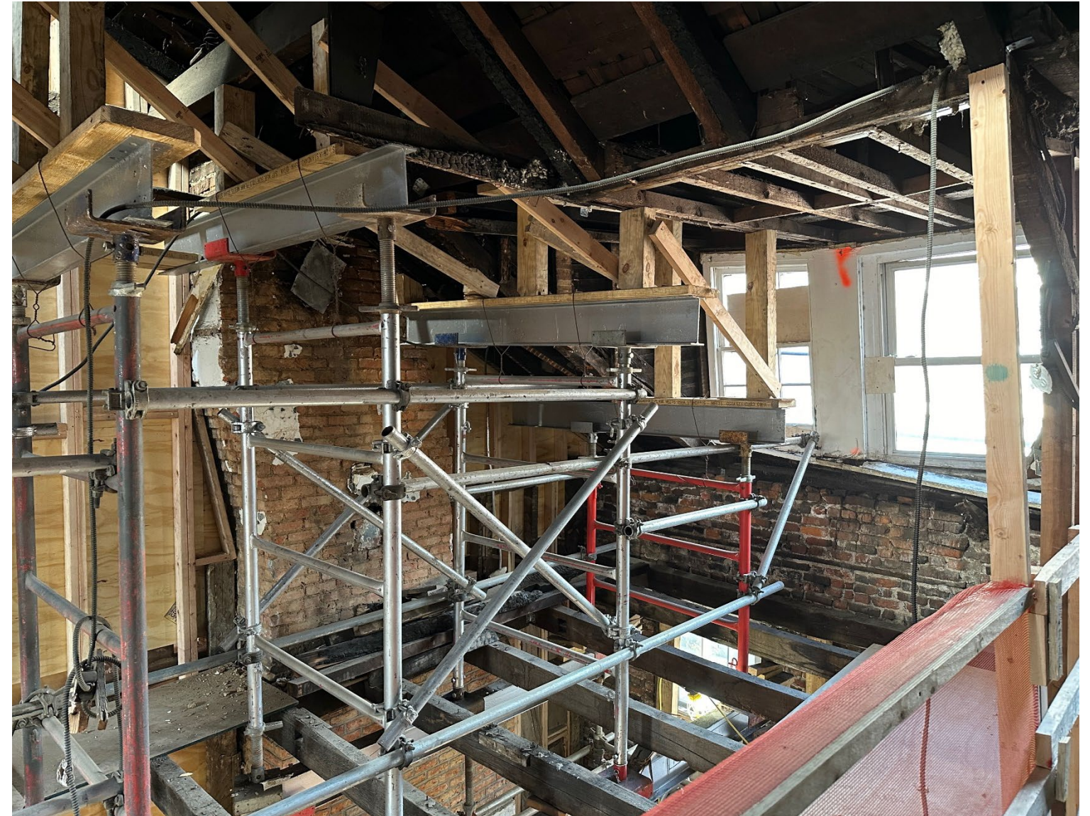
Interior Dormer 18 Christopher St With necessary shoring, building structure severely compromised
