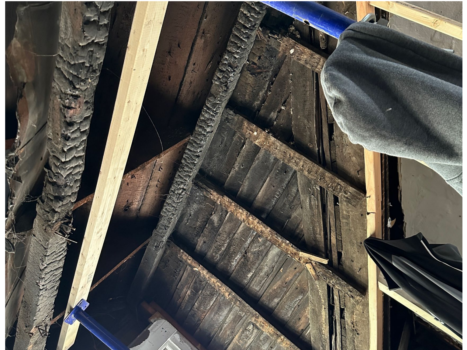
Burned Interior Dormer 20 Christopher St from multiple fires throughout the years
