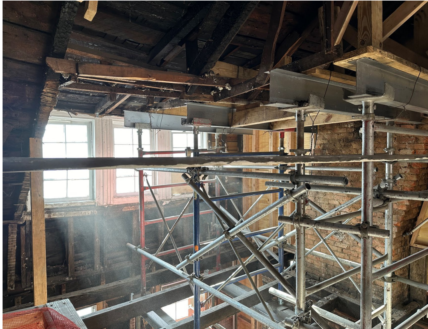
Interior Dormer 20 Christopher St With necessary shoring, building structure severely compromised
