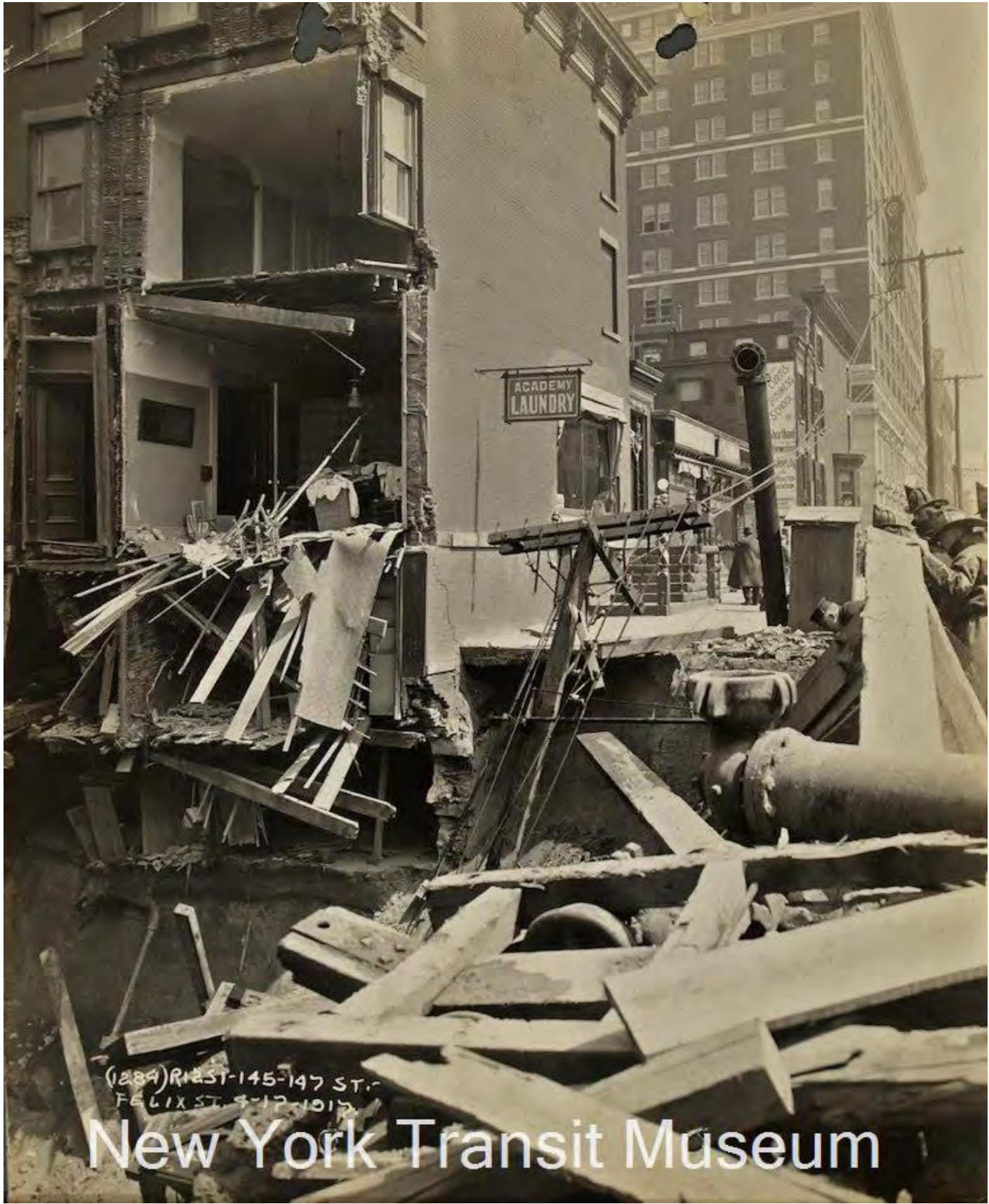
Shows condition of fronts of buildings 145 and 147 St. Felix Street after cave-in. The camera is set at the northwest corner of Hanson Place and St. Felix Street, looking east.
