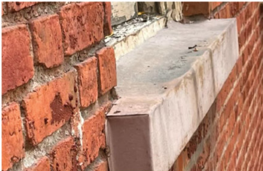
Sill Covered in Break Metal
