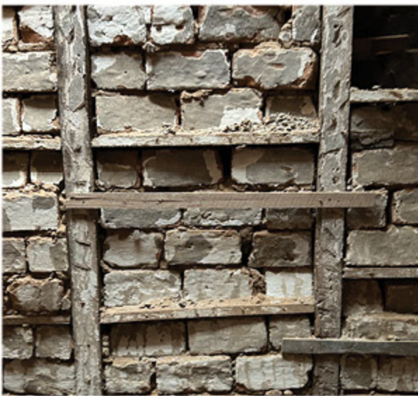
Decay of brick nogging wall, including loose brick and rot at original structural timbers
