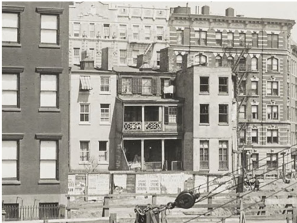
50 Charles Street (1916) Source: NYHS
