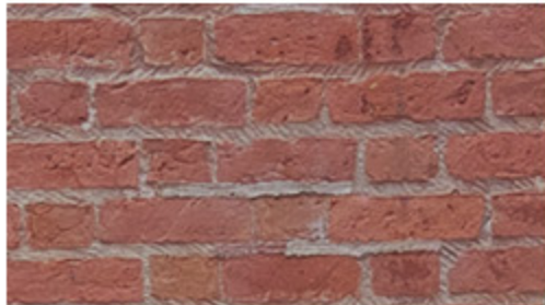
Existing Restored Brick 85 Sullivan Areaway
