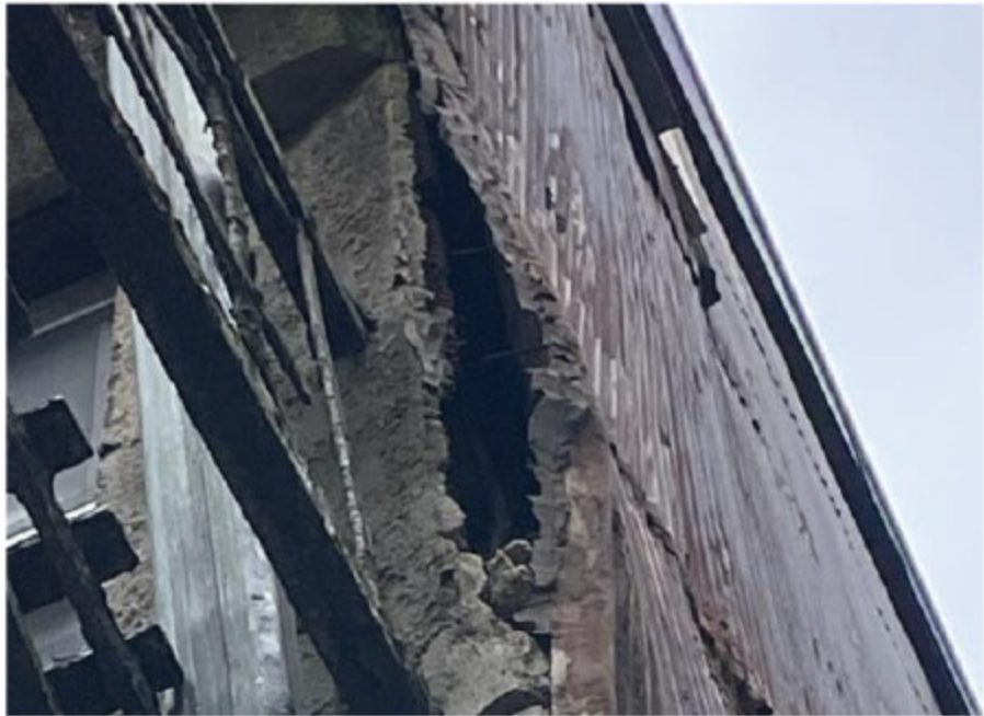
Buckling Wall Separation of the north and east wall, source of considerable water infiltration
