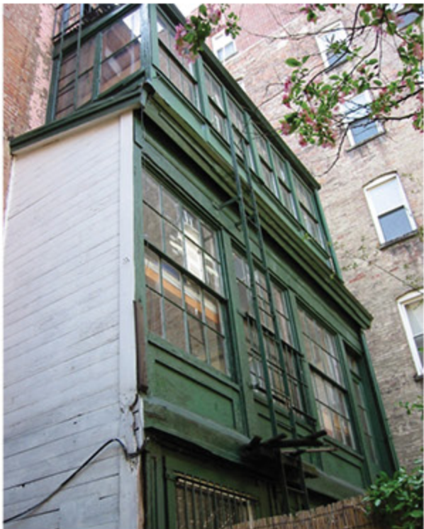
235 W 11th Street (built 1844)
