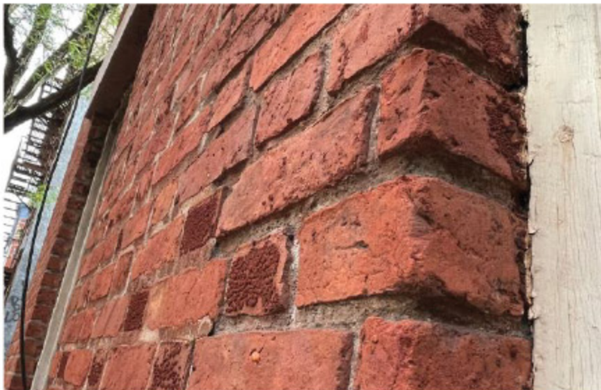
Mortar Erosion
