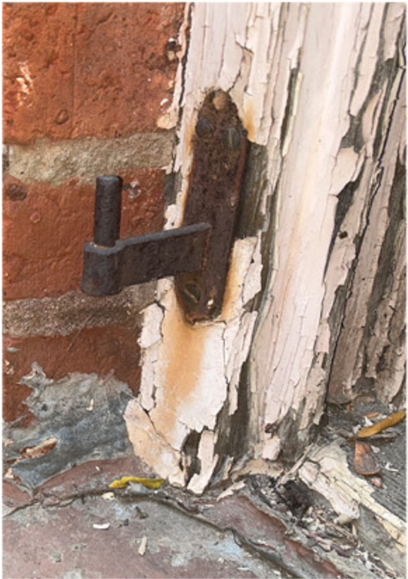
Existing Shutter Pintle Visible at 10 windows, 83 and 85 Sullivan
