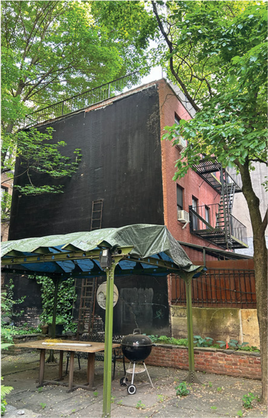
Existing Rear Building at 81 Sullivan Street
