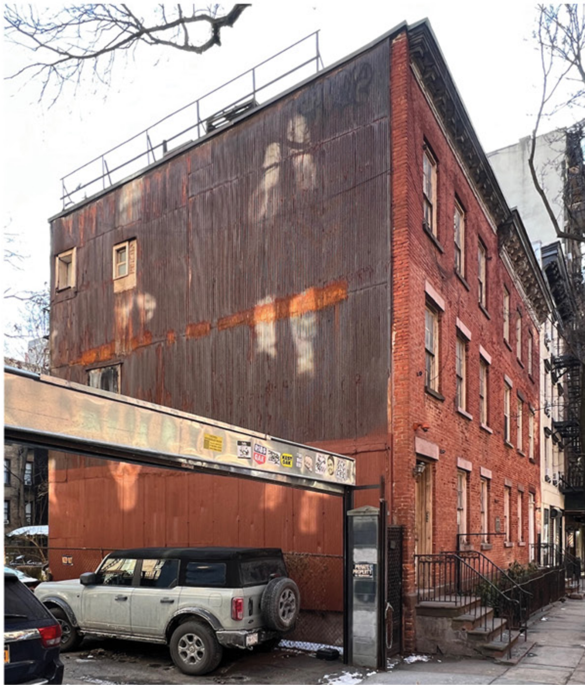
85 Sullivan Street North Facade Current photograph, deteriorated metal cladding, installed in 1930s
