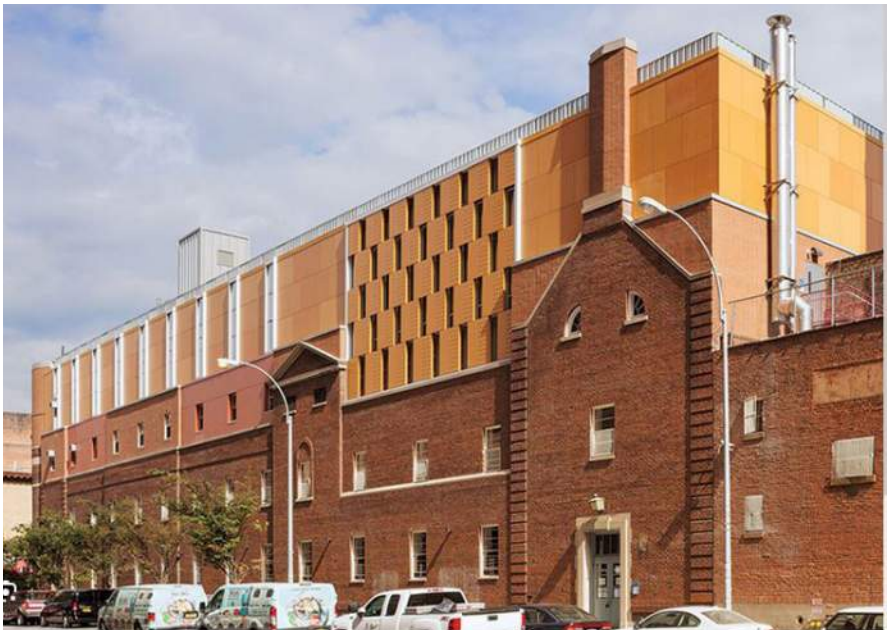
ST LUKE'S SCHOOL: CHANGE IN MATERIAL FROM BRICK OF EXISTING SCHOOL BUILDING IN 2017 VERTICAL EXPANSION
