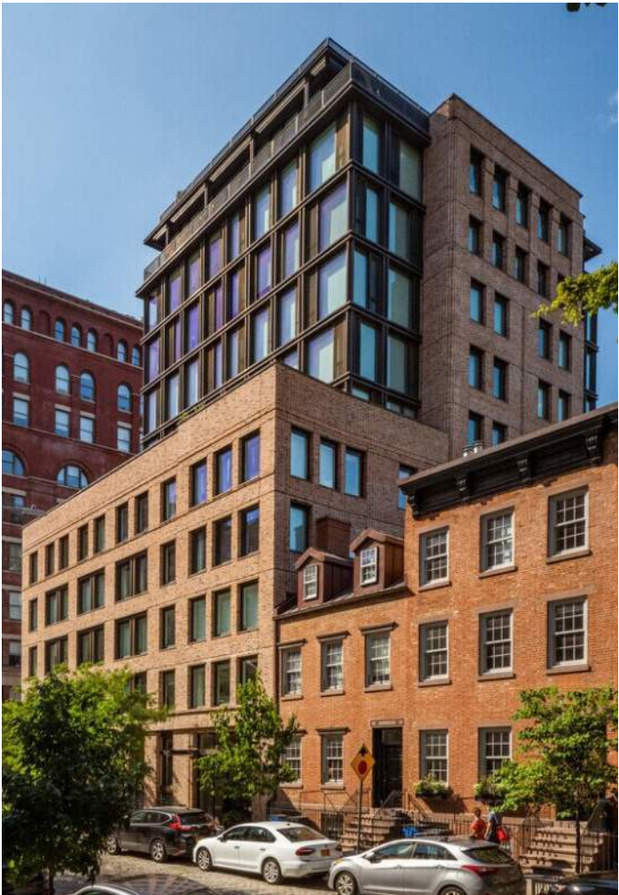
100 BARROW STREET: MATERIAL DISTINCTION BETWEEN BRICK BASE AND METAL PANEL ABOVE CONTEXTUAL DATUM, GRANITE WATER TABLE BASE
