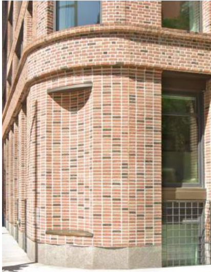
100 BARROW STREET: MATERIAL DISTINCTION BETWEEN BRICK BASE AND METAL PANEL ABOVE CONTEXTUAL DATUM, GRANITE WATER TABLE BASE
