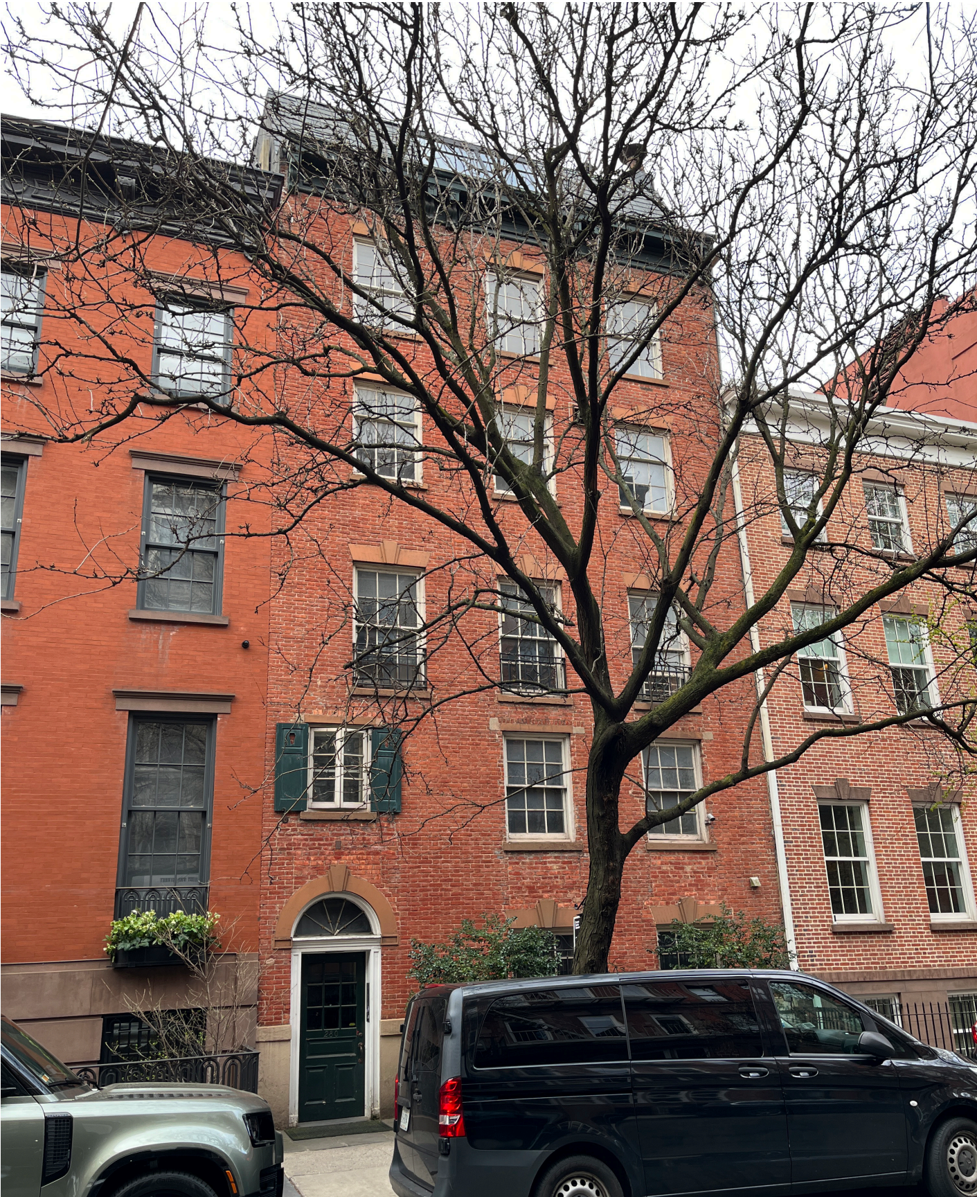
1. EXISTING FACADE OF 280 WEST 11TH STREET
