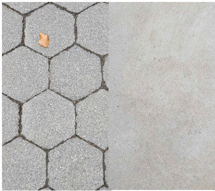
Asphalt Hex Tiles on Poured in Place Concrete Base
