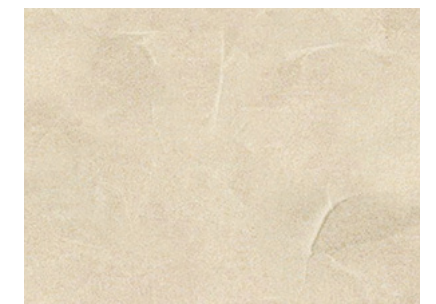
Plaster @ Interior Vault Ceiling
