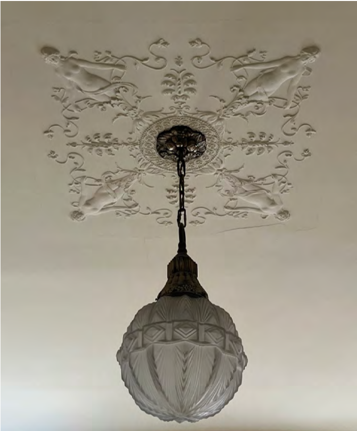
KITCHEN DECORATIVE PLASTER CEILING MEDALLION & LIGHT FIXTURE
