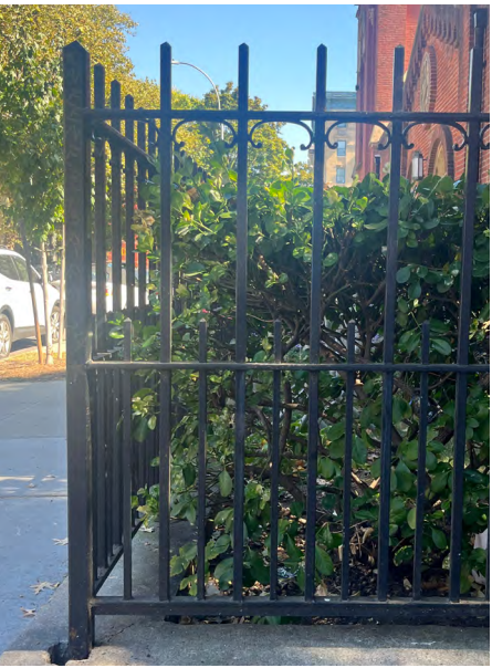
BROWN MEMORIAL BAPTIST CHURCH (484 WASHINGTON AVE) PROPERTY FENCE
