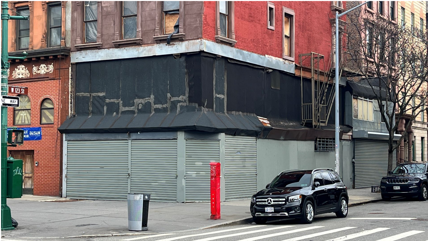
CORNER OF LENOX AVENUE AND WEST 123 RD STREET EXISTING STOREFRONT (LOOKING NORTHEAST)
