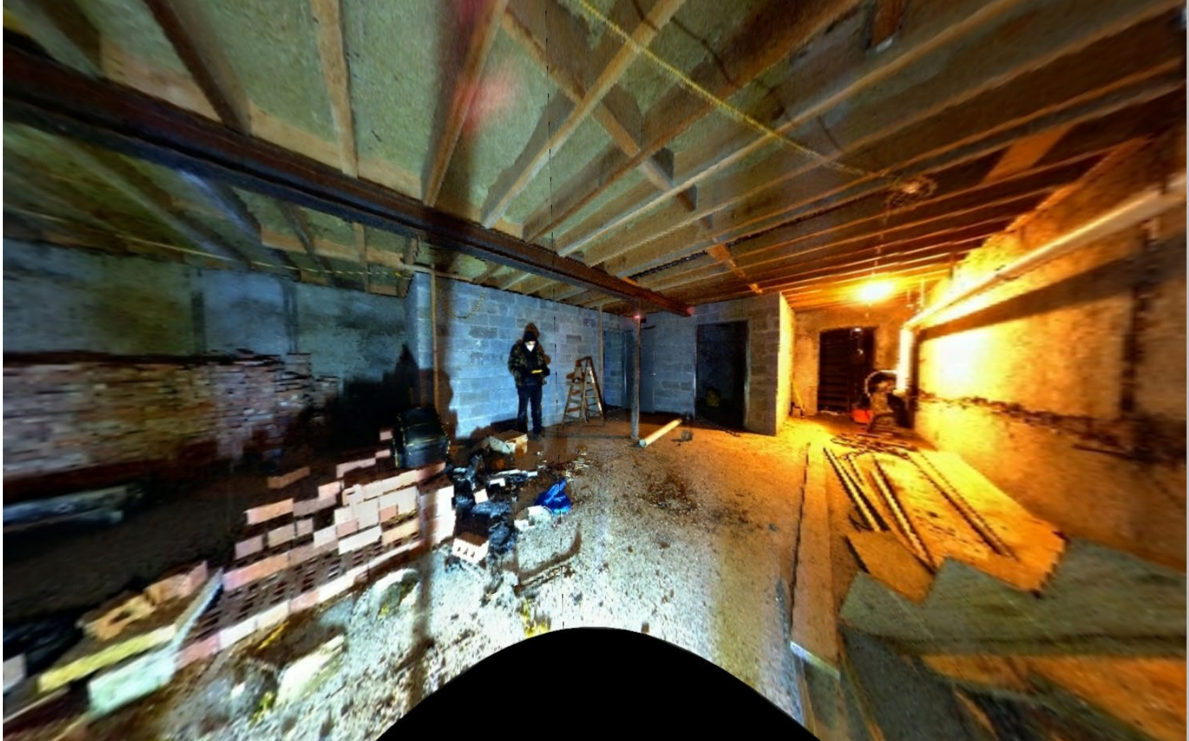
EXISTING CELLAR (LOOKING WEST)
