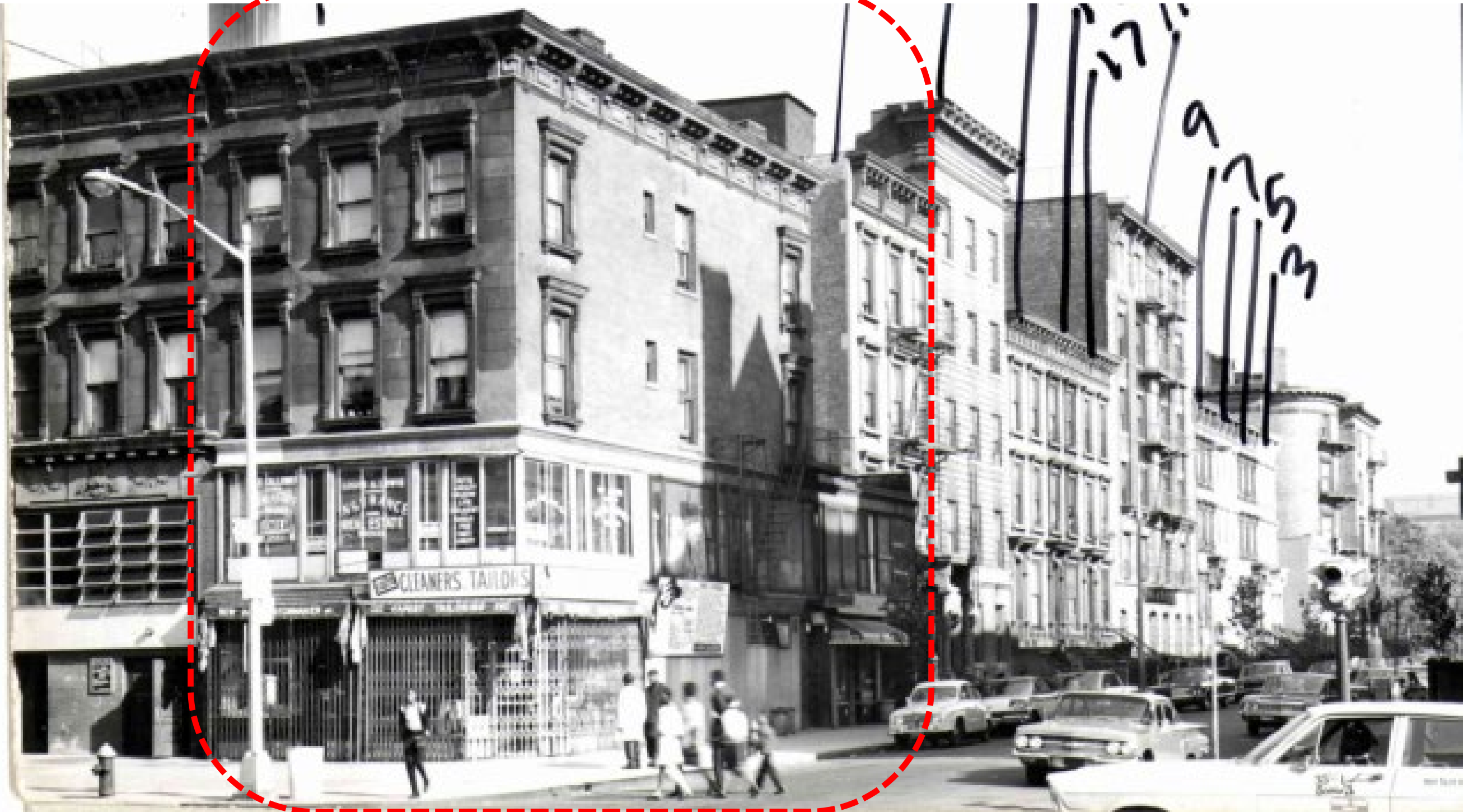
LPC DESIGNATION PHOTO, ca. 1971 (COURTESY OF NYC LANDMARKS PRESERVATION COMMISSION)
