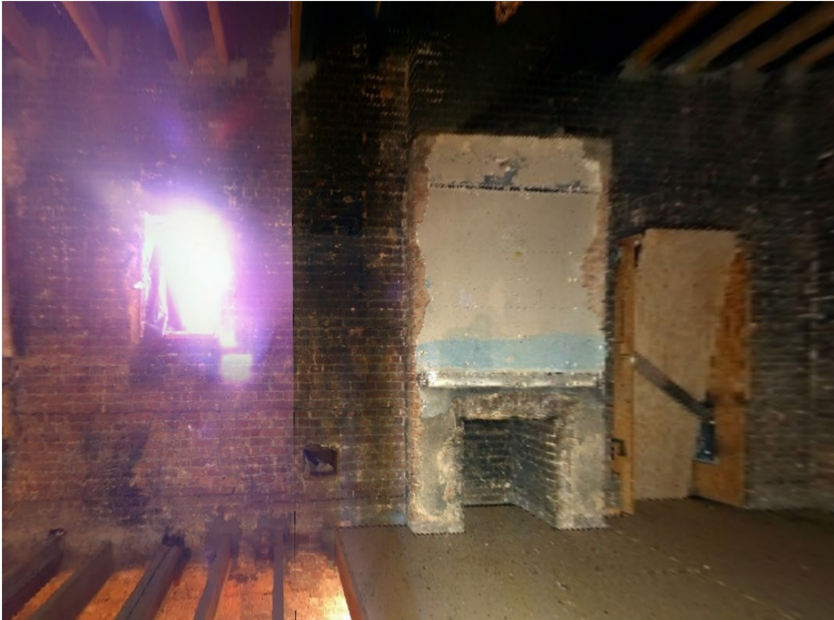
EXISTING FOURTH FLOOR (LOOKING SOUTH)
