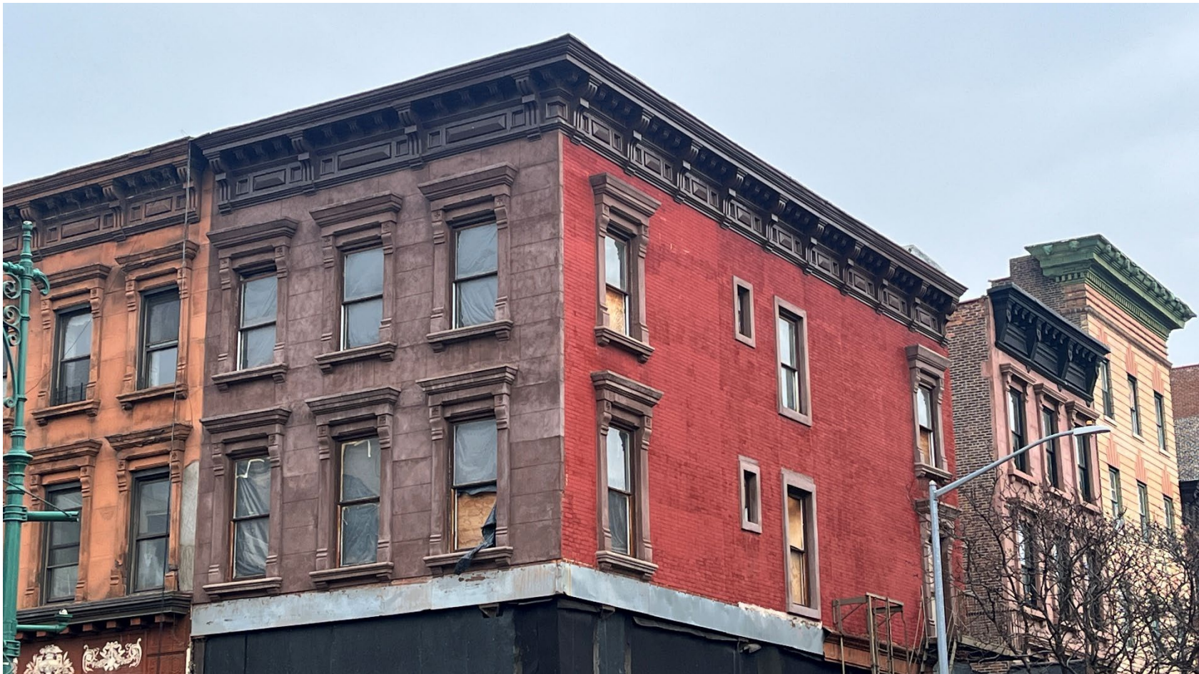
CORNER OF LENOX AVENUE AND WEST 123 RD STREET EXISTING MASONRY FACADES (LOOKING NORTHEAST)
