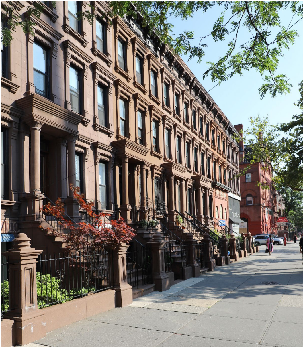
EXISTING VIEW ALONG LENOX AVENUE SIDEWALK
