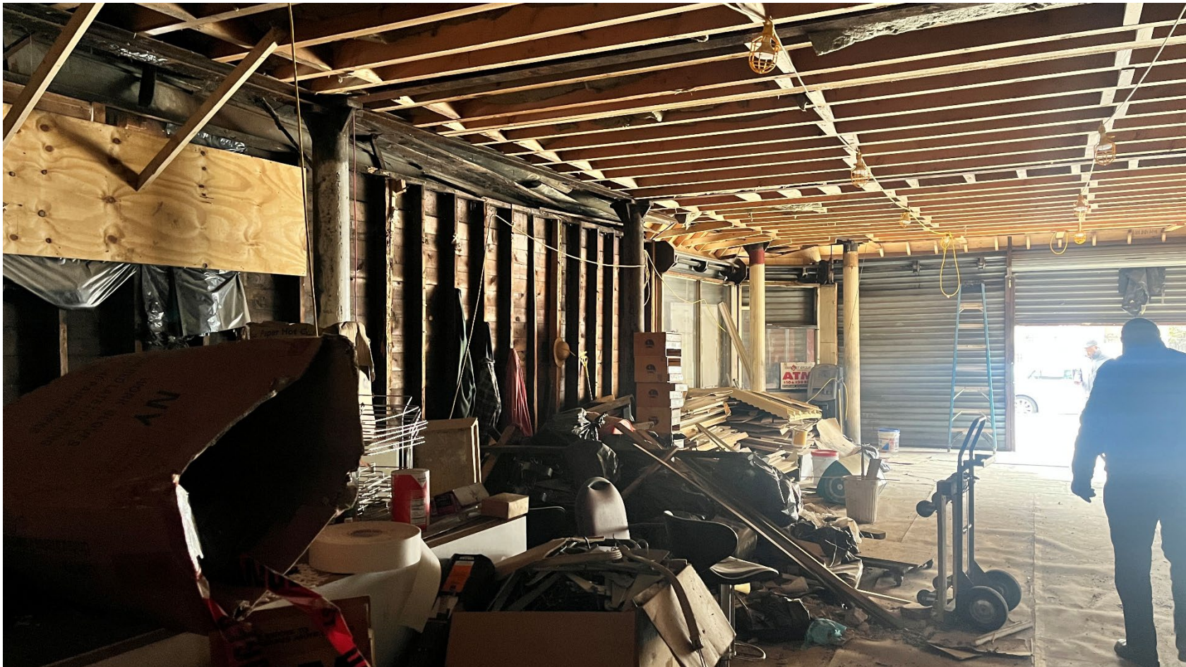
EXISTING FIRST FLOOR (LOOKING WEST)
