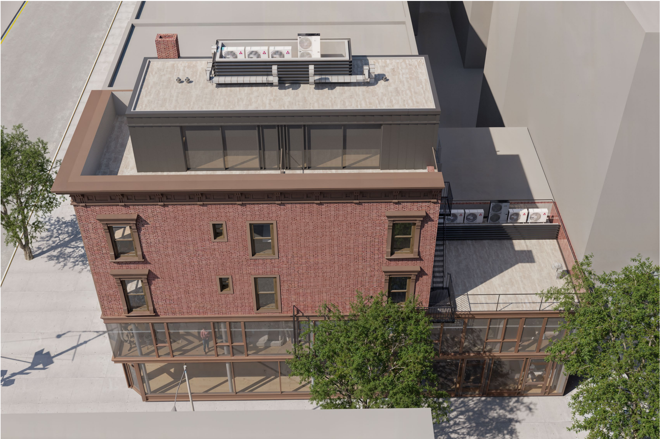
AERIAL VIEW ALONG WEST 123 RD STREET
