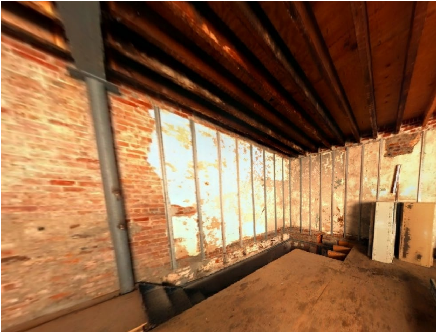
EXISTING SECOND FLOOR (LOOKING SOUTH)
