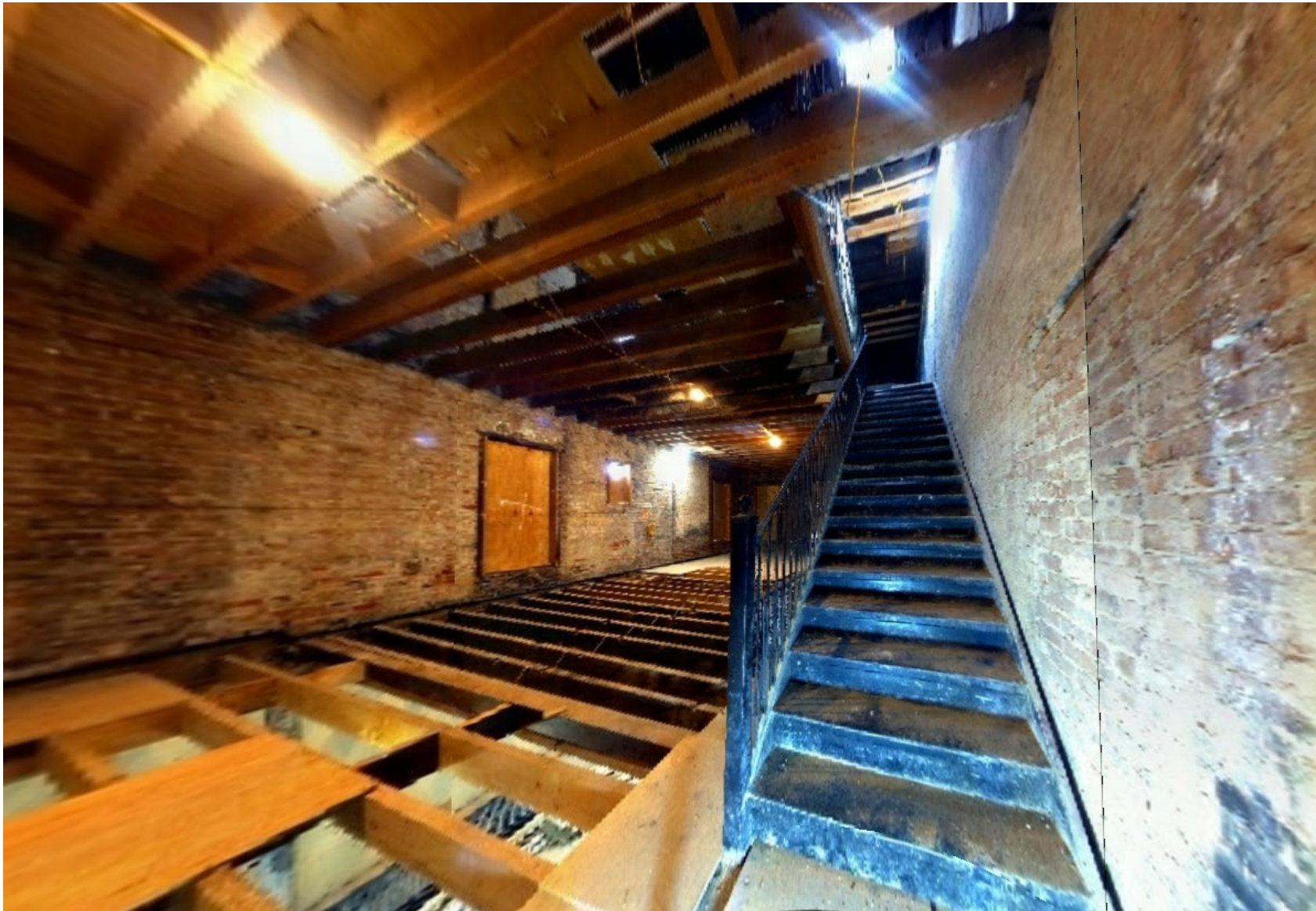
EXISTING THIRD FLOOR (LOOKING SOUTHWEST)
