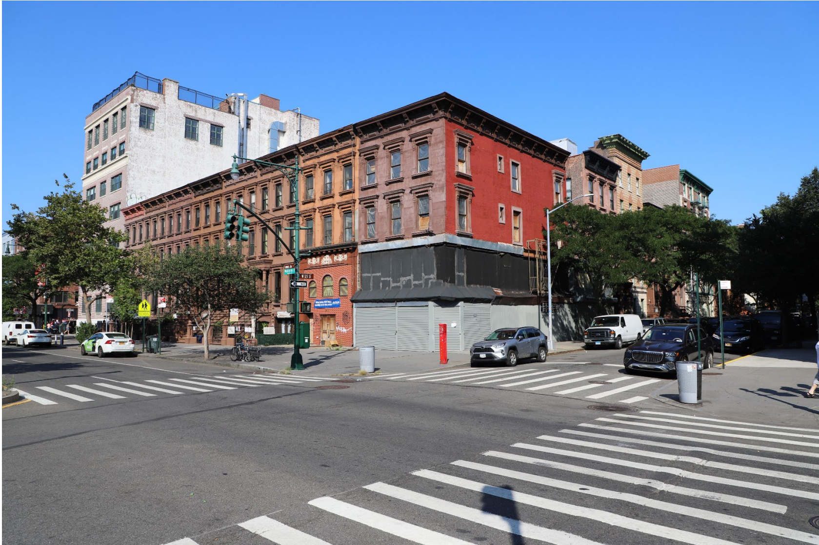
EXISTING CORNER VIEW AT LENOX AVENUE AND WEST 123RD STREET
