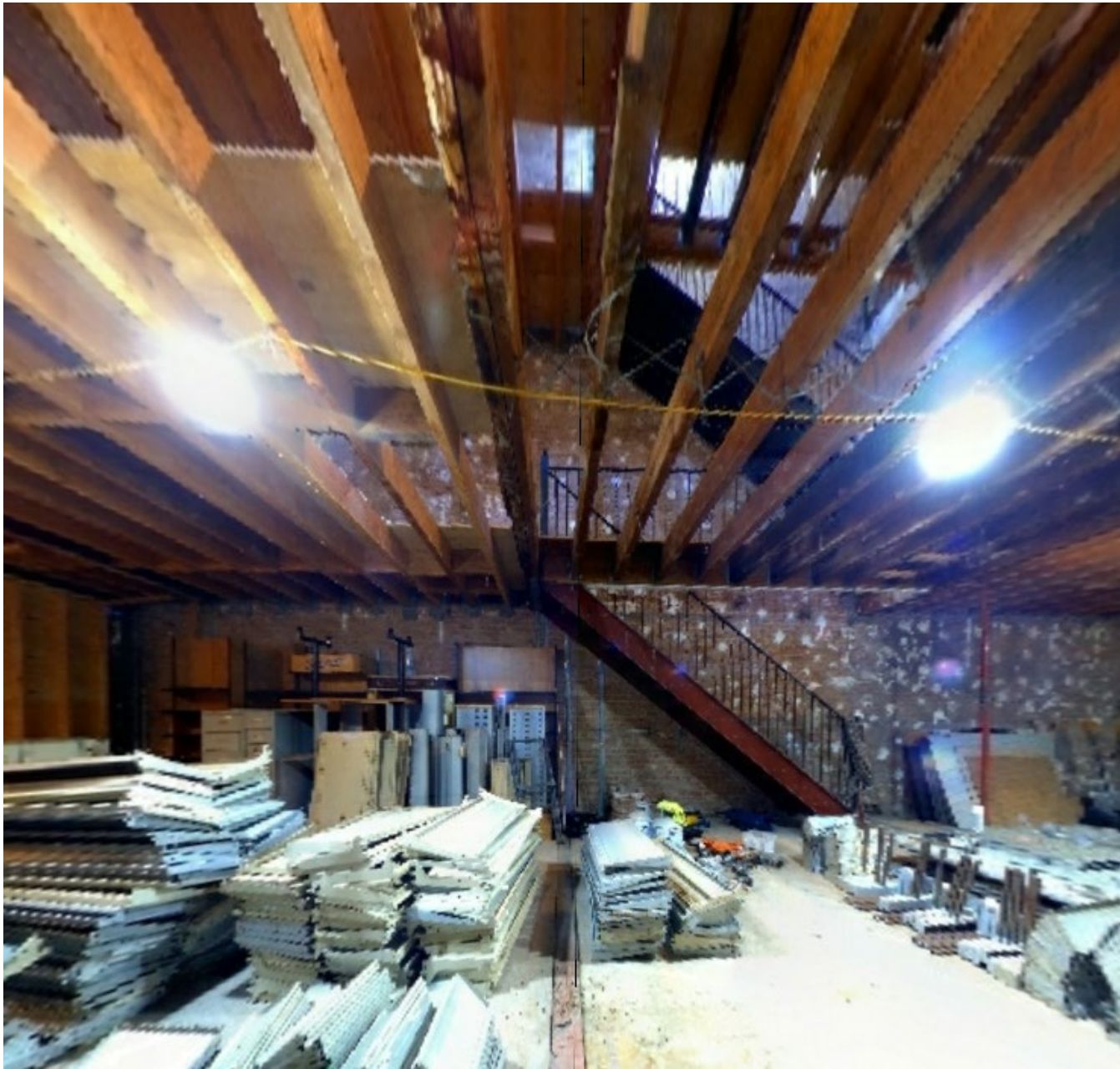
EXISTING SECOND FLOOR (LOOKING NORTH)
