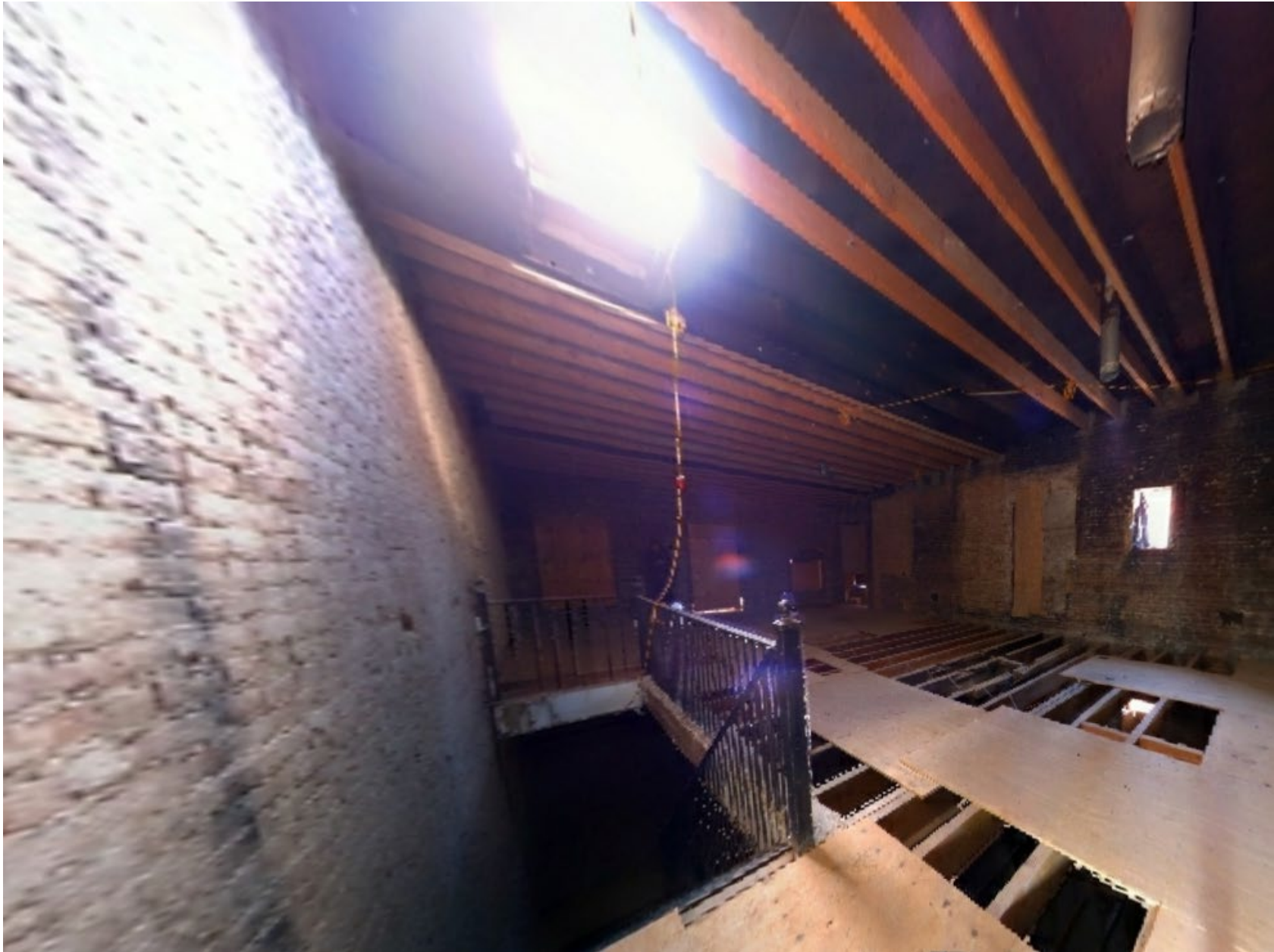
EXISTING FOURTH FLOOR (LOOKING SOUTHEAST)
