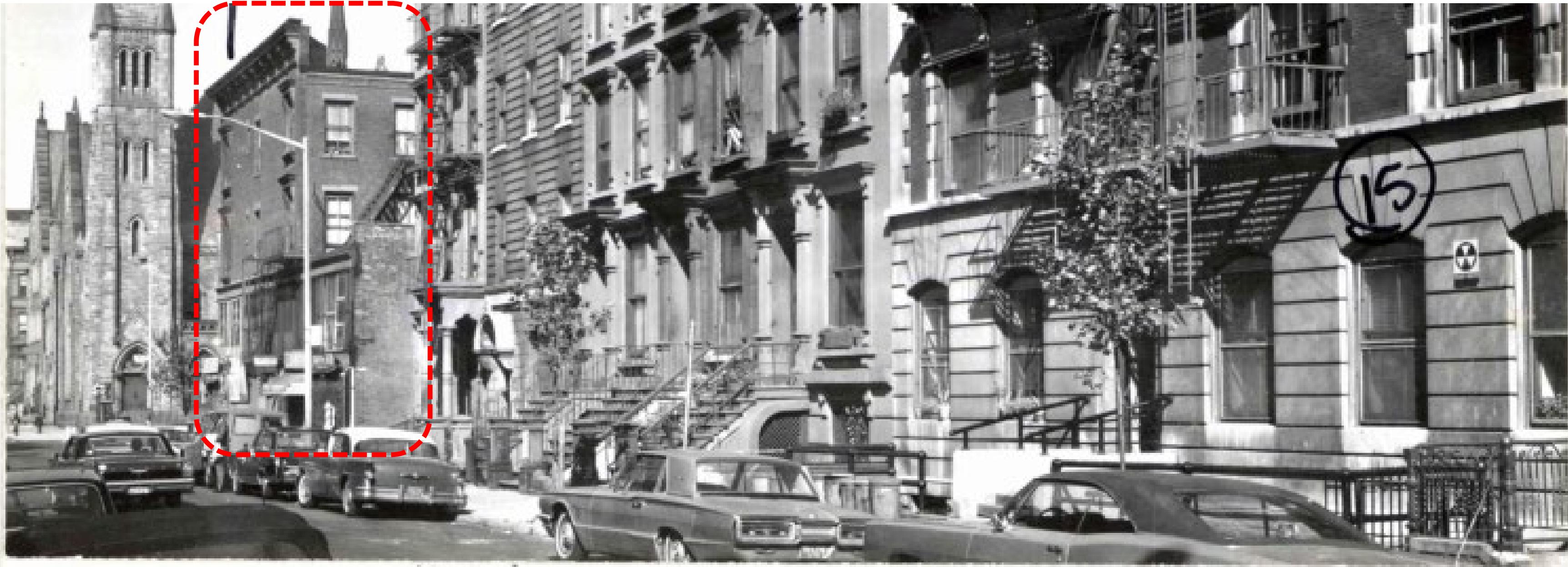
LPC DESIGNATION PHOTO, ca. 1971 (COURTESY OF NYC LANDMARKS PRESERVATION COMMISSION)
