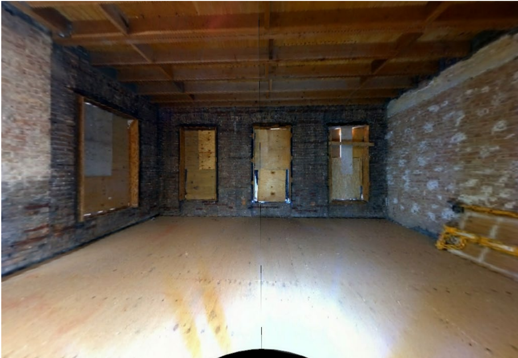
EXISTING THIRD FLOOR (LOOKING WEST)
