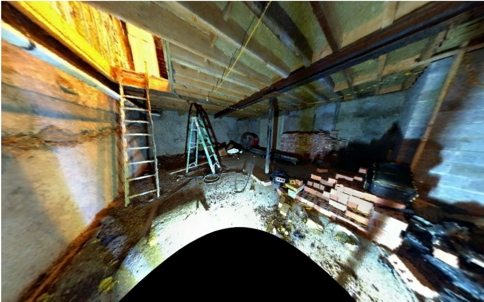
EXISTING CELLAR (LOOKING EAST)
