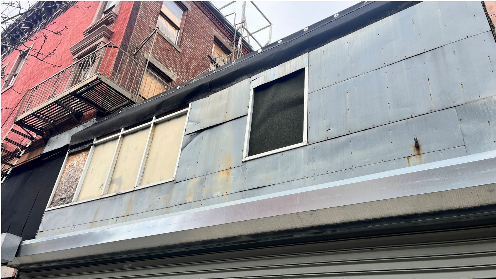
EXISTING WEST 123 RD STREET SECOND FLOOR STOREFRONTS AND MASONRY FACADE
