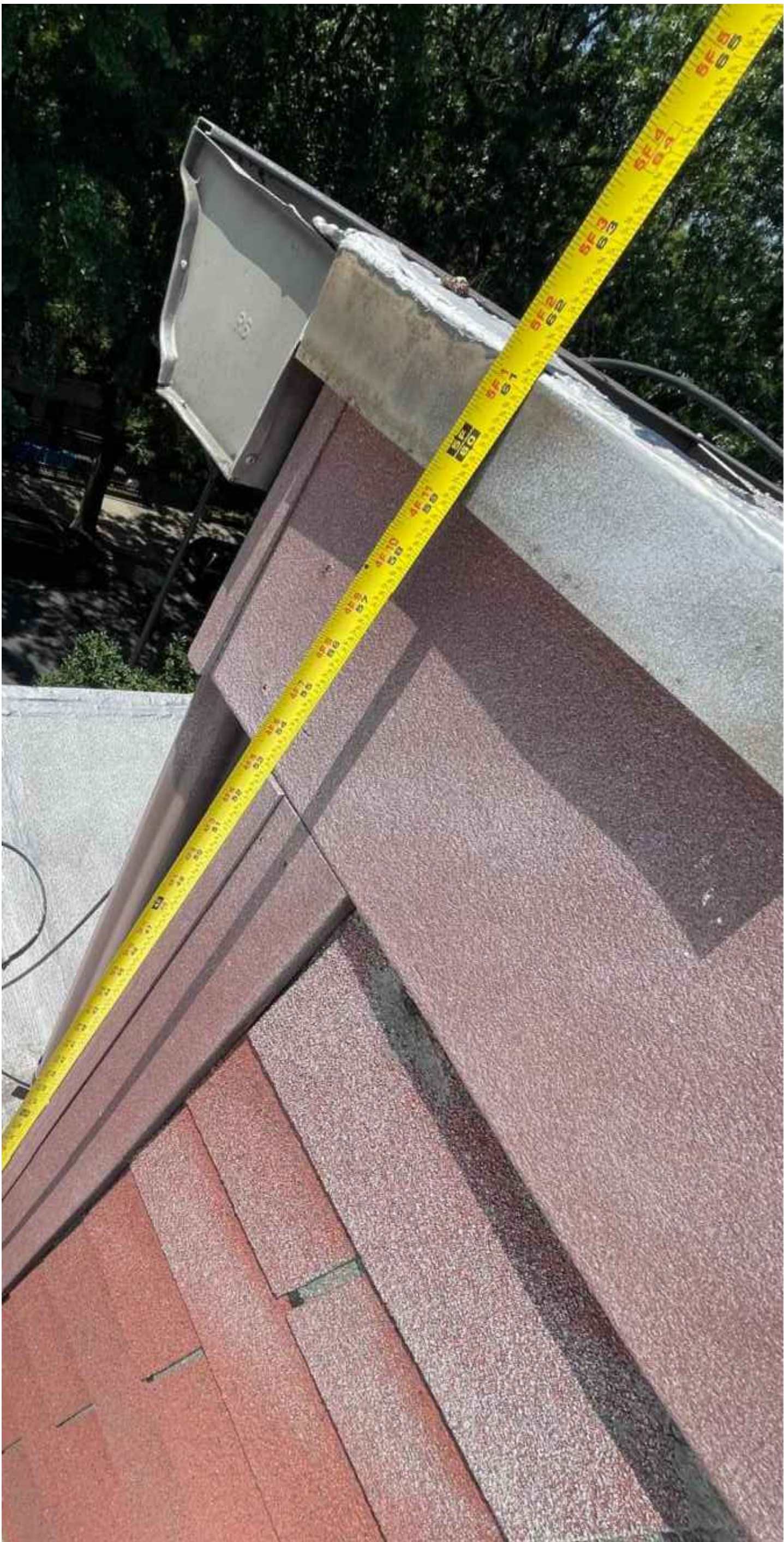
ROOF VIEW TOWARDS 181 PROSPECT PLACE
