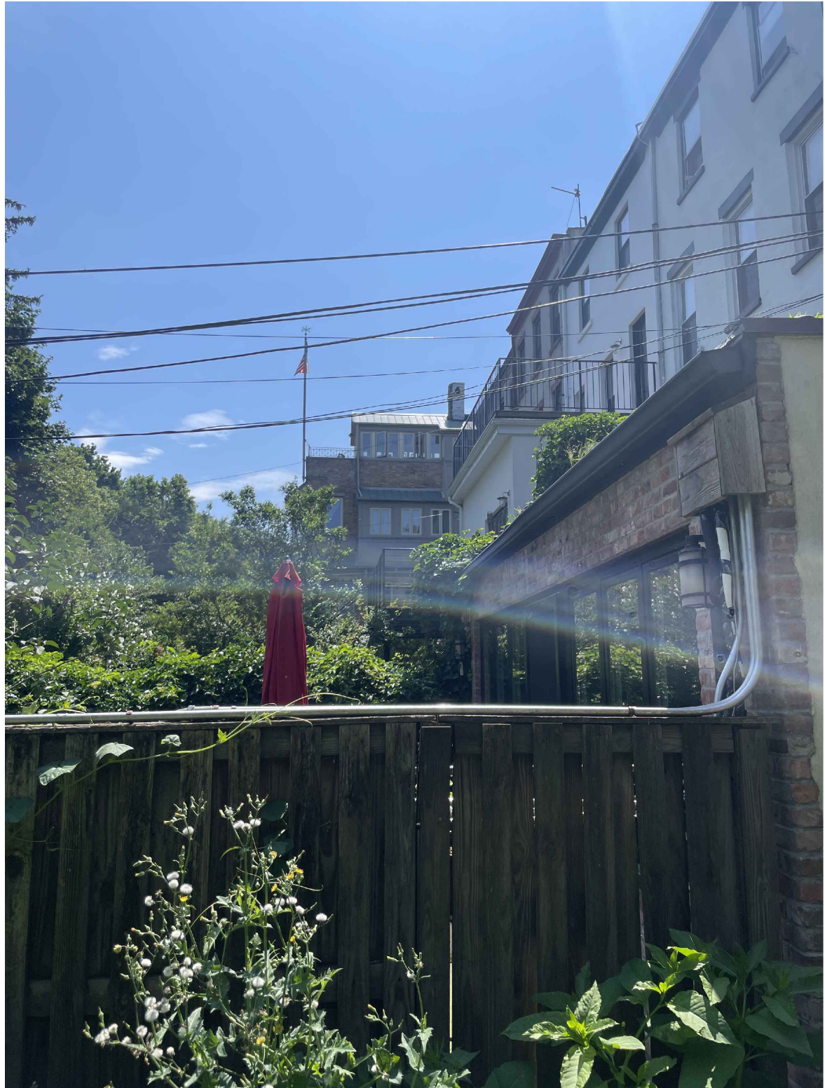
REAR FACADE FACING PAST 185 PROSPECT PLACE
