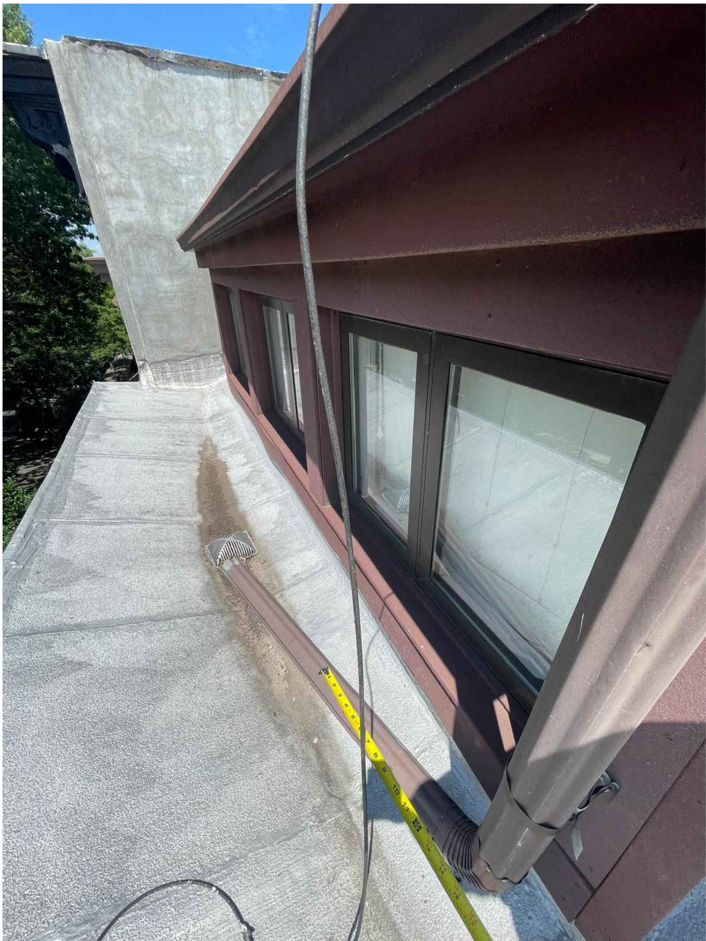
ROOF VIEW TOWARDS 181 PROSPECT PLACE
