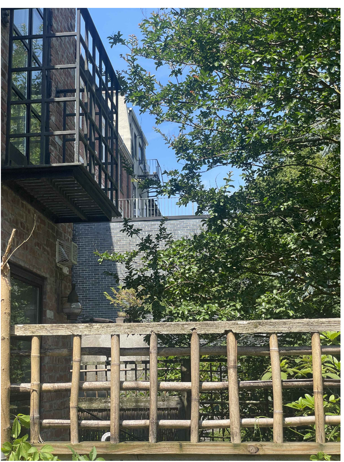
REAR FACADE FACING PAST 181 PROSPECT PLACE
