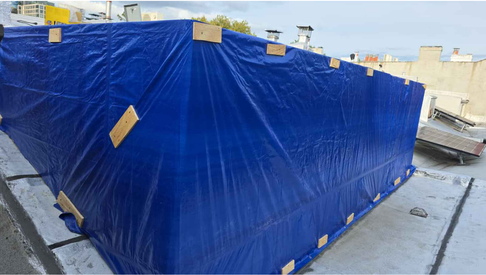
ROOF VIEW AT 183 PROSPECT PLACE FACING NORTHEAST
