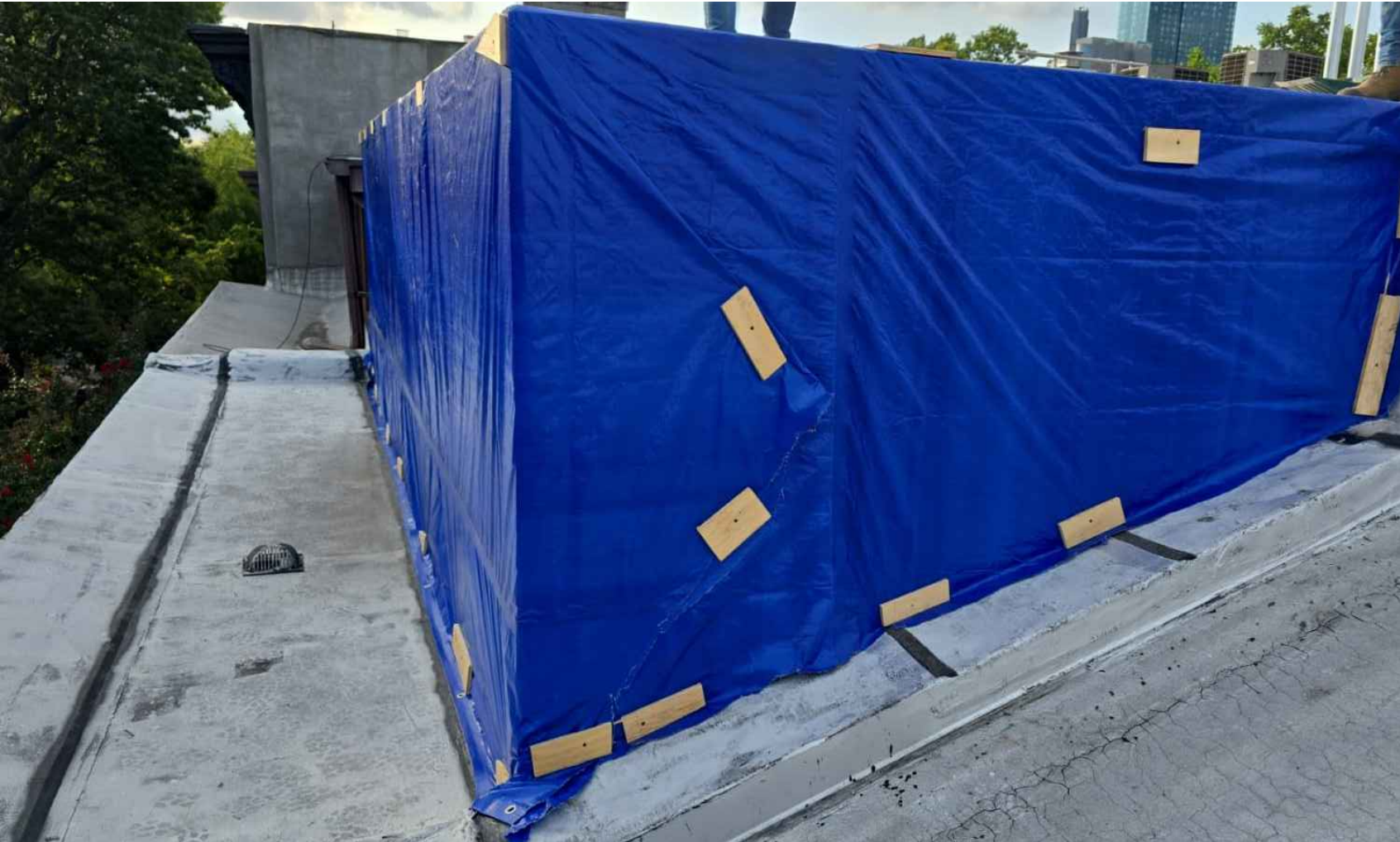
ROOF VIEW AT 183 PROSPECT PLACE FACING SOUTHWEST
