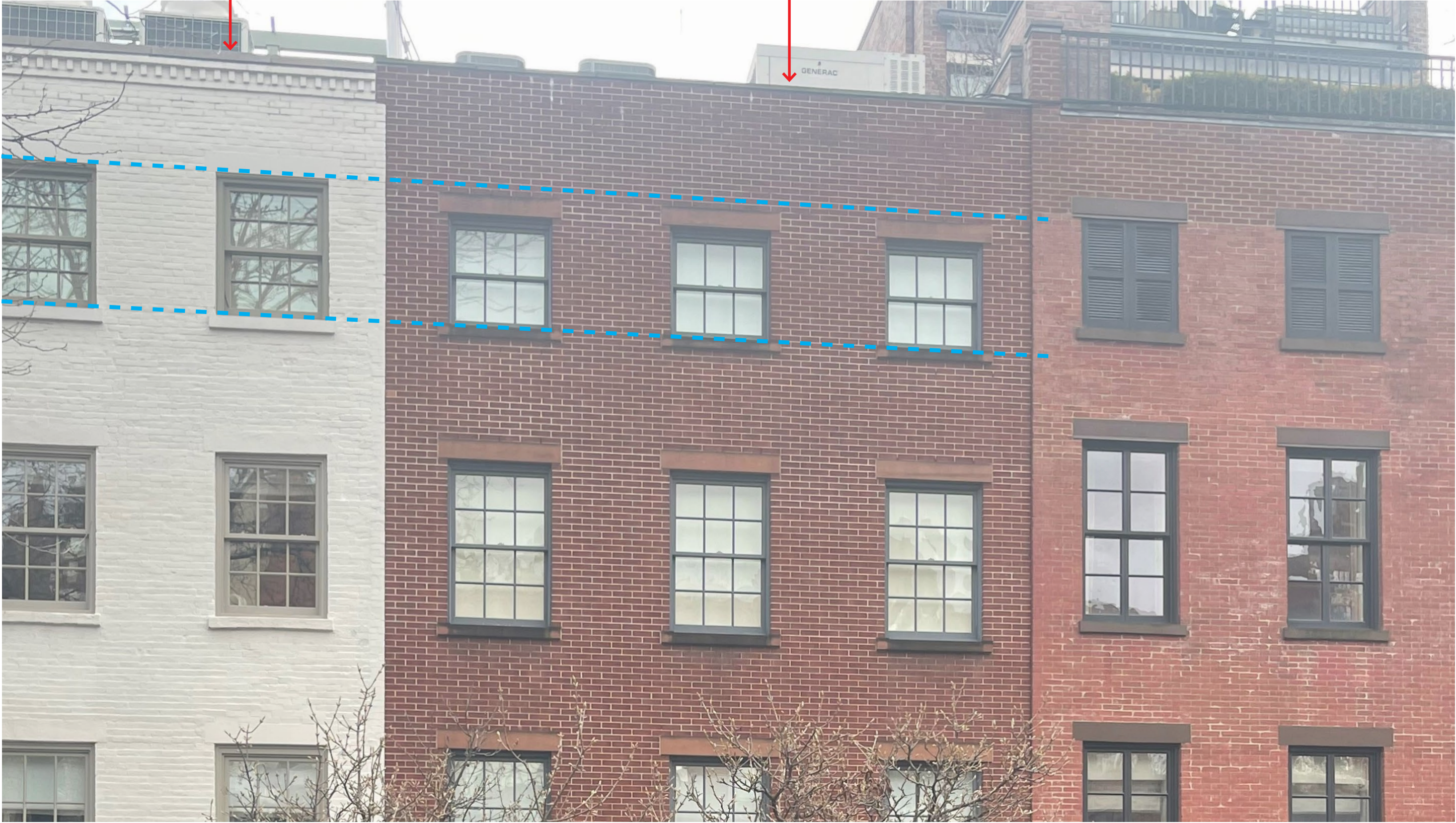
Existing window conditions at the fourth floor, rear facade
