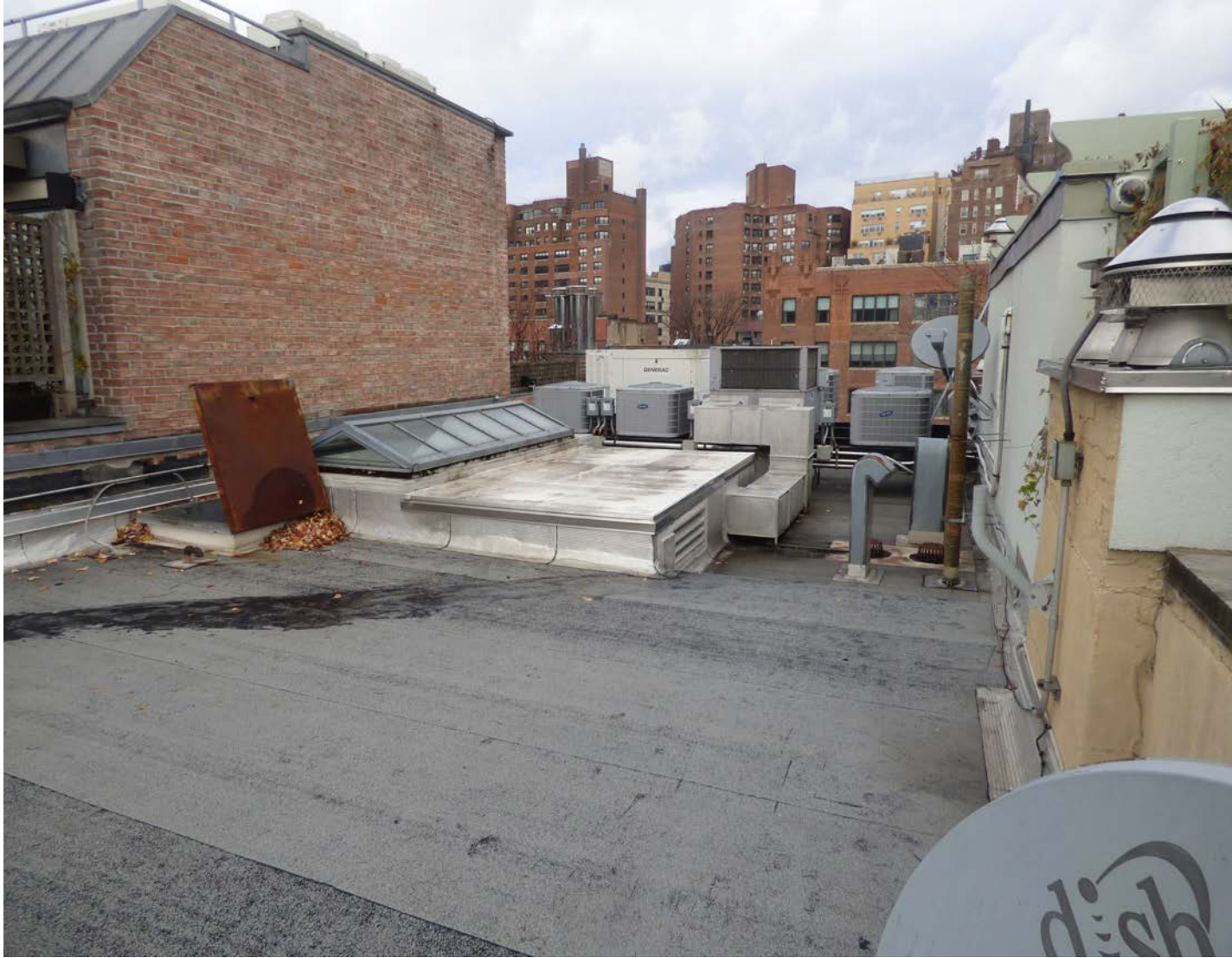
Existing roof conditions, looking north from Bank Street parapet
