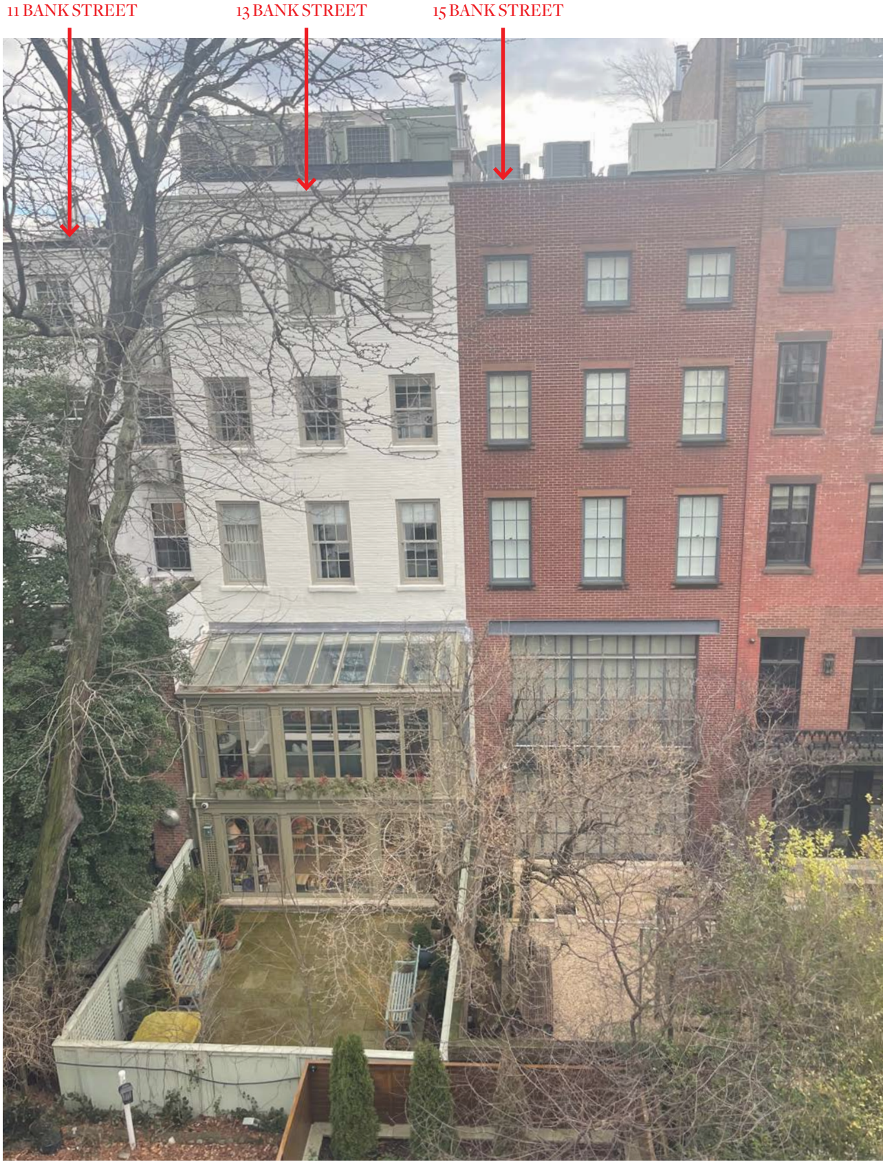
Existing conditions at 13 and 15 Bank Street
