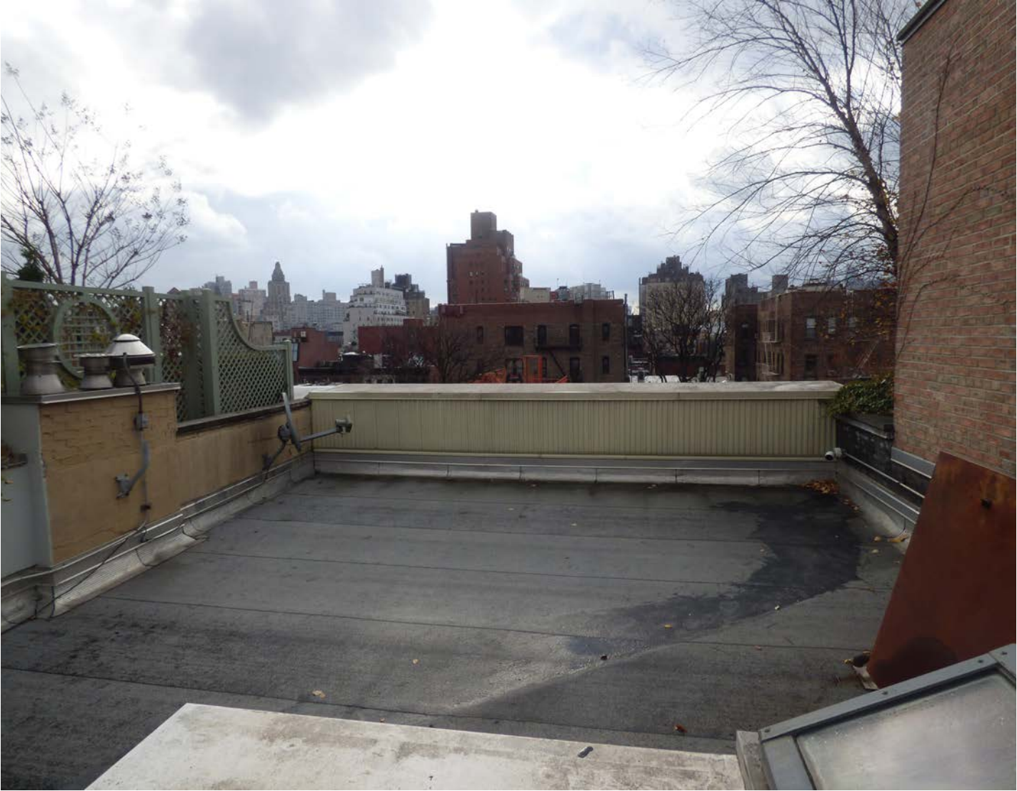
Existing roof conditions, looking south from Bank Street parapet
