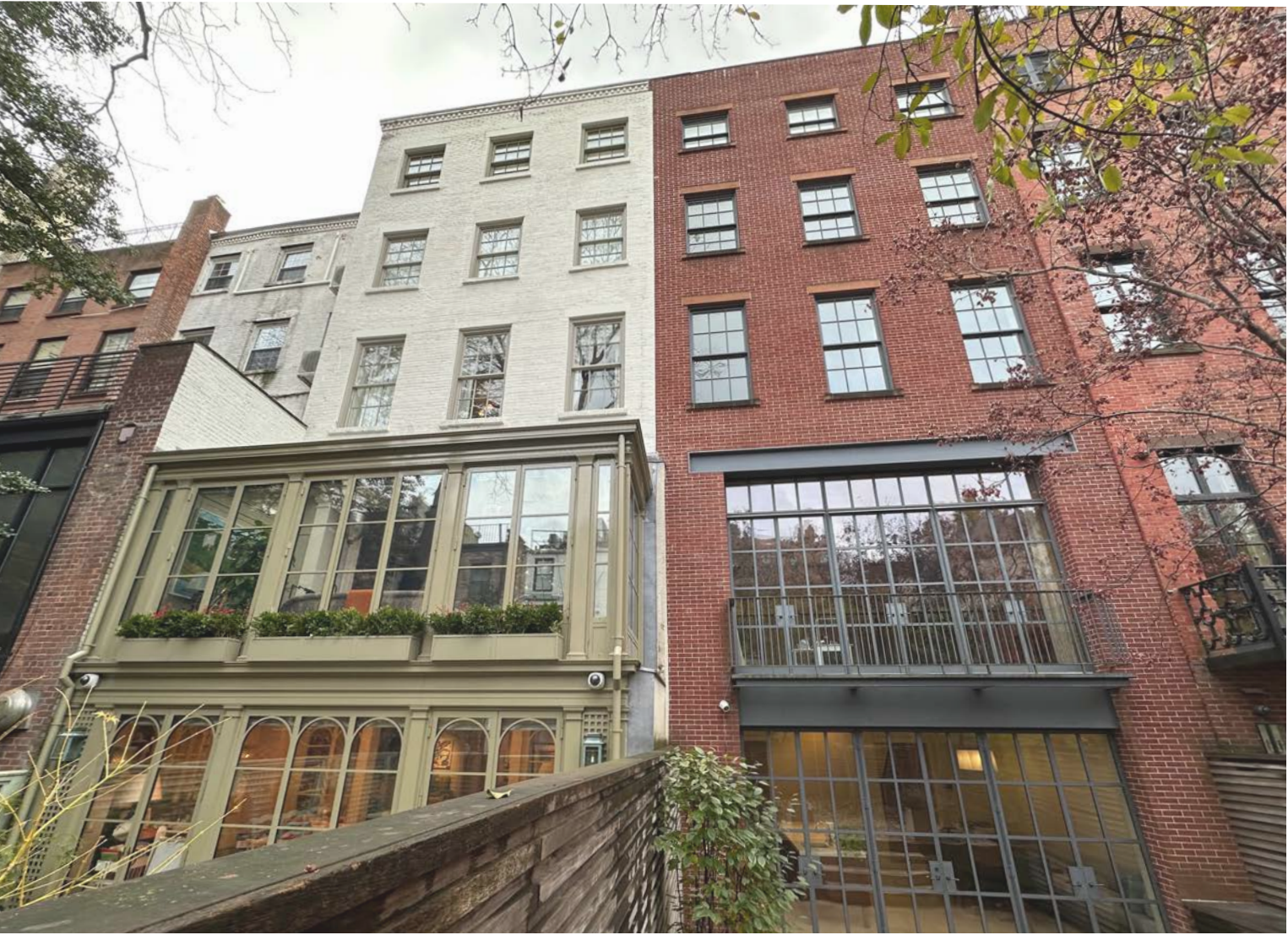
View from 15 Bank rear yard
