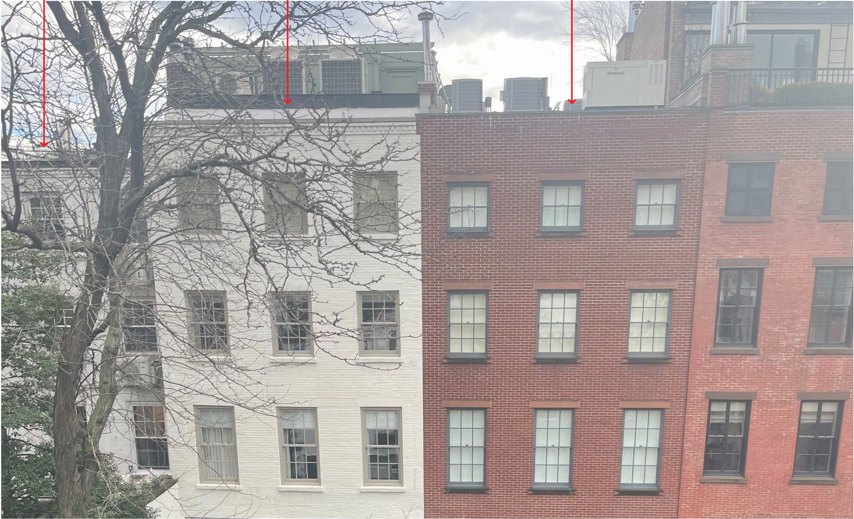
Rear Facade Windows
