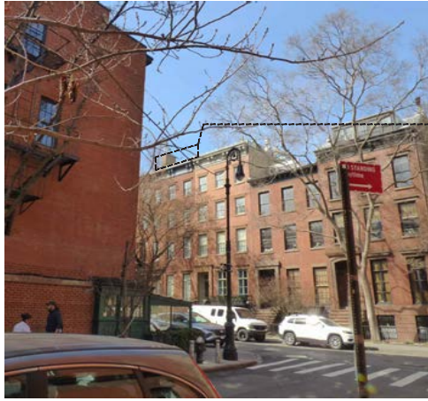
6 A306.01 13 BANK ST - VIEW FROM WAVERLY PLACE
