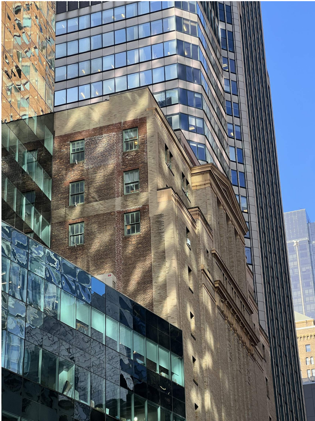
1. 56TH STREET - VIEW FROM NORTH EAST CORNER
