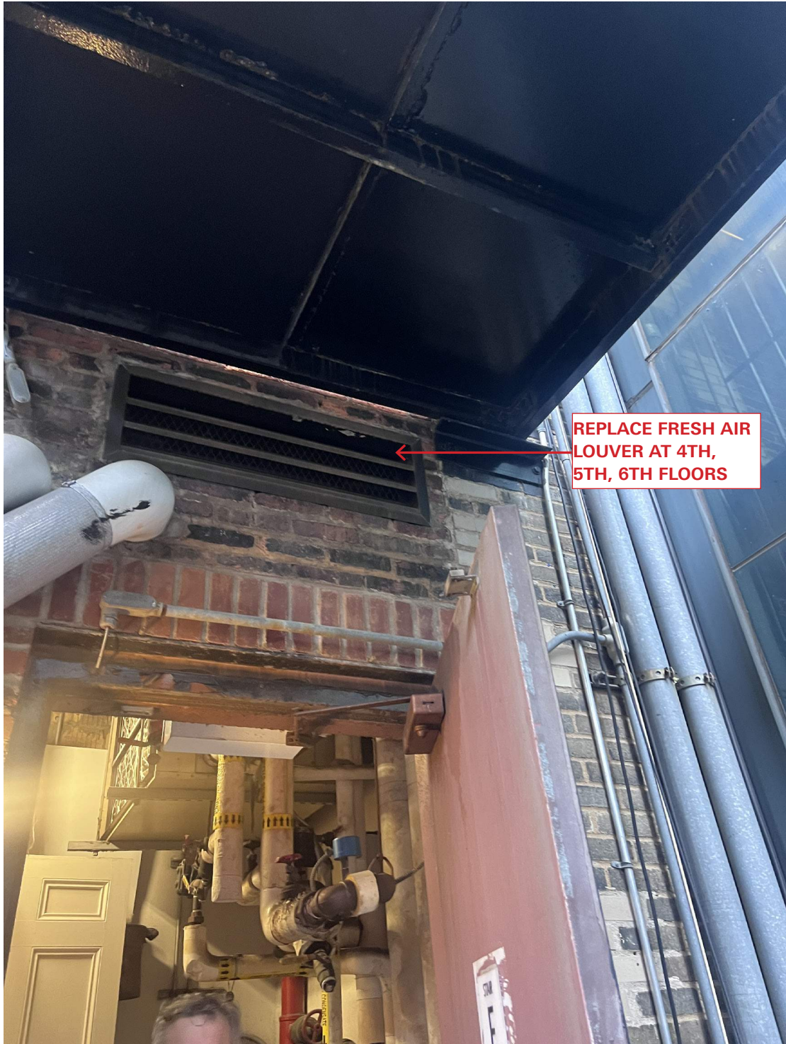
3. SOUTH FACADE - EXISTING LOUVER
