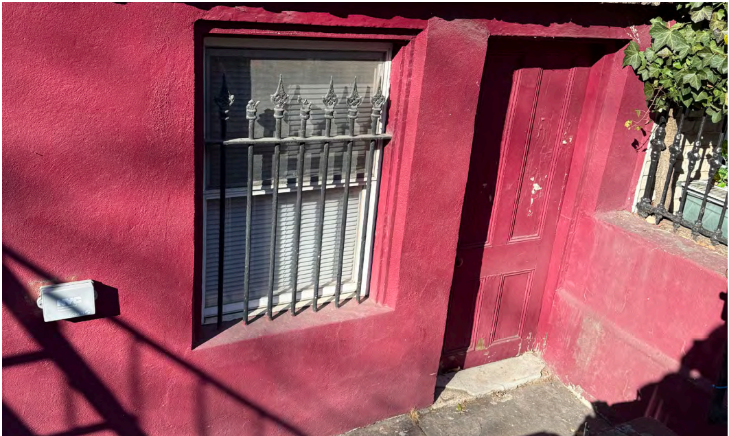
113 NOBLE STREET, EXISTING FRONT AREAWAY
