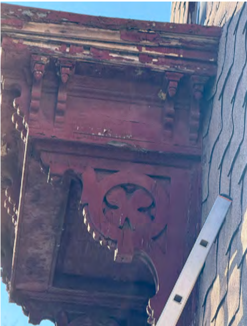
113 NOBLE STREET, EXISTING FRONT DOOR SURROUND
