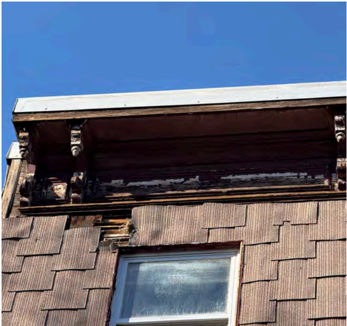
113 NOBLE STREET, EXISTING FRONT CORNICE
