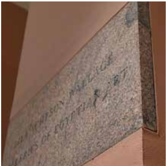
MARBLE INSET INTO CLAY PAINTED COLUMN
