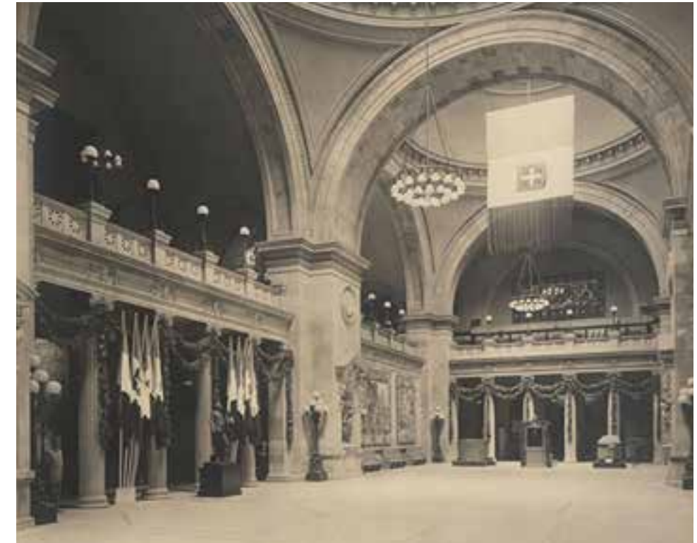
GREAT HALL, LOOKING NORTH, 1917 New light fixtures were added.
