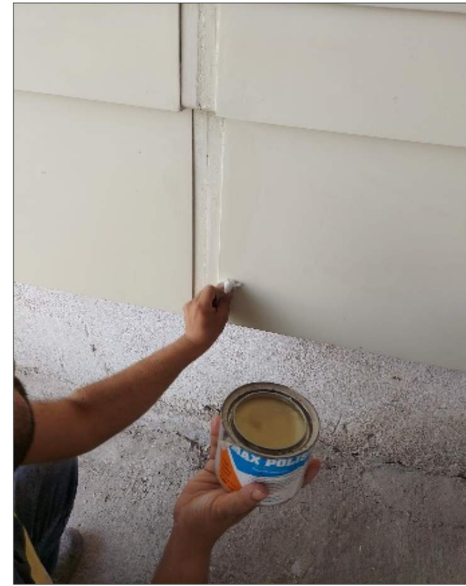
3. APPLY WAX ON FLAT EDGES ON PANEL
