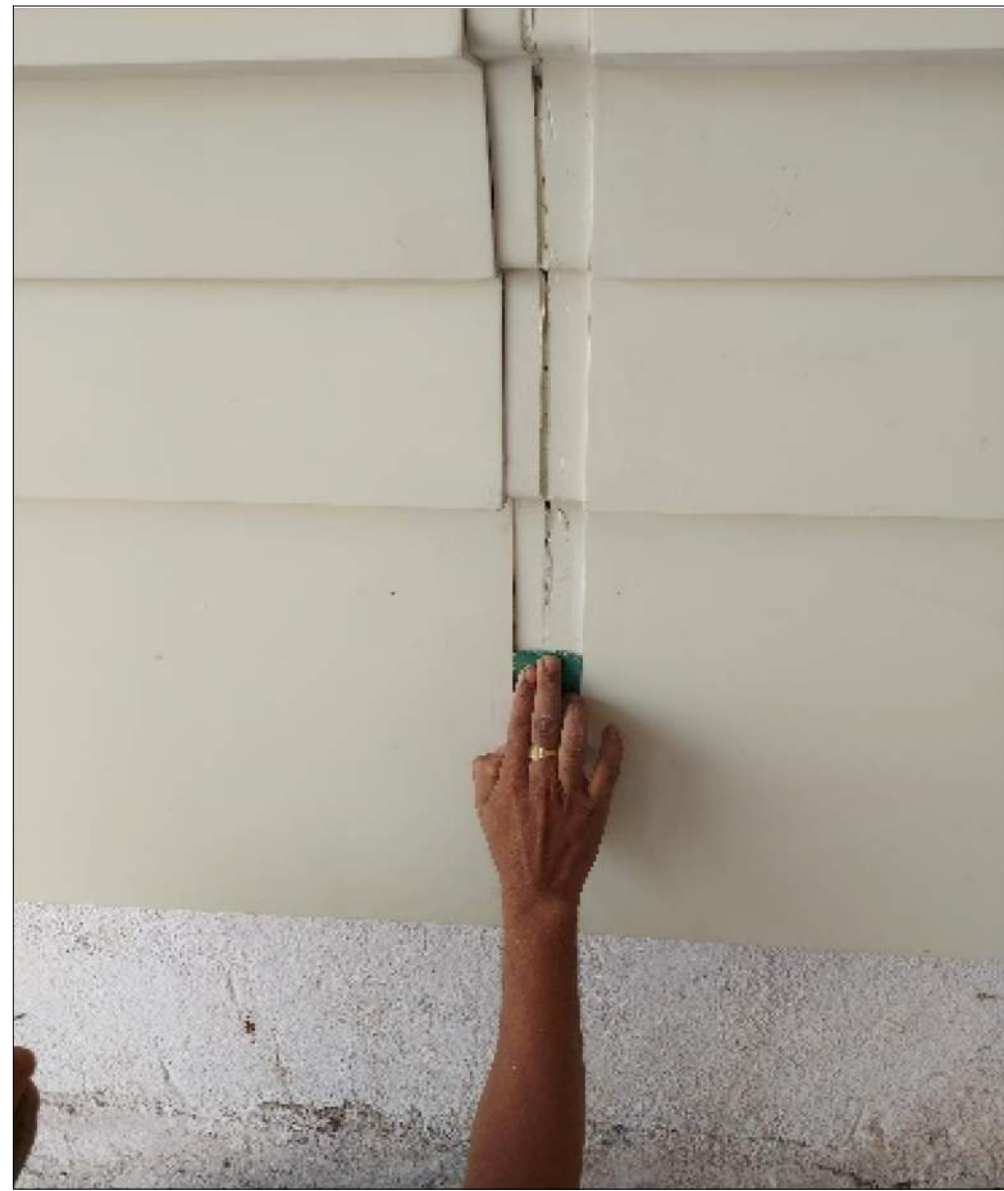
1. SAND AREA BETWEEN PANELS
