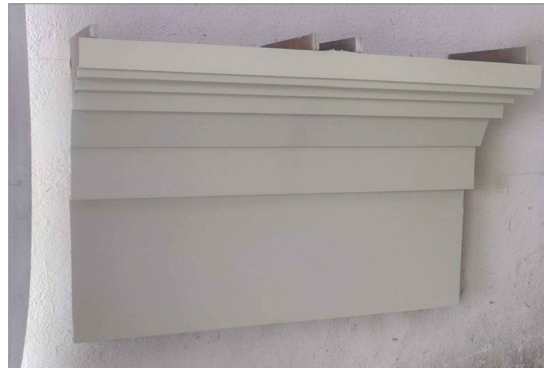
11. FIELD PAINT THE FINISHED CORNICE
