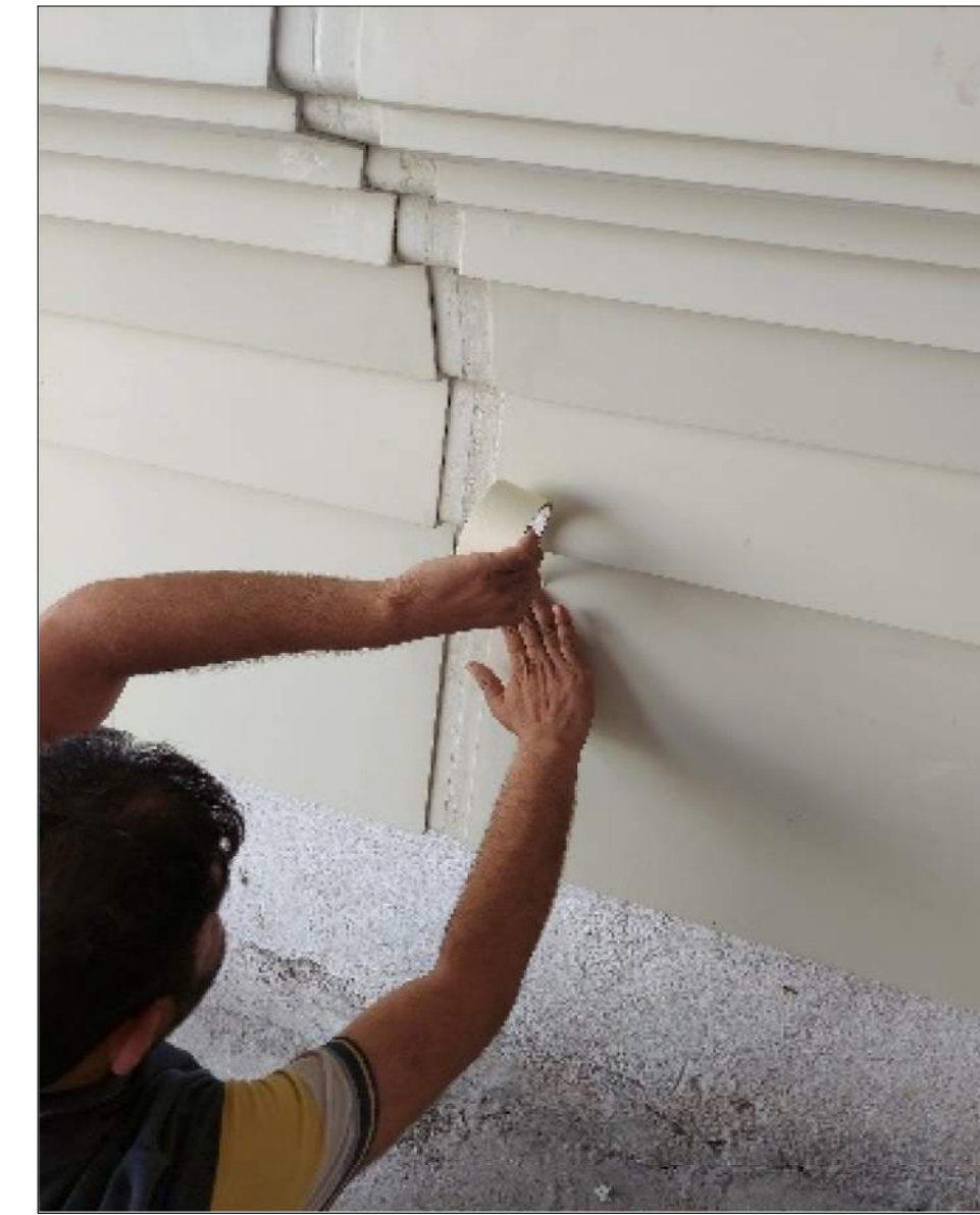
4. APPLY MASKING TAPE ON BOTH PANEL FLAT SURFACE EDGES
