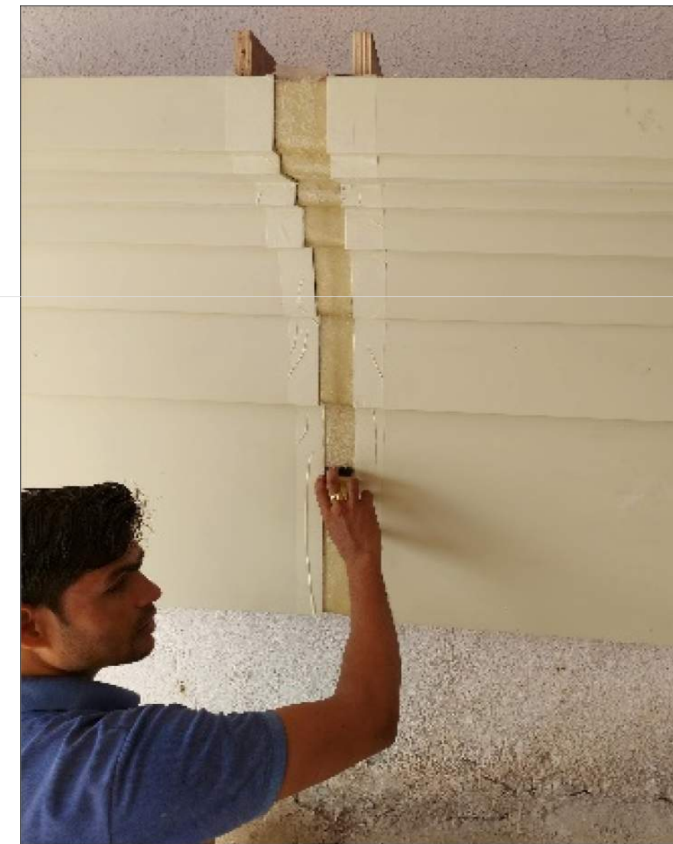
8. SAND TAPED JOINT
