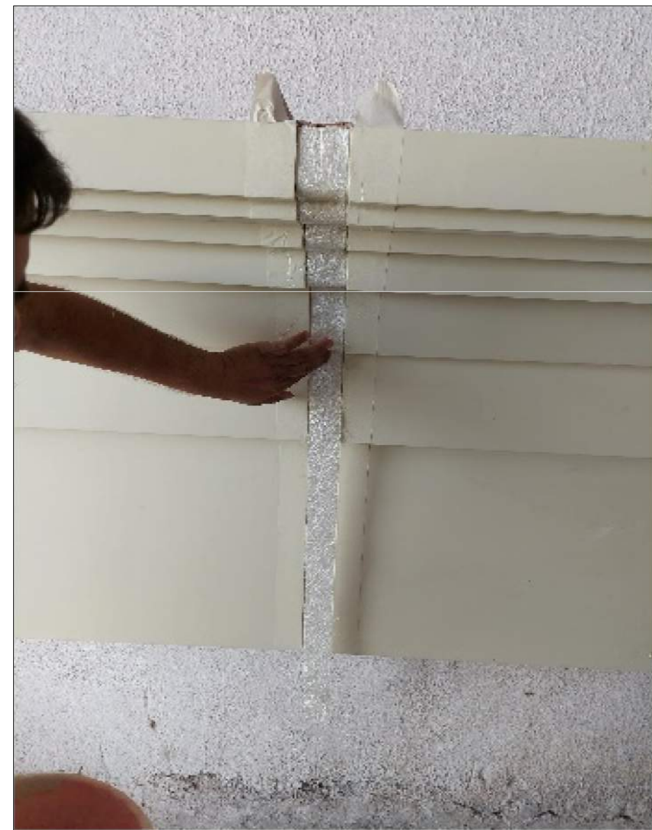
6. BOND 2 LAYERS OF 450 GSM MAT WITH RESIN AT RECESS JOINT
