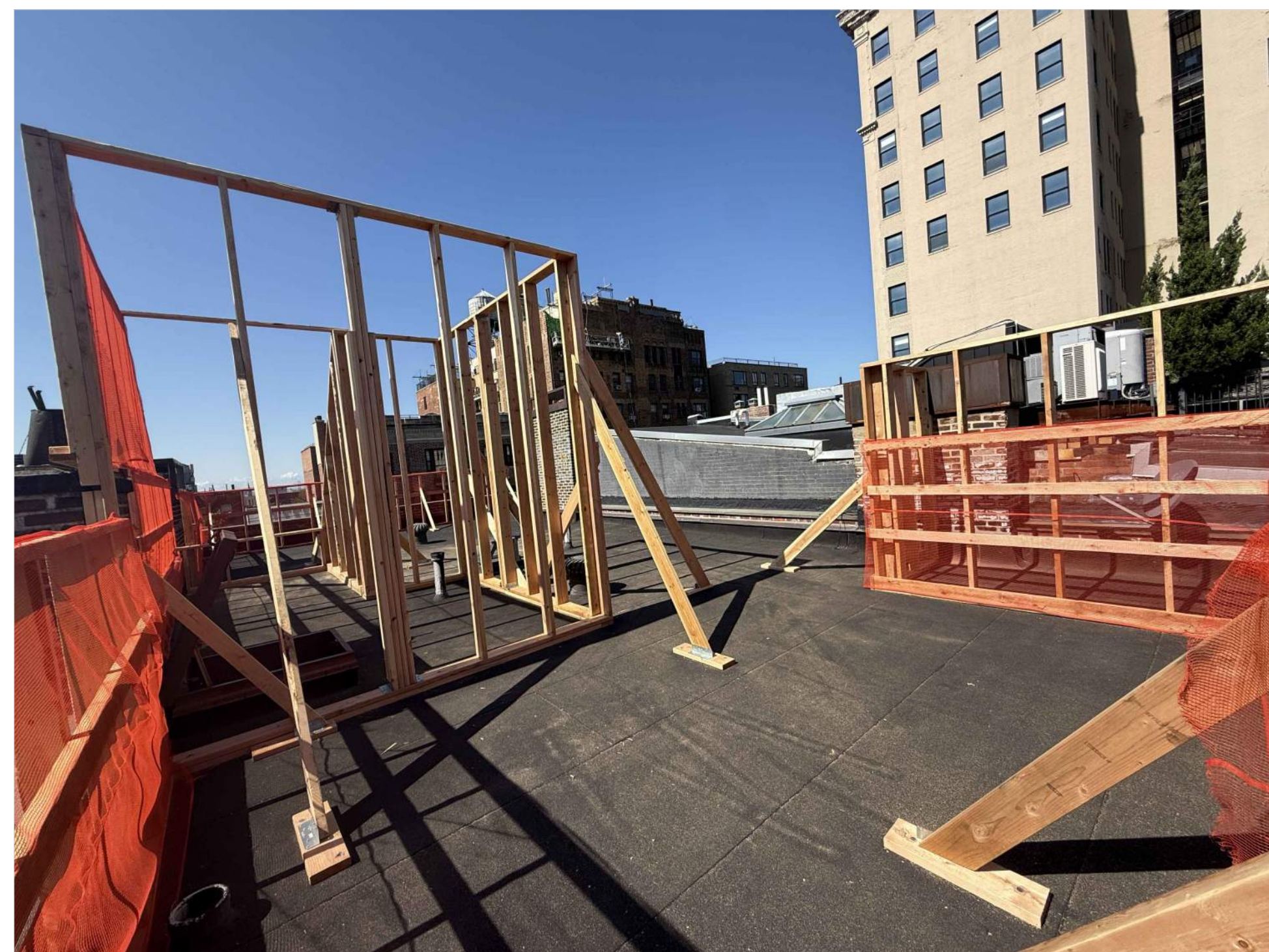
3. VIEW LOOKING SOUTH
