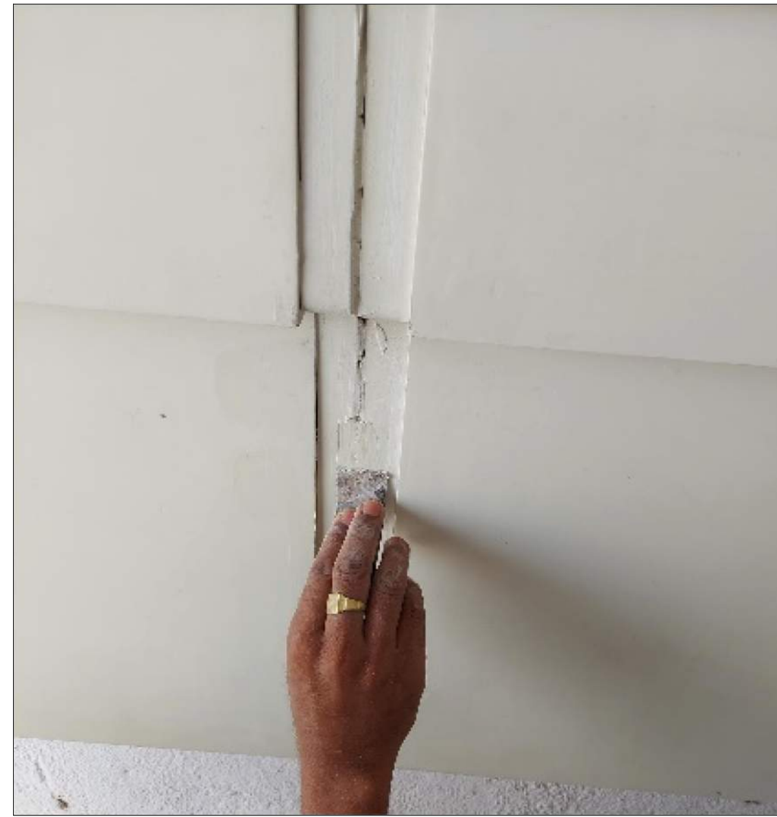
2. INFILL JOINT WITH PUTTY
