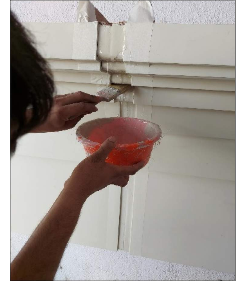
5. APPLY RESIN ON RECESS JOINT AREA
