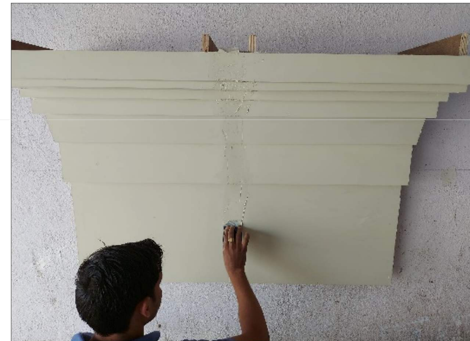
9. APPLY PUTTY TO TAPED JOINT
