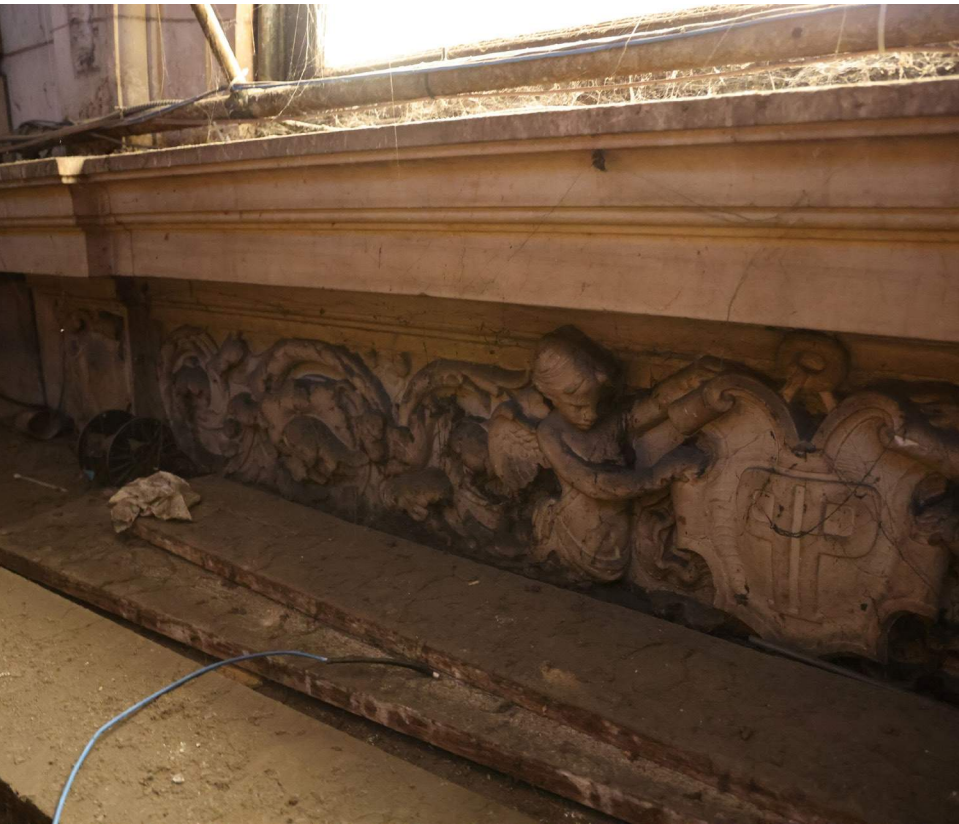
Stone Door Surround (Above Mail Room Enclosure)
