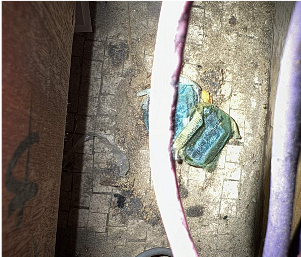
Mosaic Flooring (Under Front Desk)
