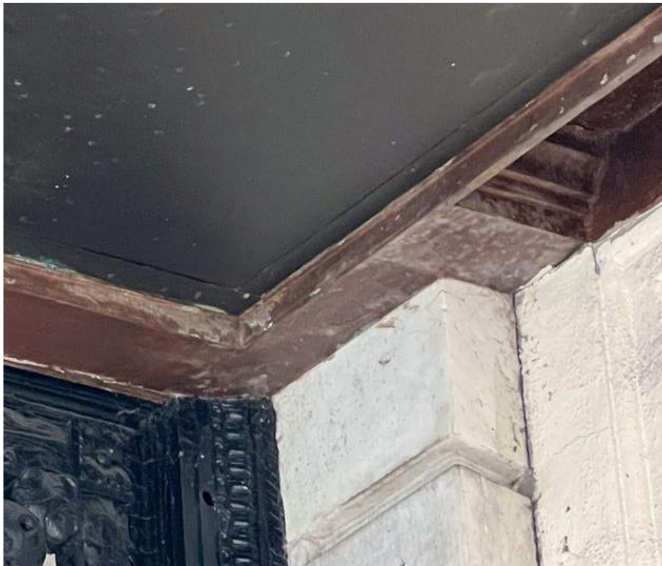
Canopy Molding (Above Mail Room Enclosure)
