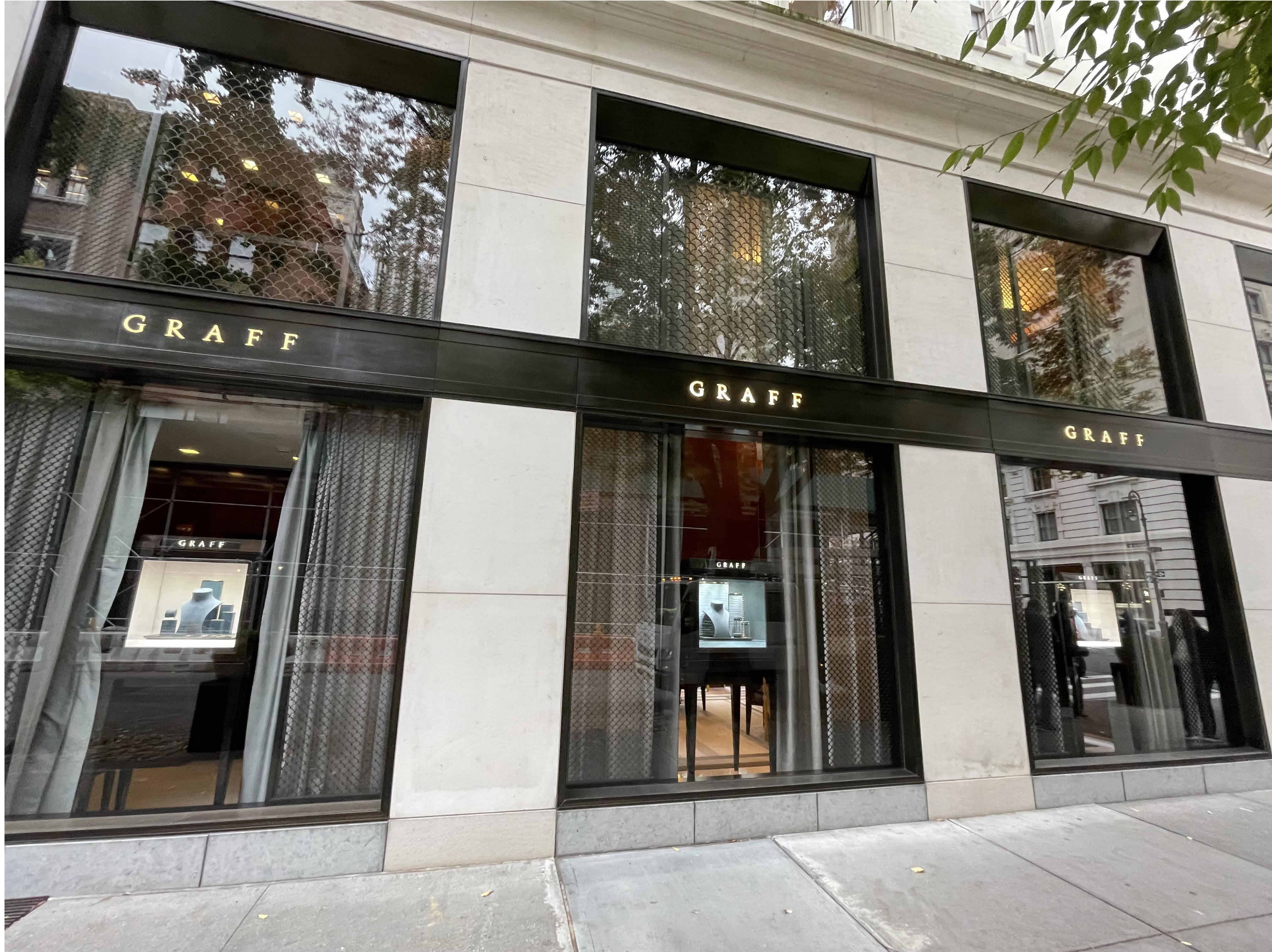
Detail of East 63rd Street storefronts.
