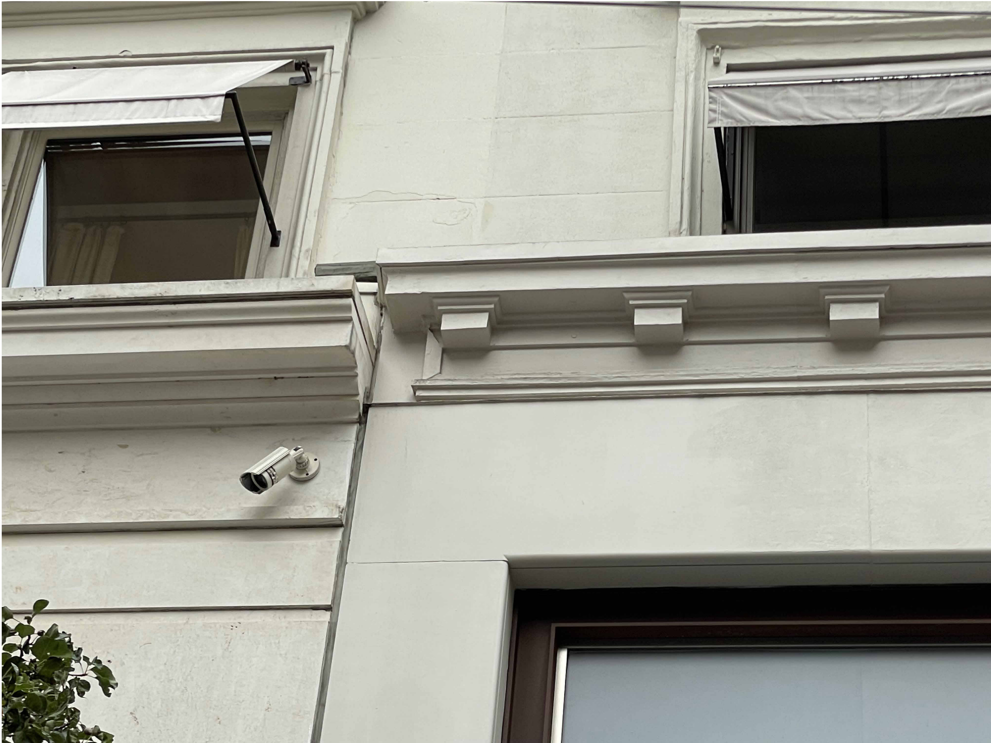
Detail of storefront cornices.
