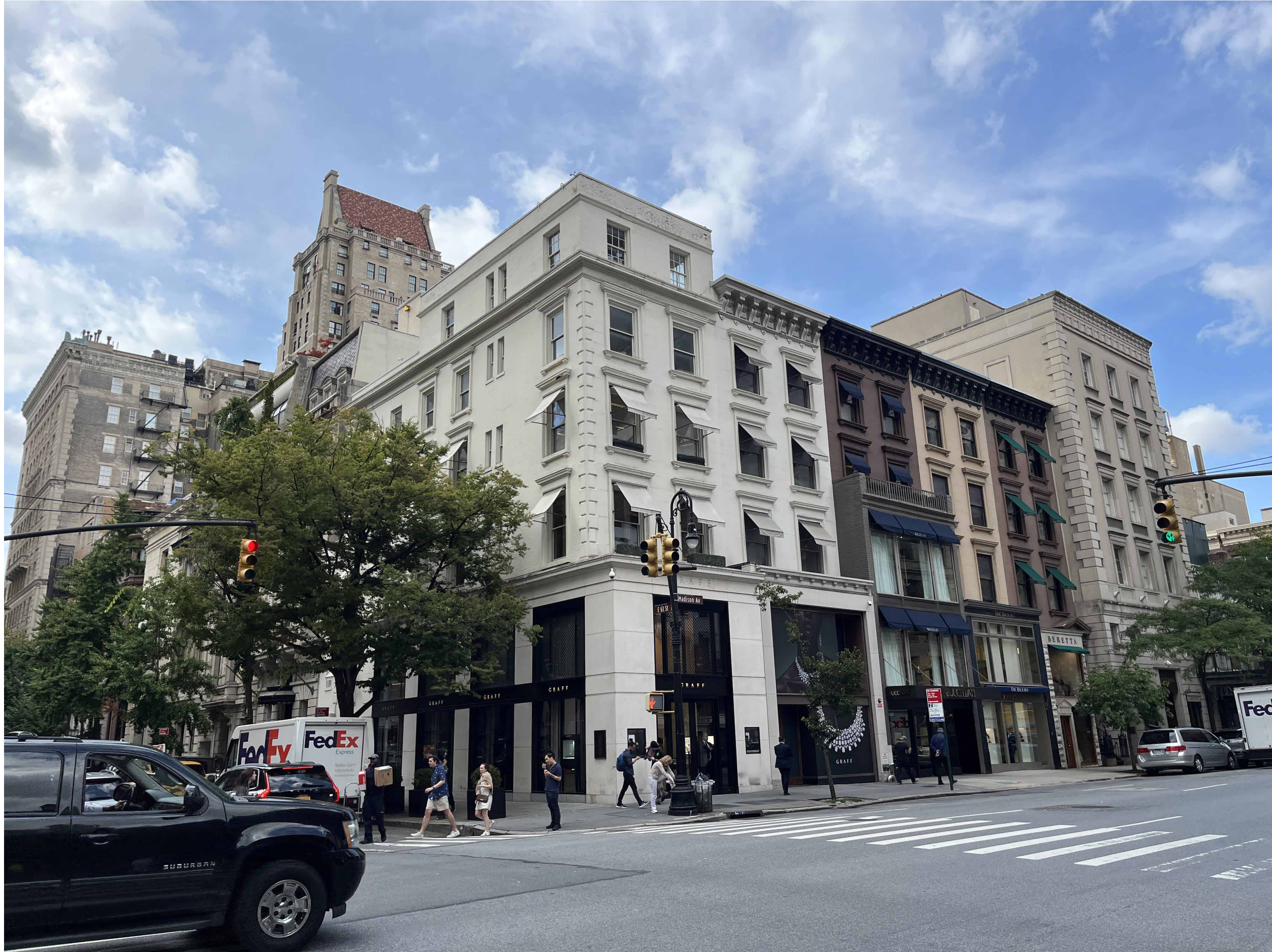
View of blockfront, looking northwest.
