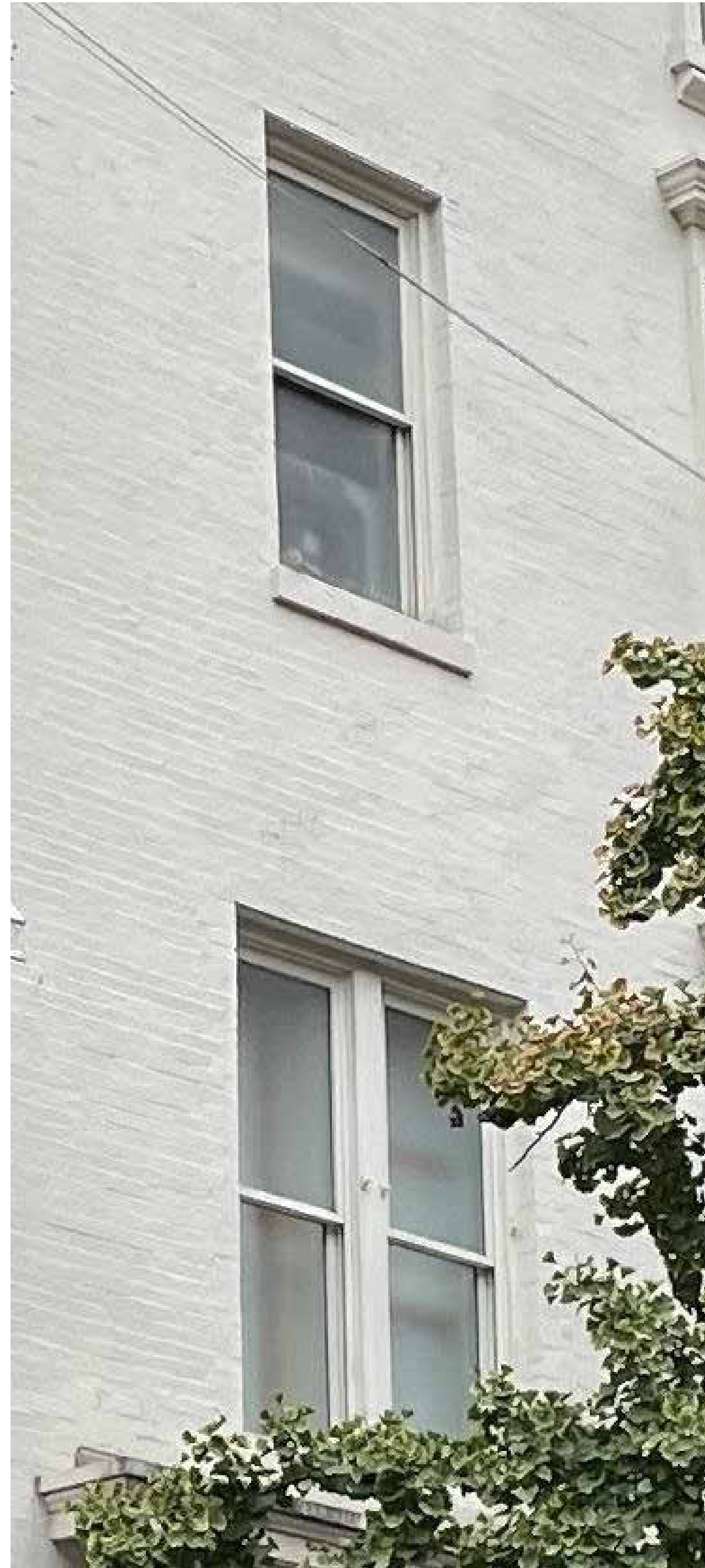
B - Non-historic window openings to be infilled
