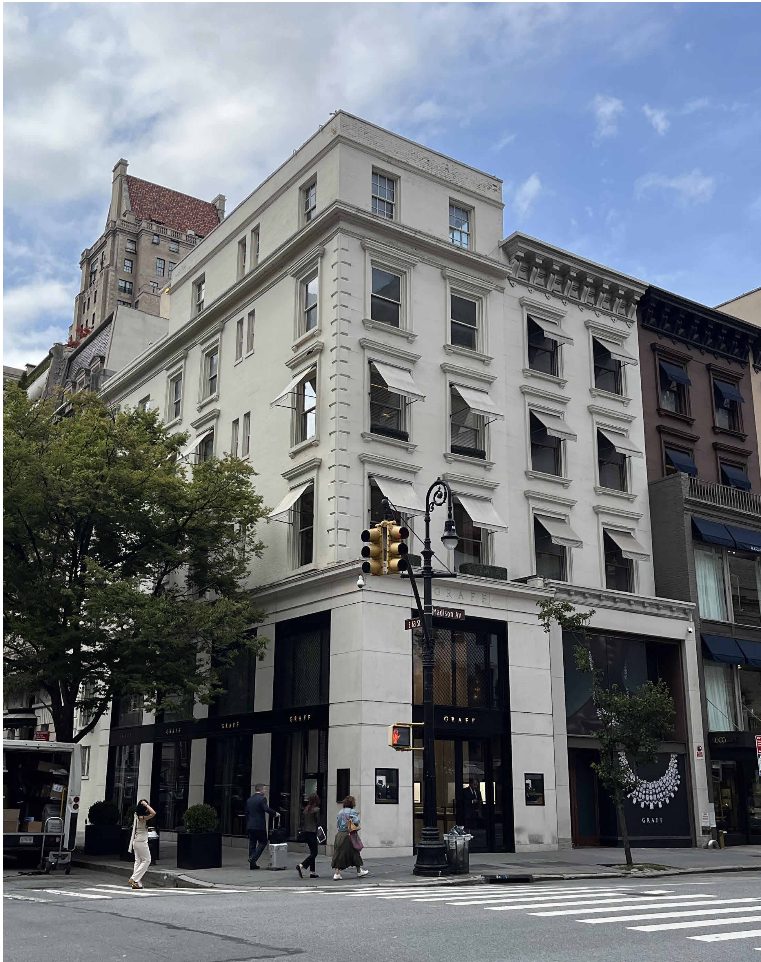
710-712 Madison Avenue, designed by Gage Inslee and built in 1871.
