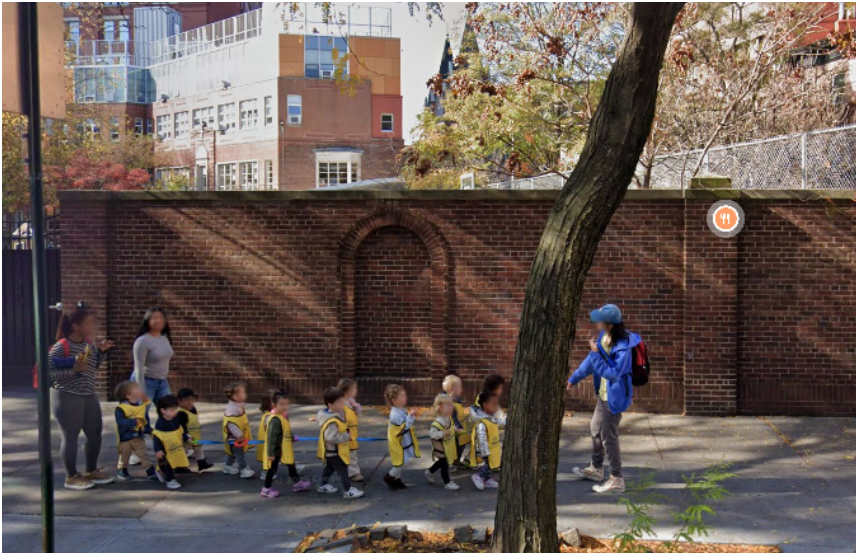
EXISTING BRICK WALL ALONG HUDSON ST
