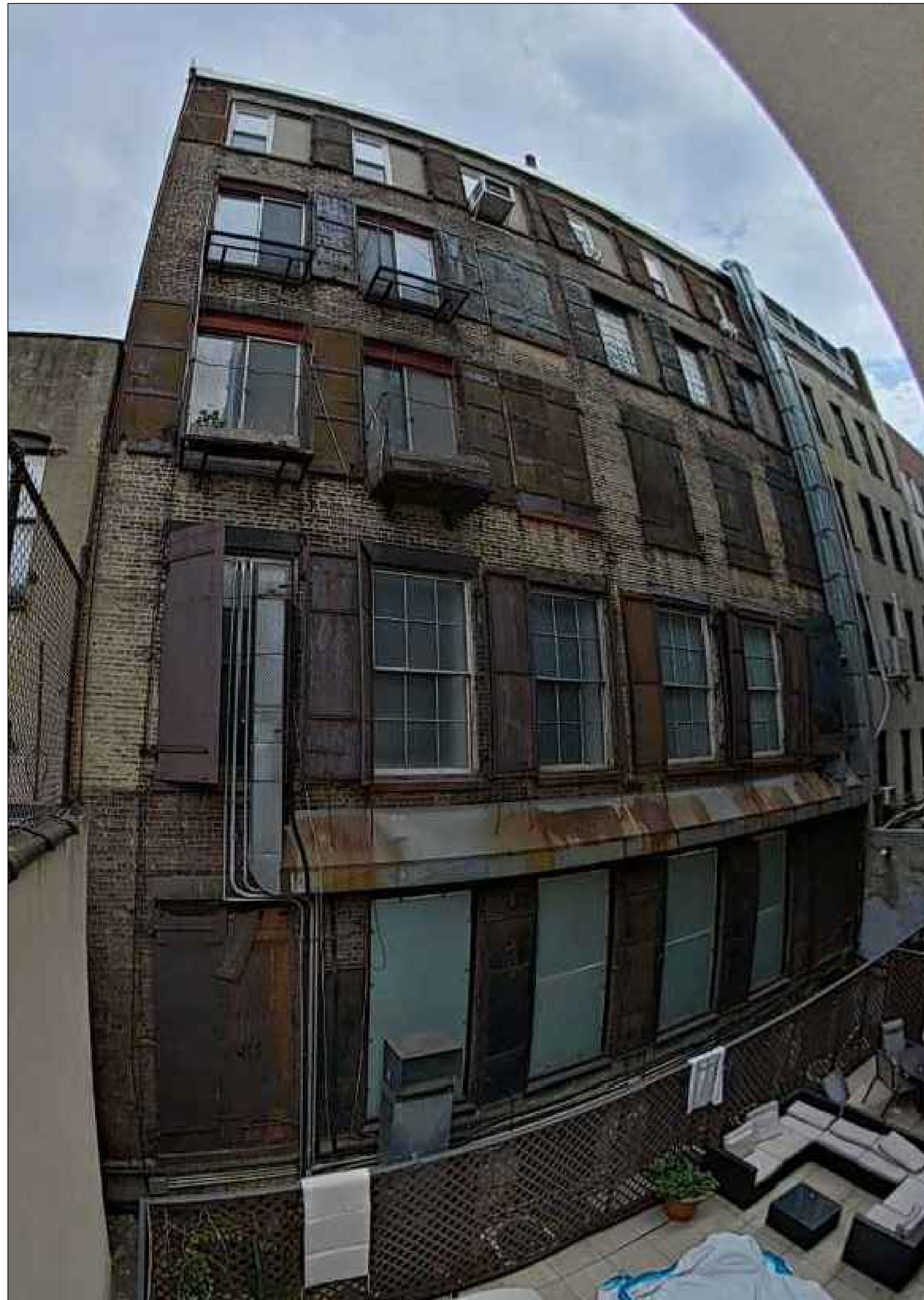
① Existing Rear Facade (West)
