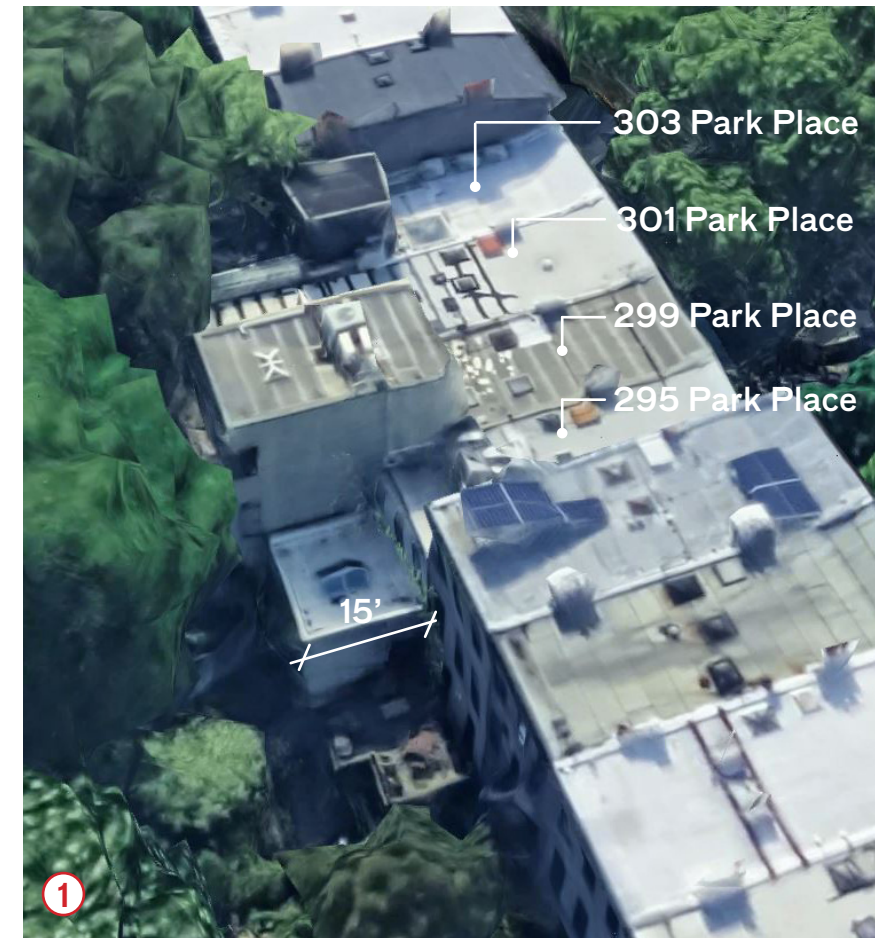
① Aerial View of Rear & Roof Additions on South of Block
