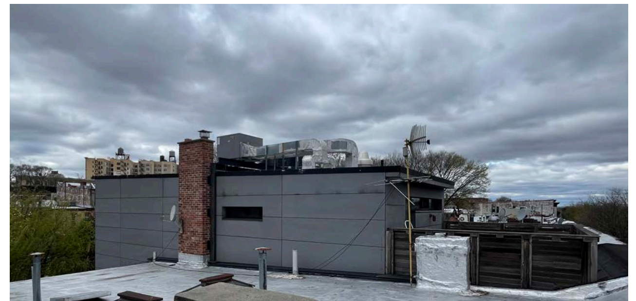
Neighboring 300 Prospect Place Roof Addition and Terrace
