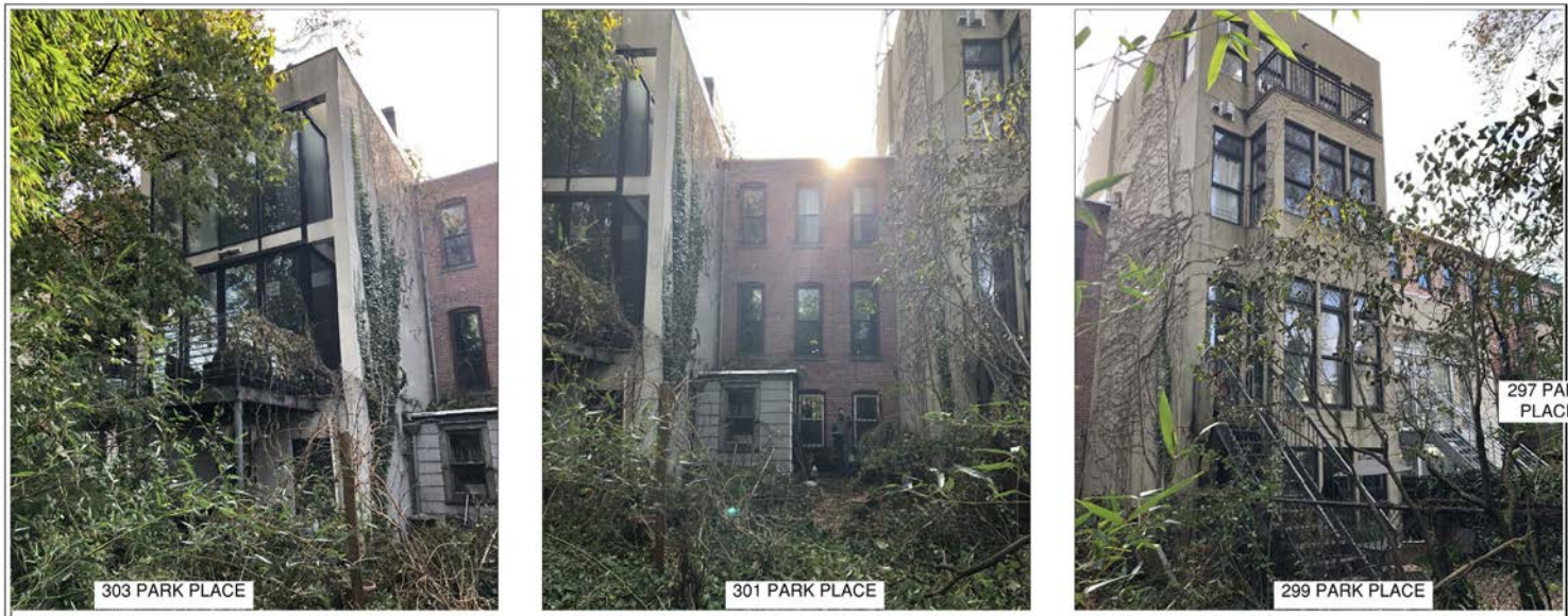
Rear View of Rear & Roof Additions on South of Block (from 2019 LPC hearing for 301 Park PI)
