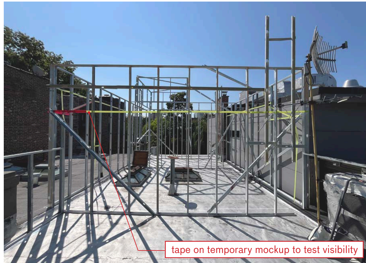
Proposed Roof Addition - Mockup
