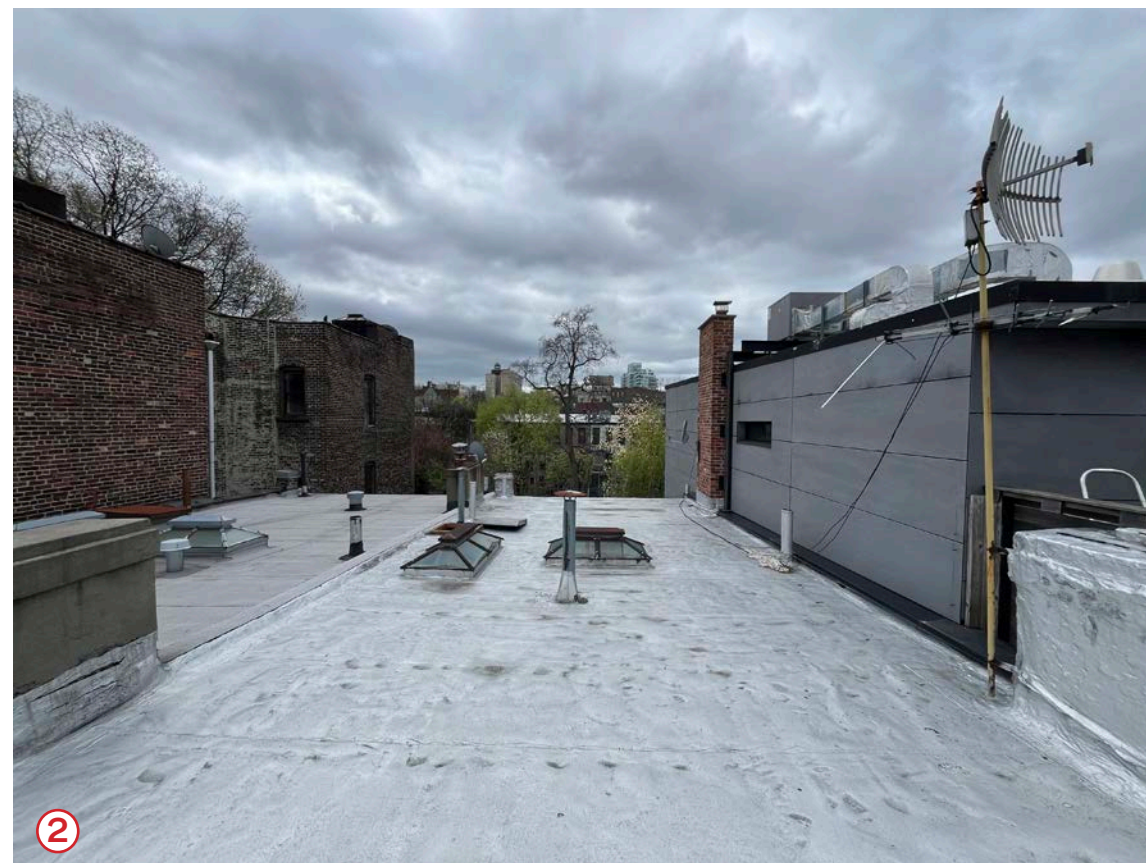
Existing Roof Photos
