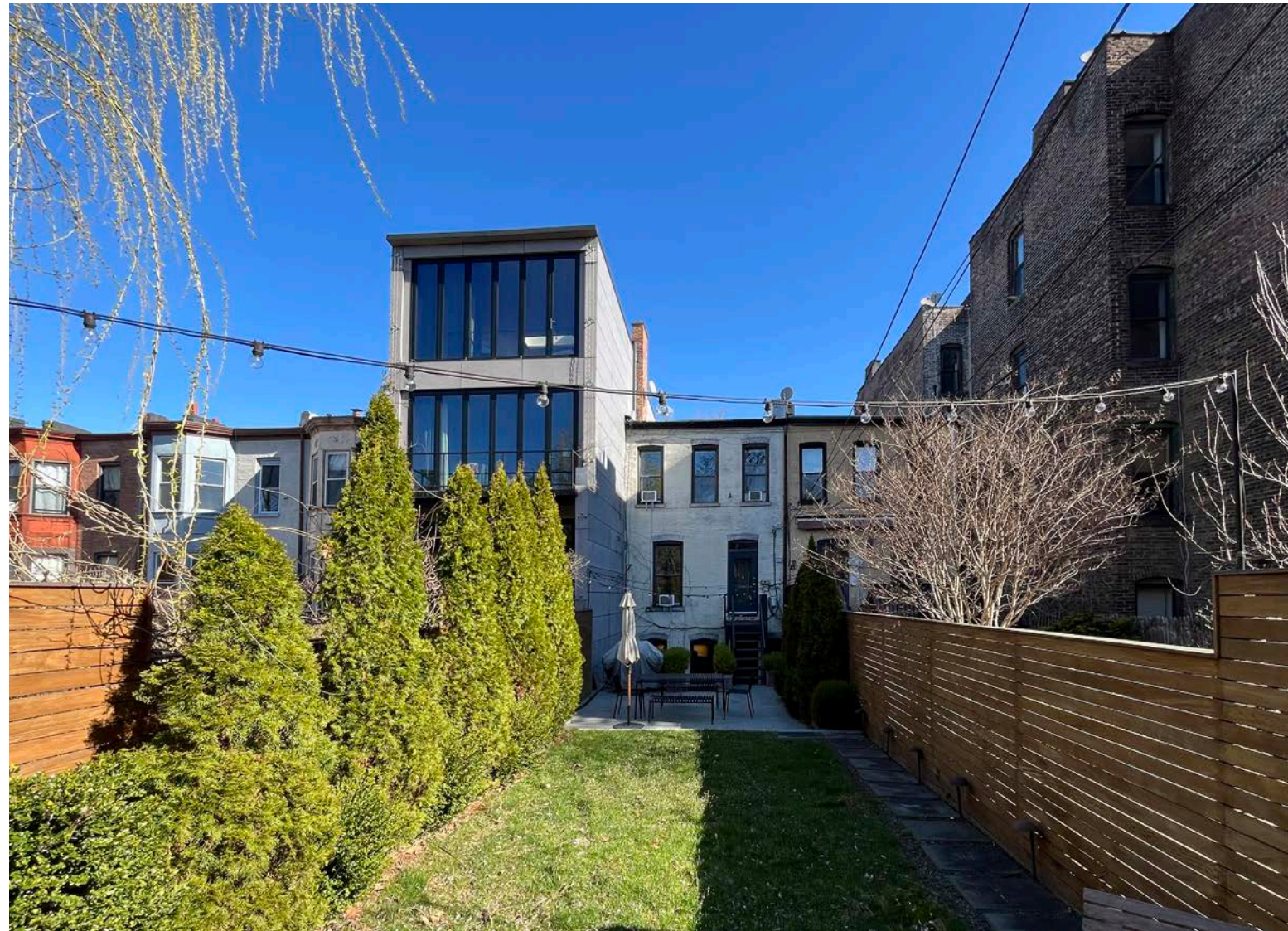
① Existing Rear Yard
