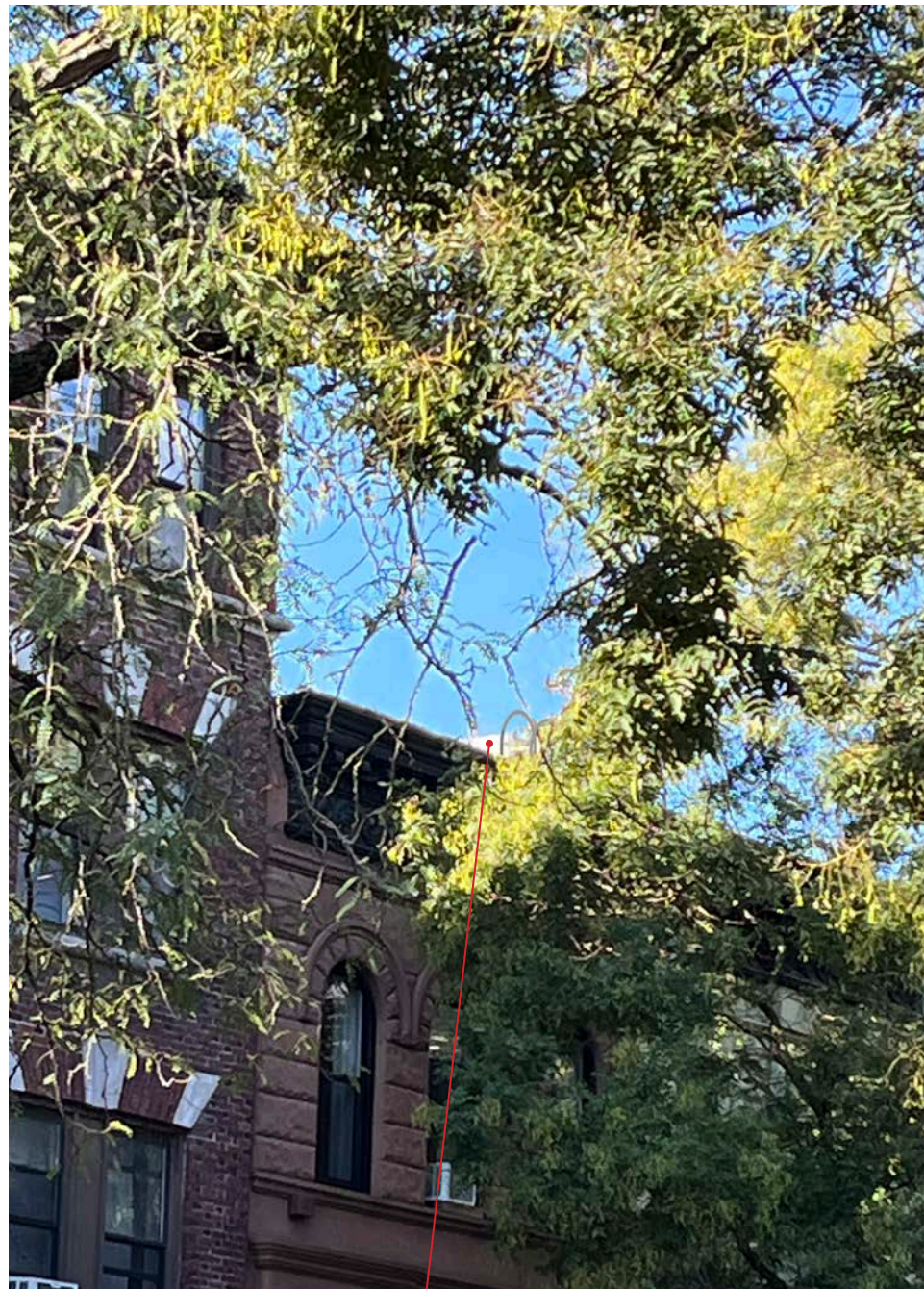
rooftop ductwork at 300 Prospect Place visible next to proposed fire ladder
