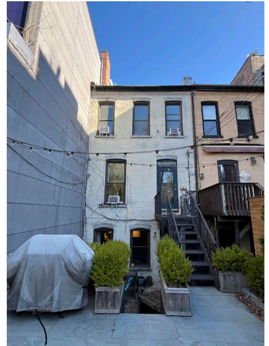
② Existing Rear Facade
