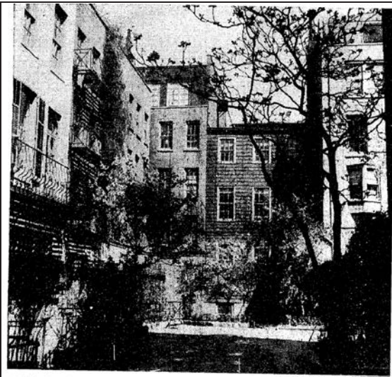
4 Bleeker Gardens is an enclave between Perry and Eleventh Streets, shared by surrounding homeowners. The "fronts" of the houses are on garden instead of street side.
