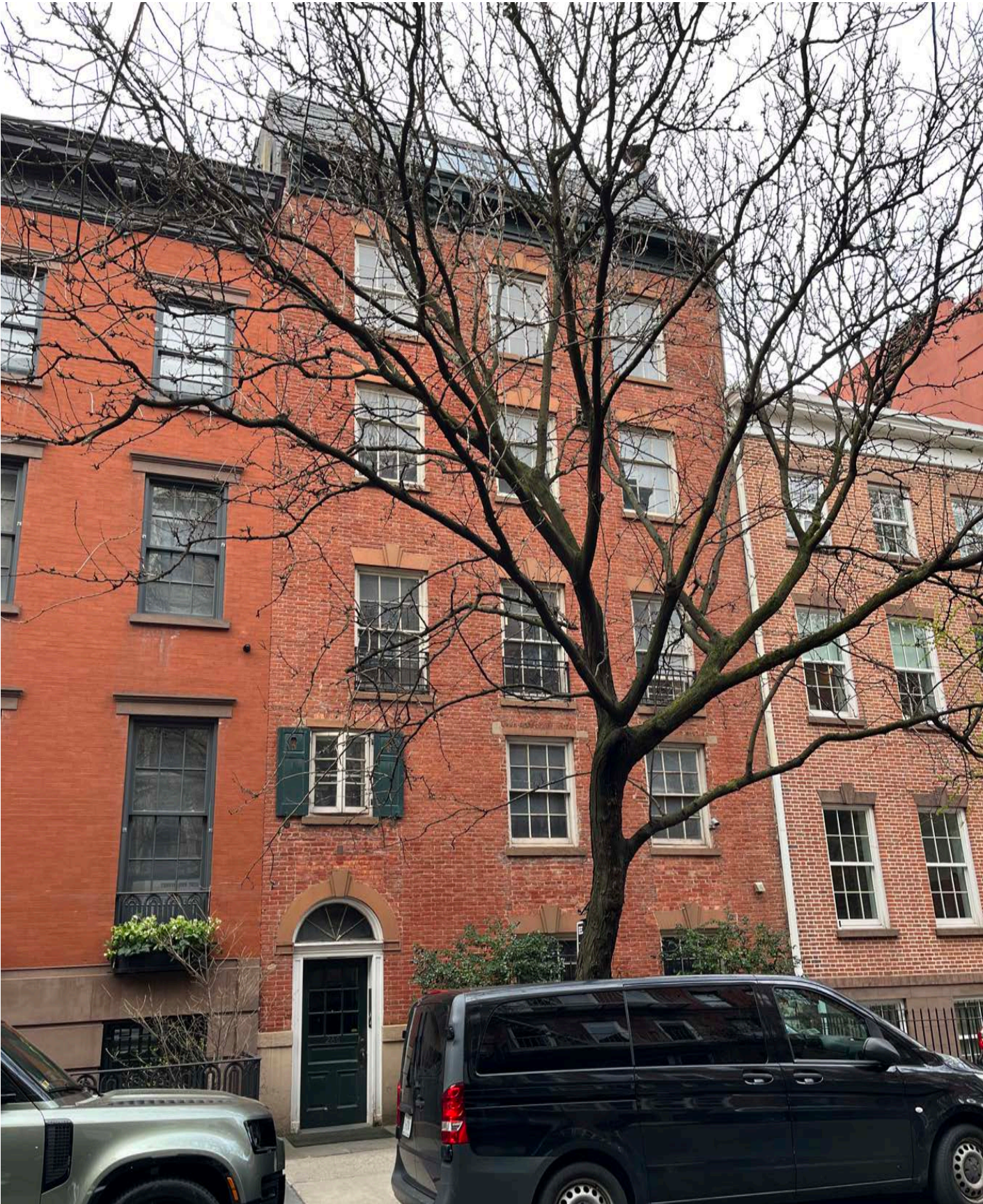
1. EXISTING FACADE OF 280 WEST 11TH STREET
