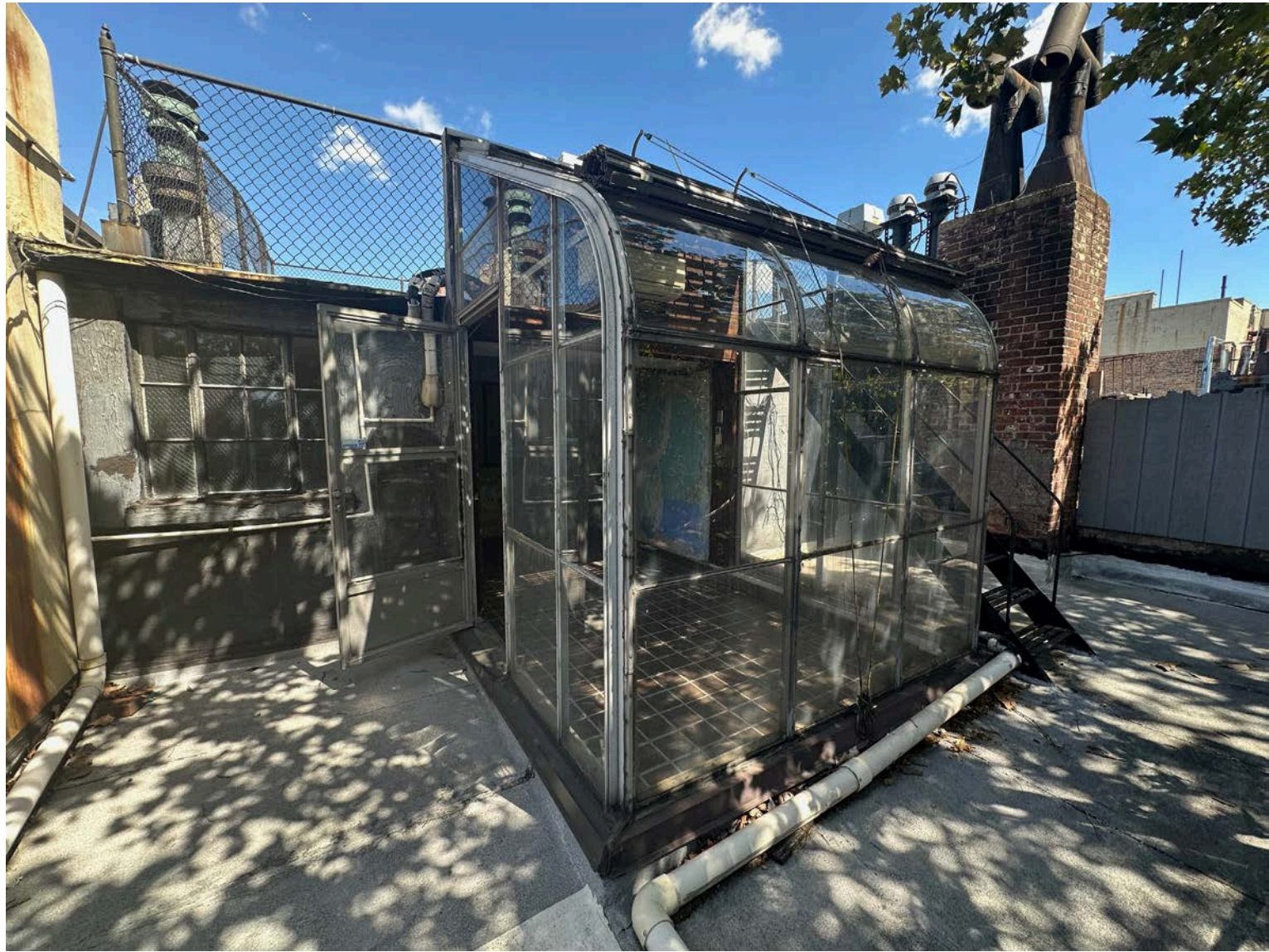
1. 5TH FLOOR REAR TERRACE LOOKING NORTH EAST
