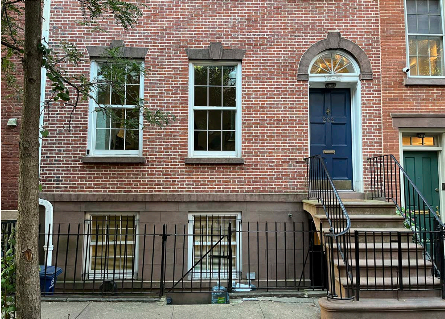
FACADE & AREAWAY @ 282 W 11TH ST.
