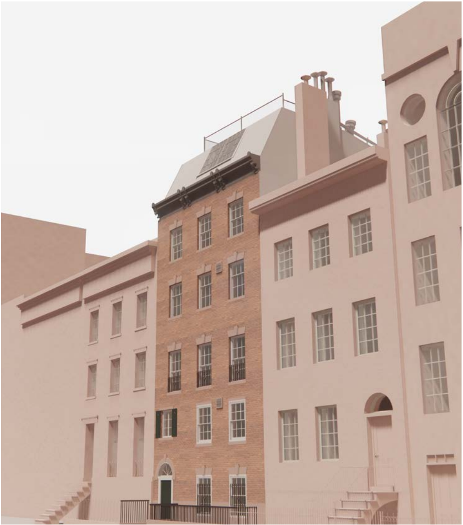
VIEW 1: W 11TH ST. +30' | EXISTING
