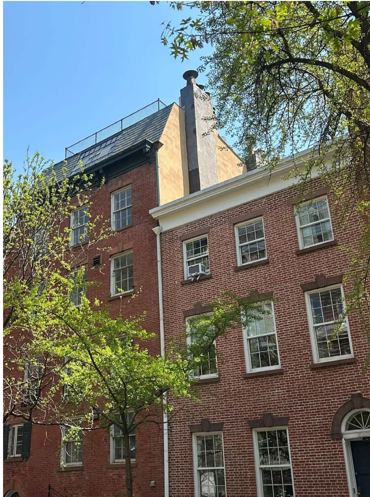
VIEW FROM W. 11TH STREET
