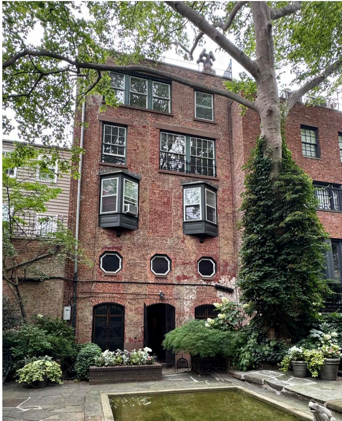
1. REAR FACADE OF 280 WEST 11TH STREET
