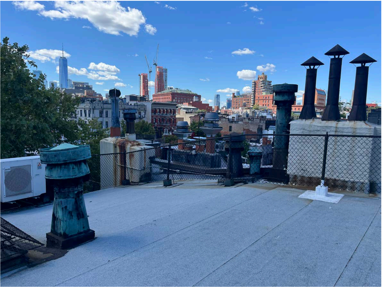
2. UPPER ROOF LOOKING SOUTH WEST
