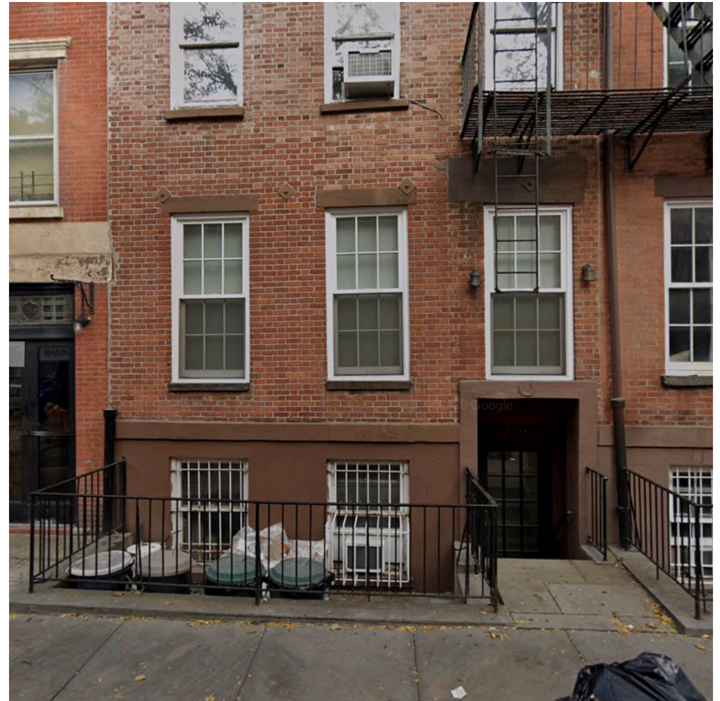
279 WEST 12TH STREET AREAWAY (BUILT 1828-1830)
