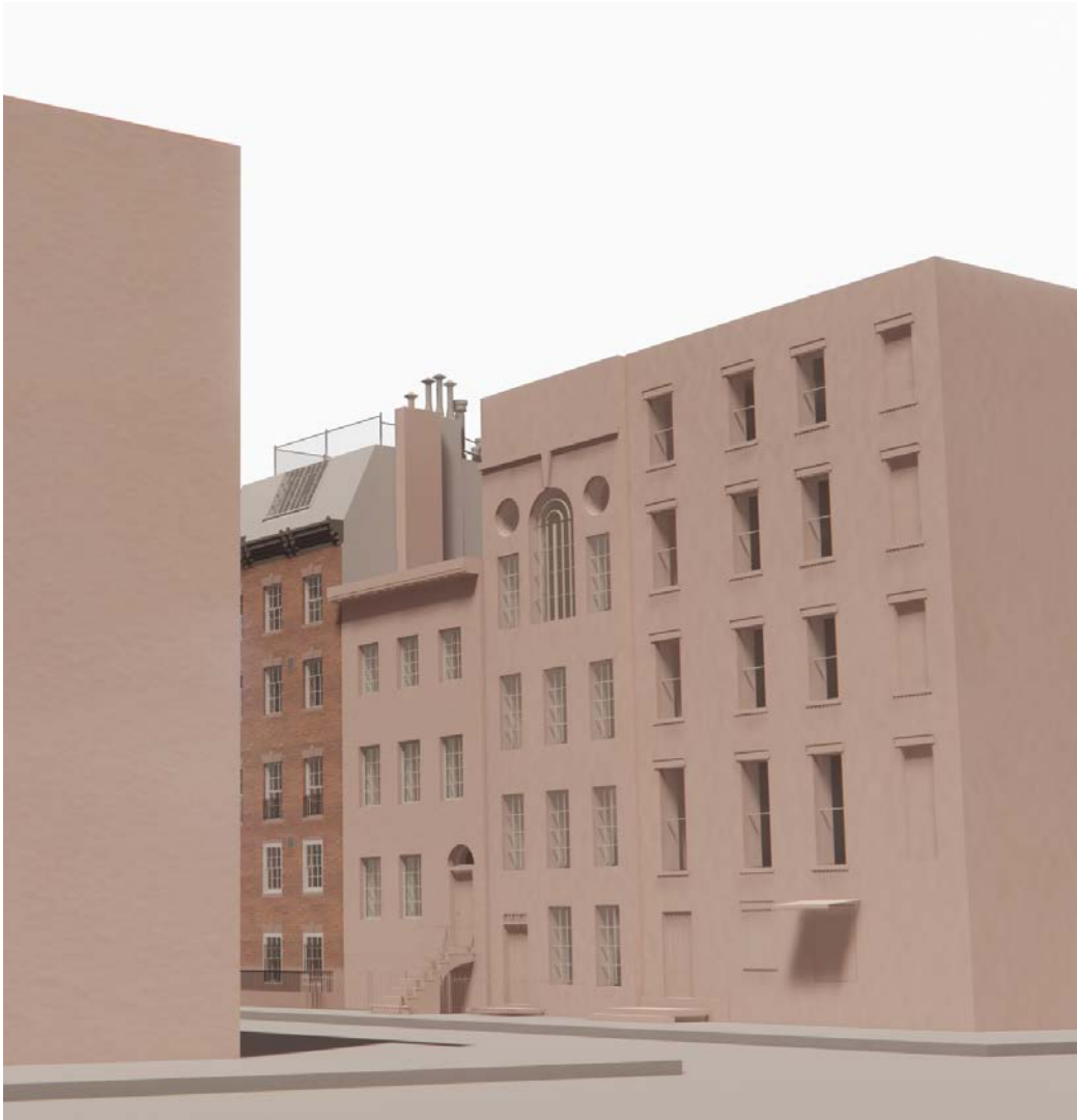
VIEW 4: BLEECKER ST 0' | EXISTING
