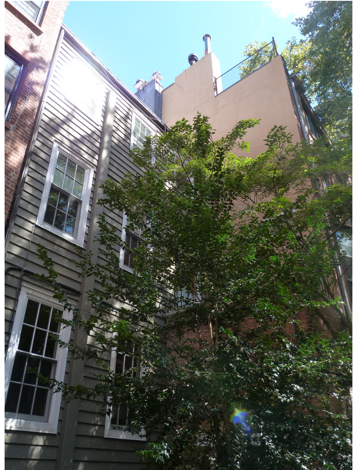
VIEW FROM REAR YARD
