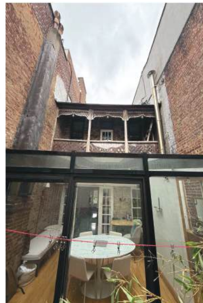
PHOTO 2: WEST VIEW (EXISTING REAR FACADE)
