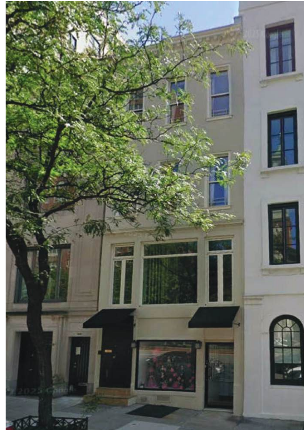
1143 PARK AVENUE CURRENT FRONT FACADE
