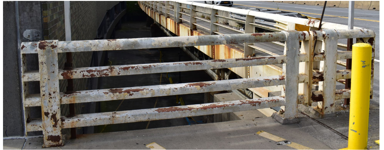
Rust buildup from long-term use
