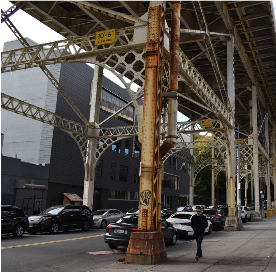
Rust buildup from long-term use
