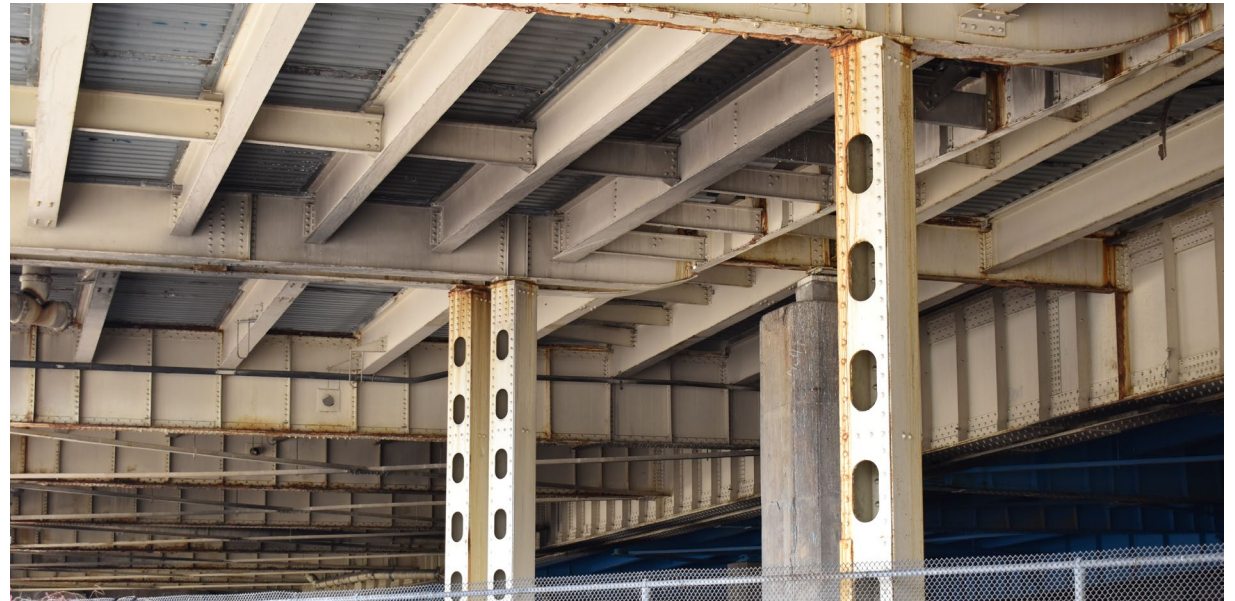
Rust buildup from long-term use
