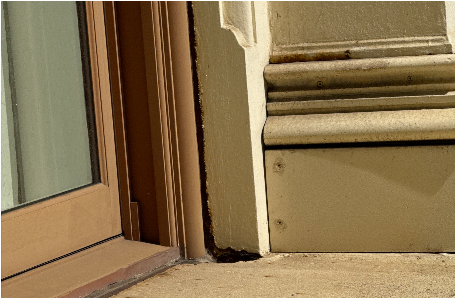
Scrape, prime and re-paint existing cast iron and install dutchman patches where there is evidence of spalls.
