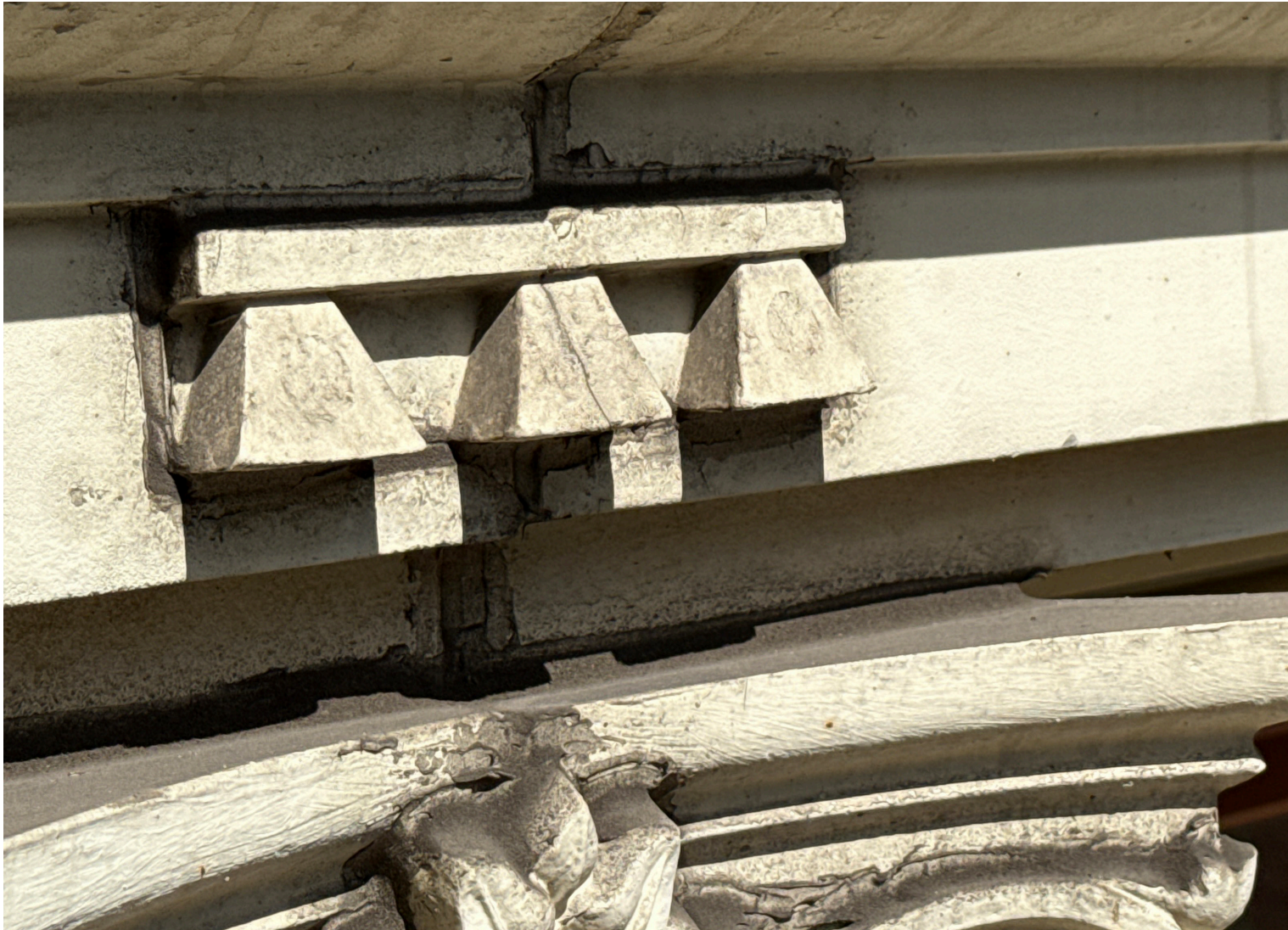
Perform crack repairs at existing GFRC
