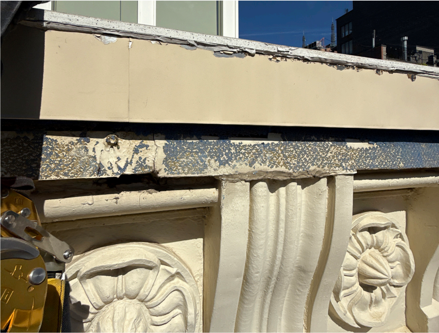
Remove exposed waterproofing along the east elevation.
