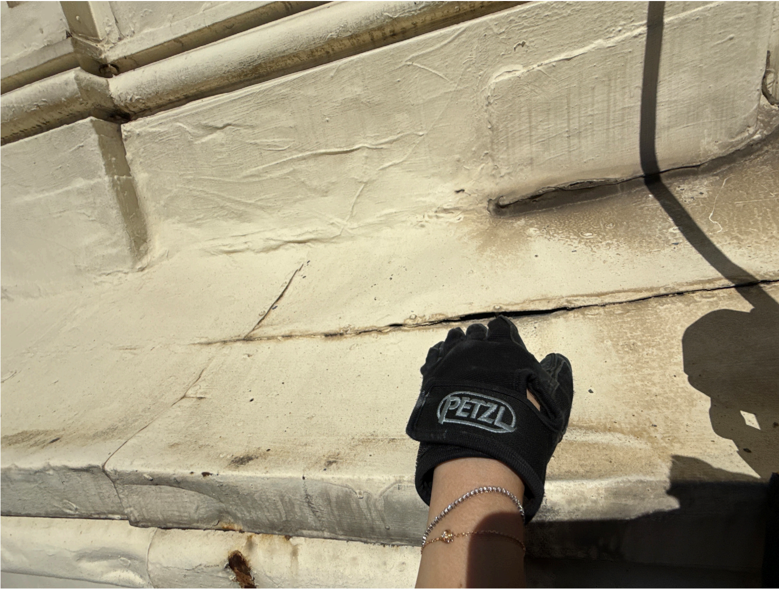
Repair the open solder joint using either soldering or mechanical fasteners.
