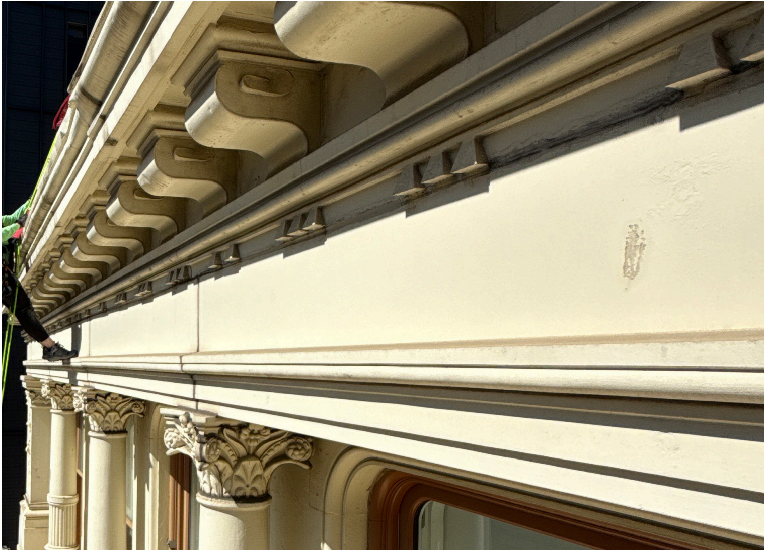
Scrape, prime and coat GFRC panels.
