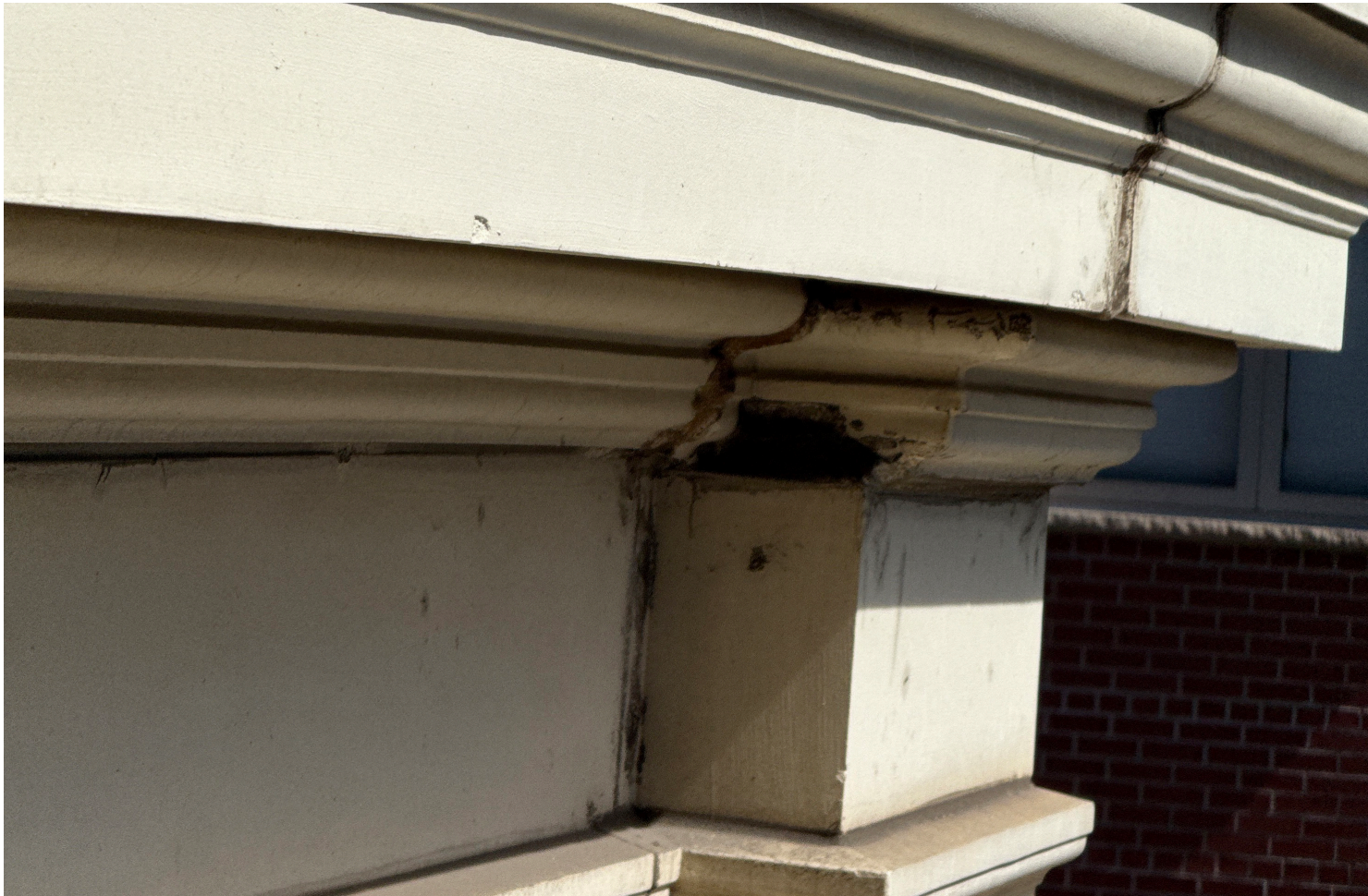
Install cast-iron dutchman patches where there is evidence of minor section loss.
