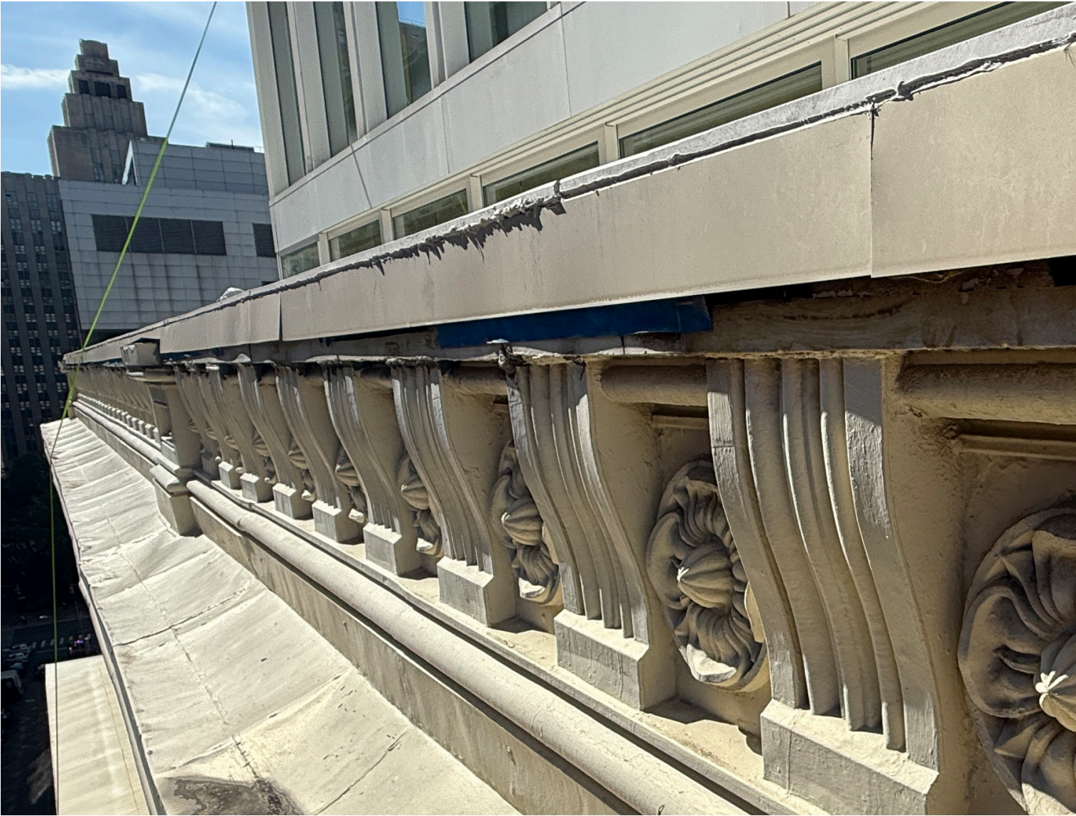
Remove exposed waterproofing along the north elevation.
