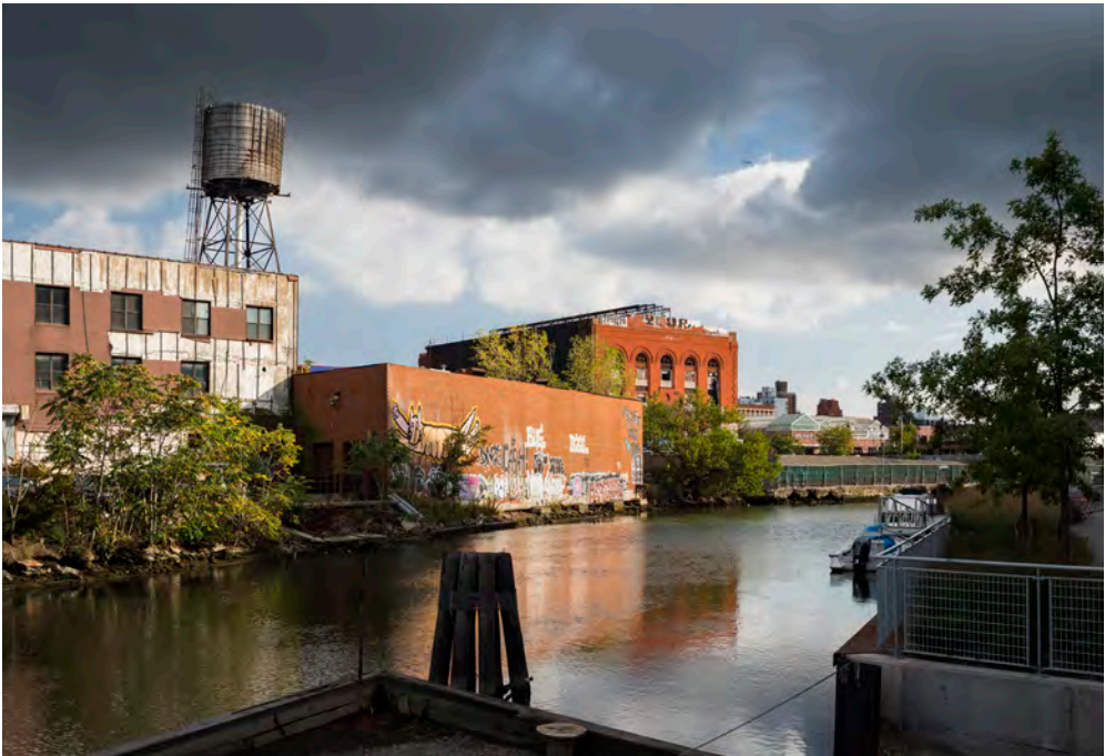
West Elevation from Gowanus Canal, North Elevation obscured by tarp
