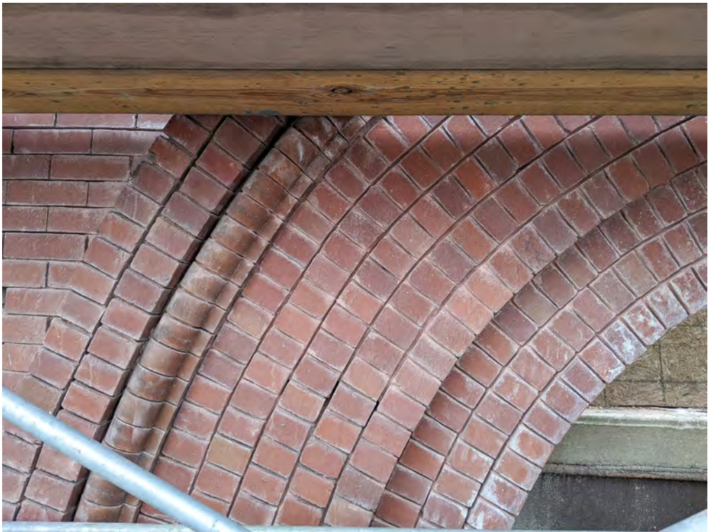
MASONRY REPOINTING REVIEW AT SEGMENTAL ARCHES
