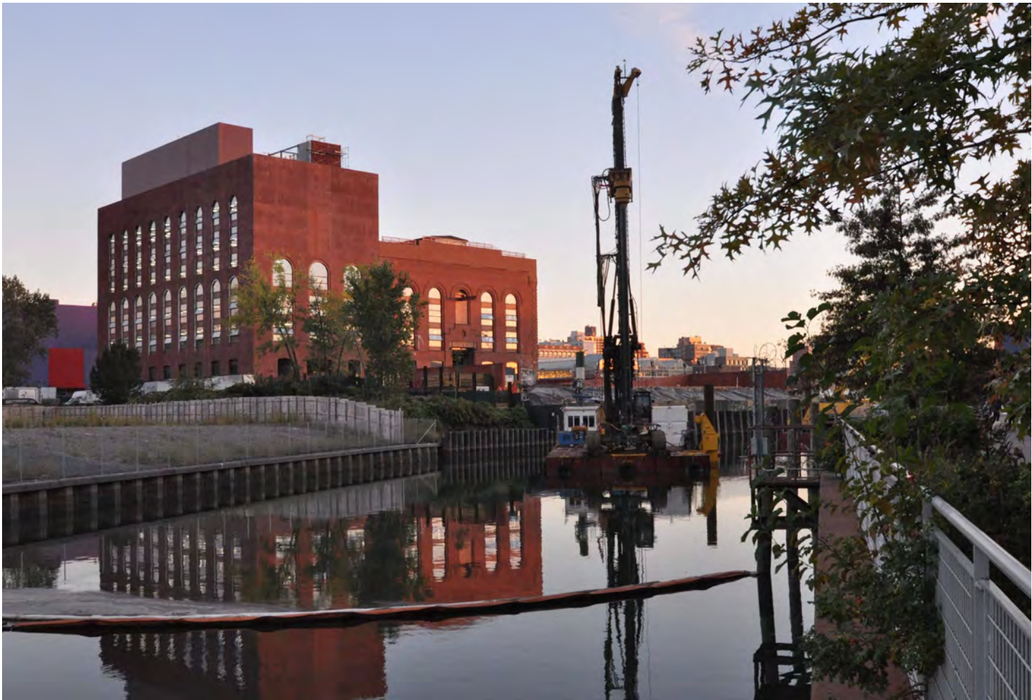
View from Gowanus Canal, North and West Elevations, 2023
