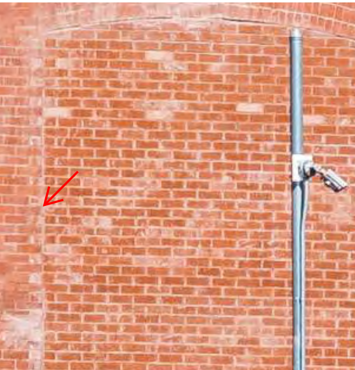
MASONRY INFILL AT EAST ELEVATION
