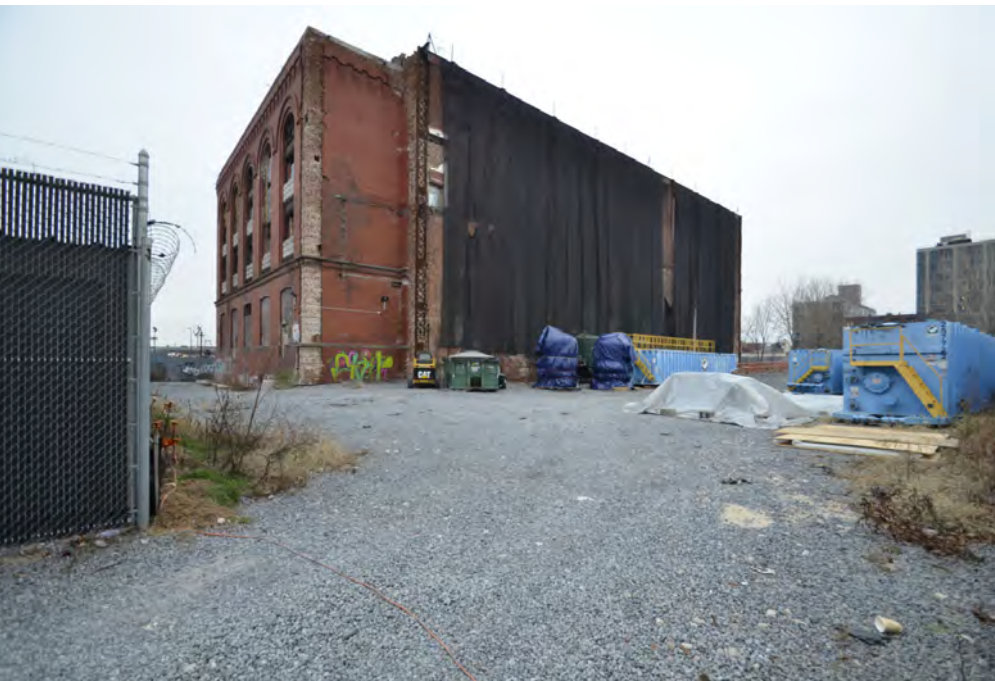
North Elevation behind protective tarp
