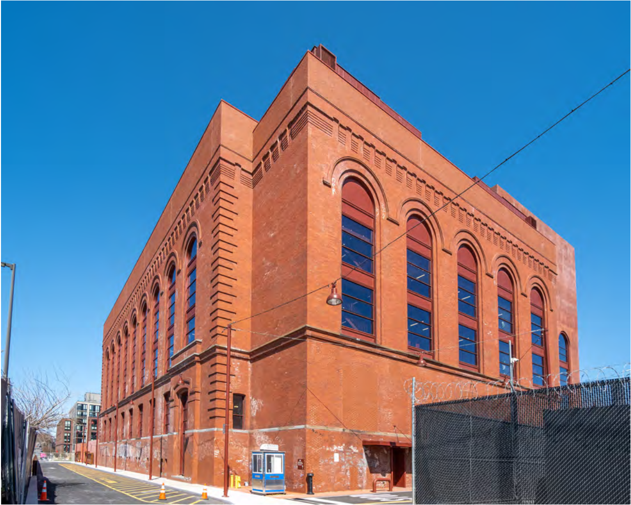
View of East and South Elevations Completed Work, 2017
