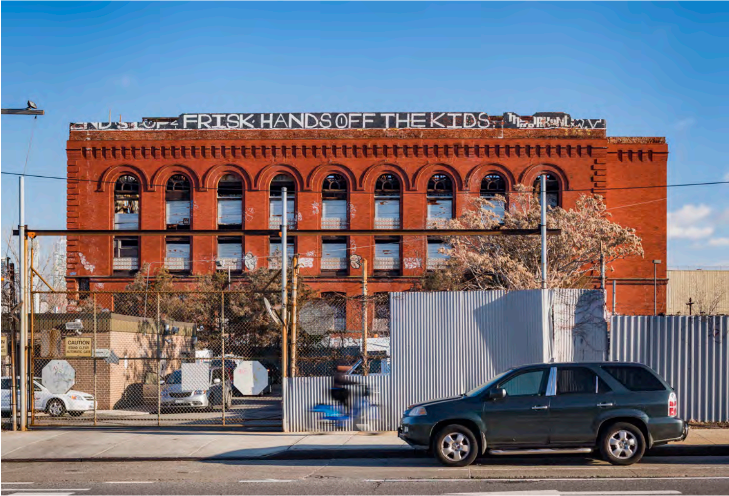
South Elevation showing deteriorated parapet condition, 2016
