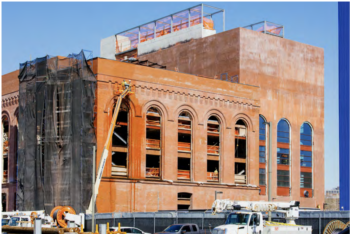
MASONRY CLEANING AND RESTORATION IN PROCESS
