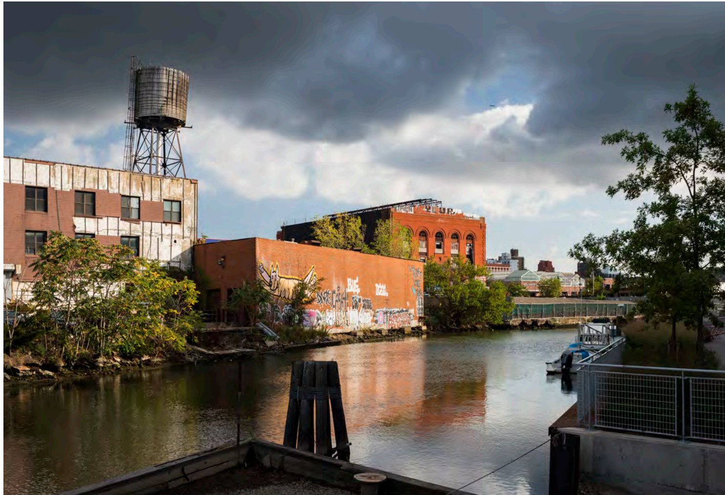
West Elevation from Gowanus Canal, North Elevation obscured by tarp, 2016
