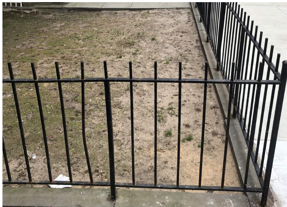
Existing Non-Historic Railing
