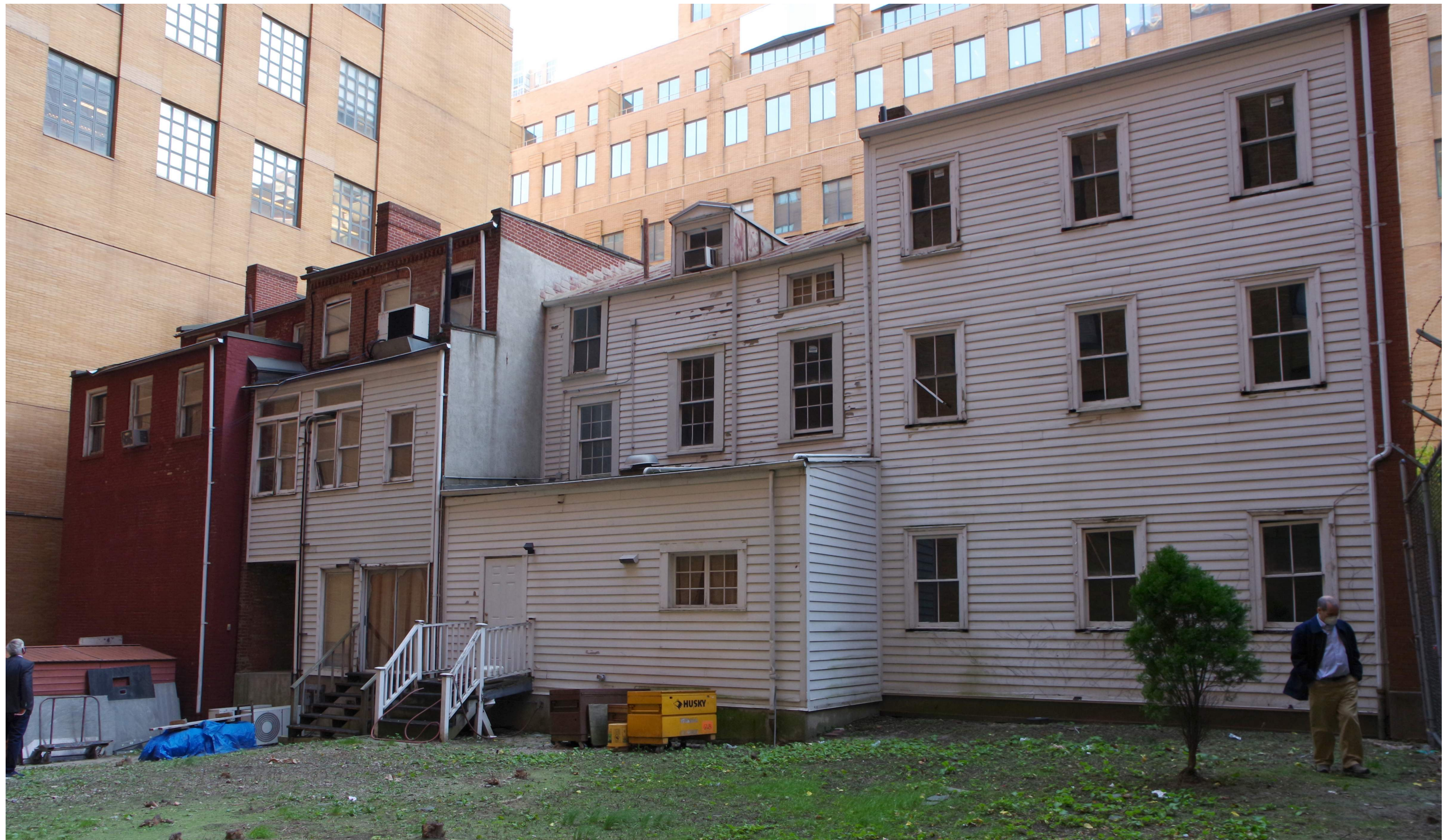
Back Facade Existing Conditions
