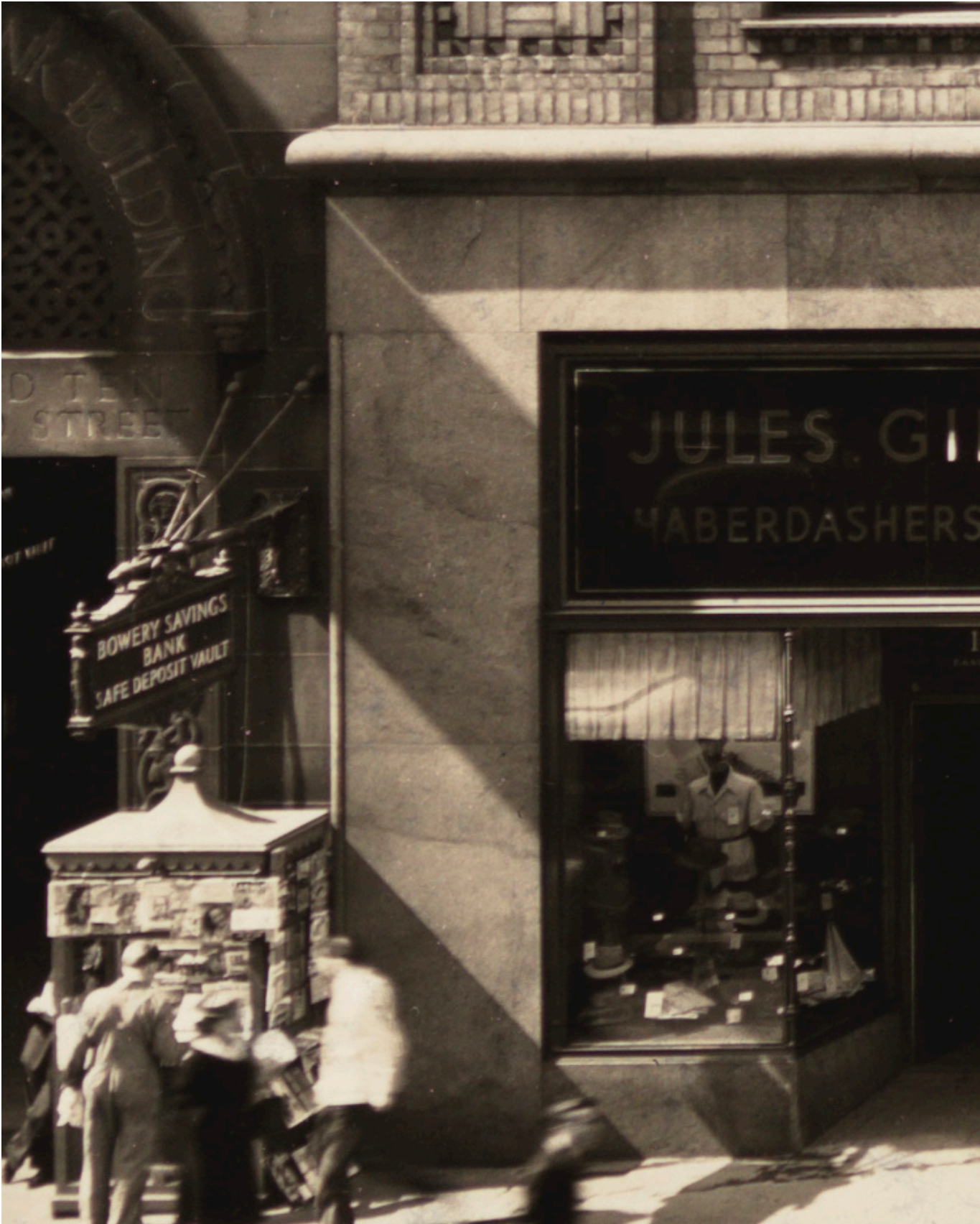
C. 1940 GRANITE PIER DETAILS MCNY
