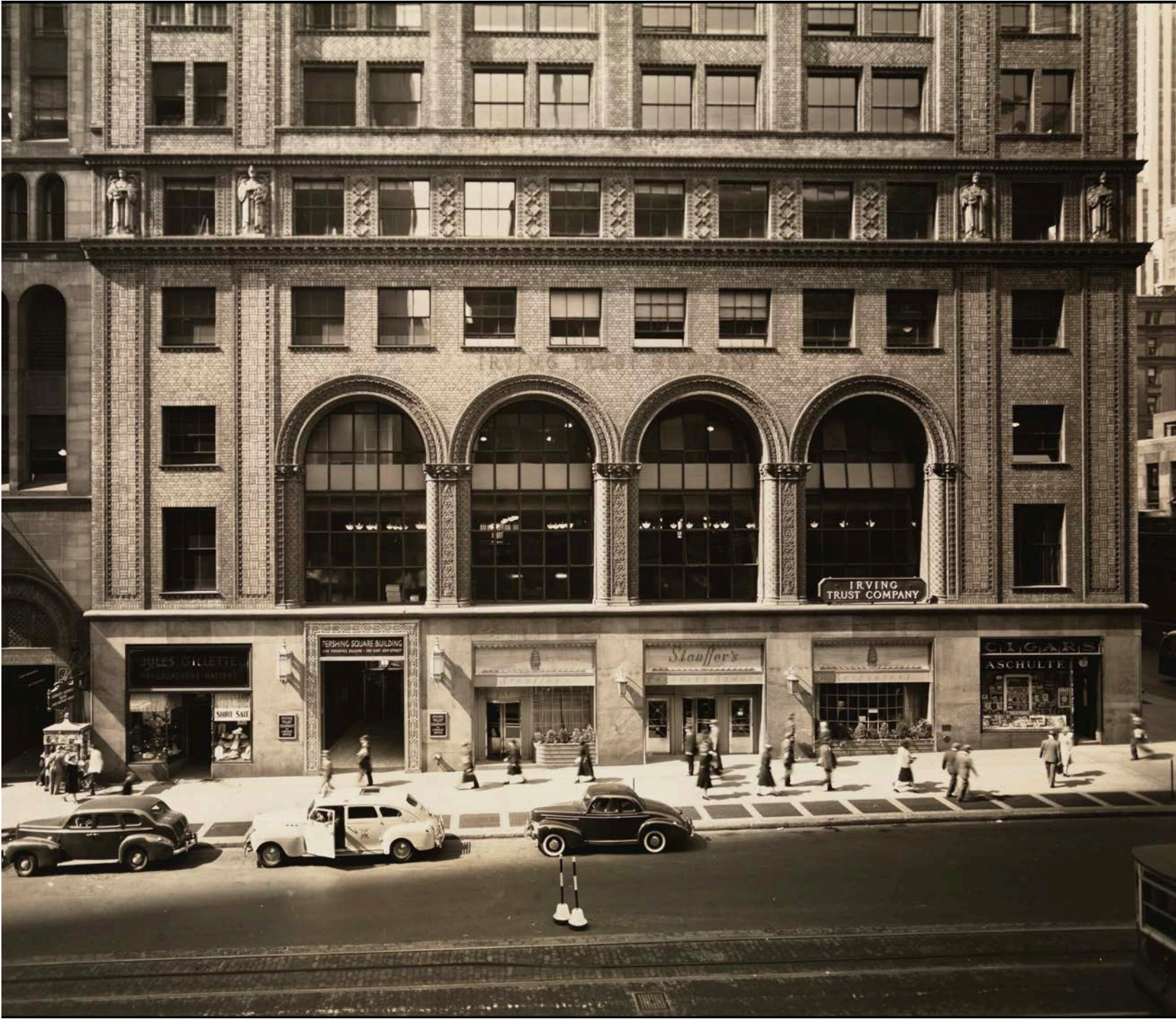
C. 1940 ENTRANCE DETAIL MCNY
