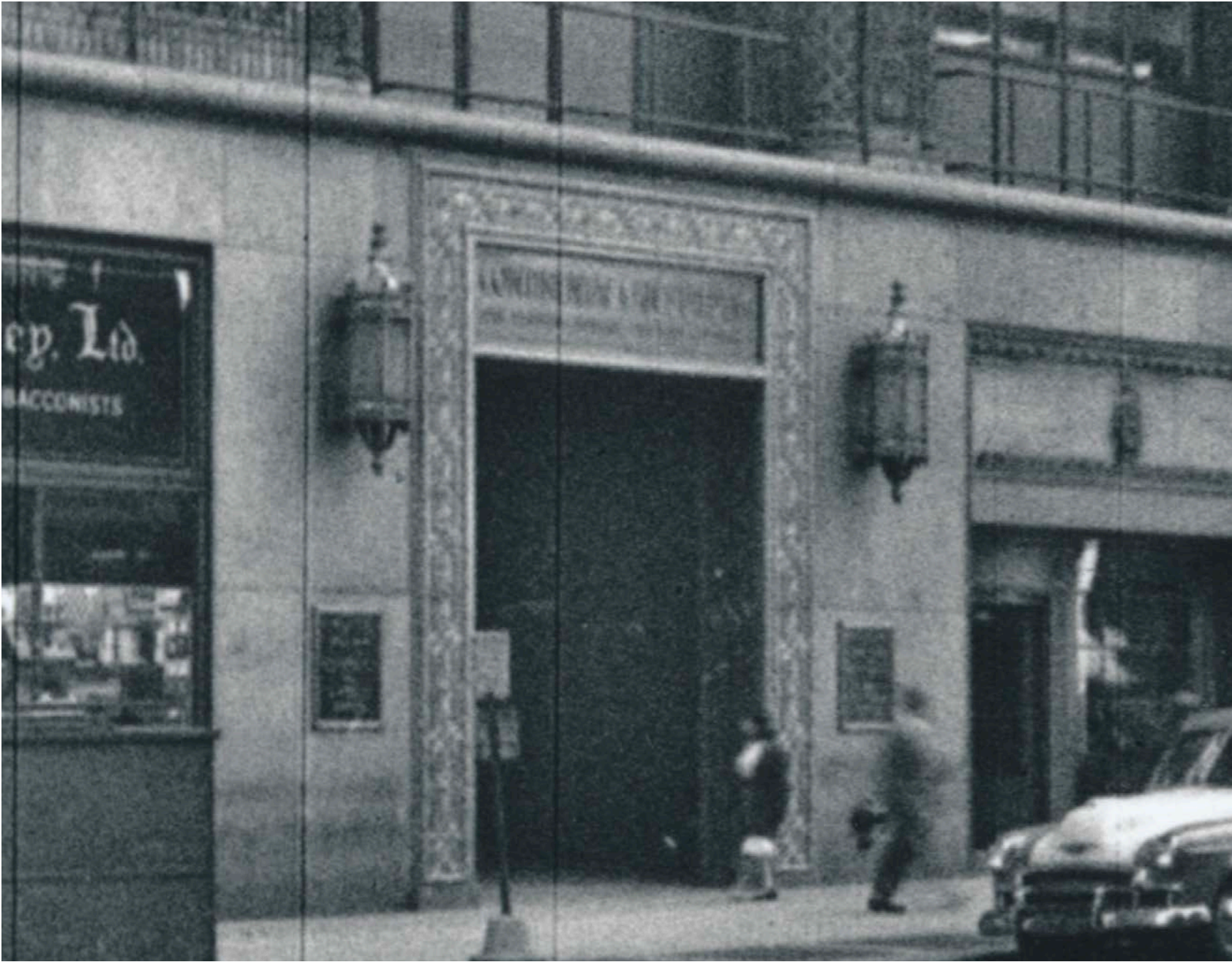
C. 1940 GRANITE PIER DETAILS MCNY
