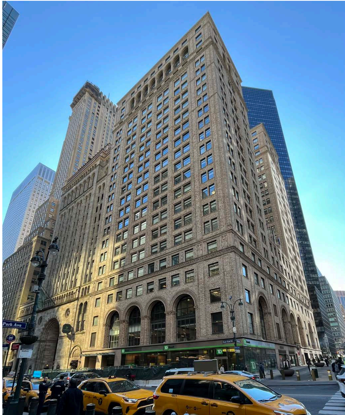
EXISTING CONDITIONS Northwest Corner of Building
