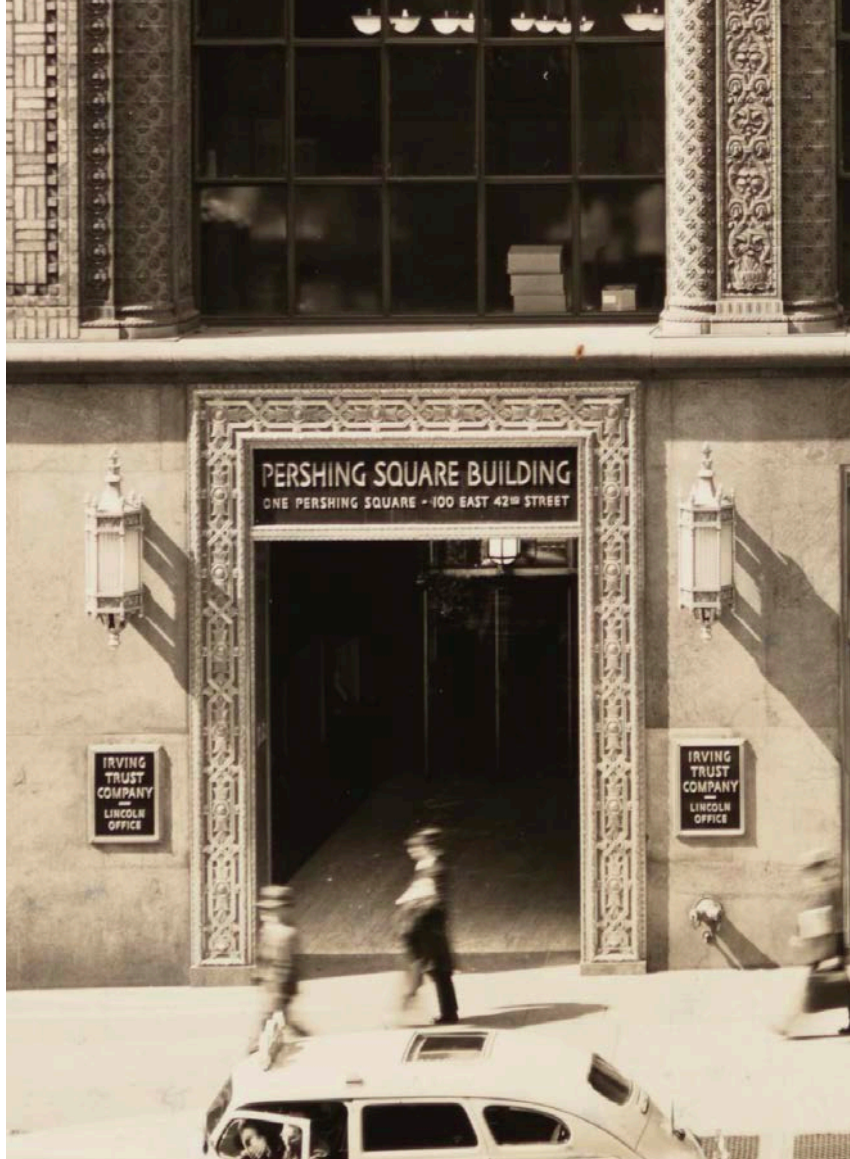
C. 1940 ENTRANCE DETAIL MCNY
