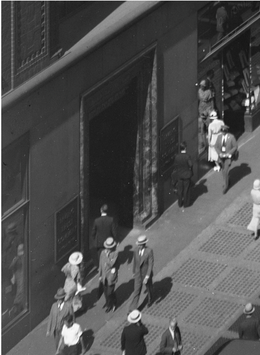
C. 1930 ENTRANCE DETAIL MCNY
