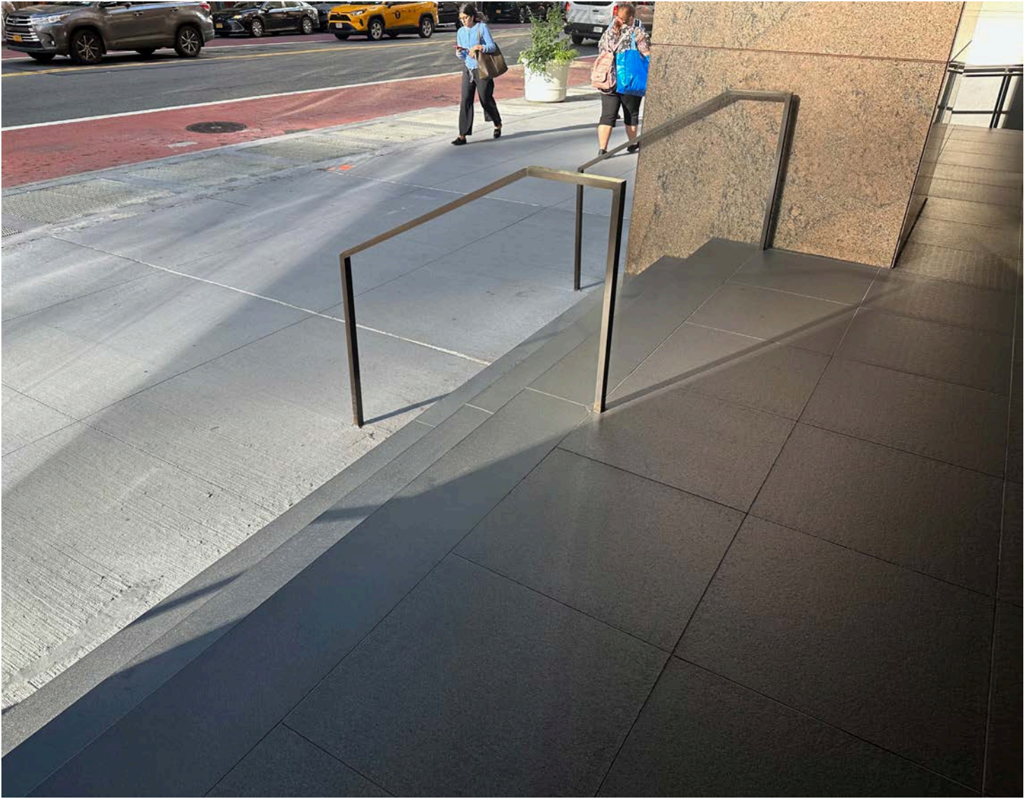
EXISTING RAILINGS AND STAIRS
