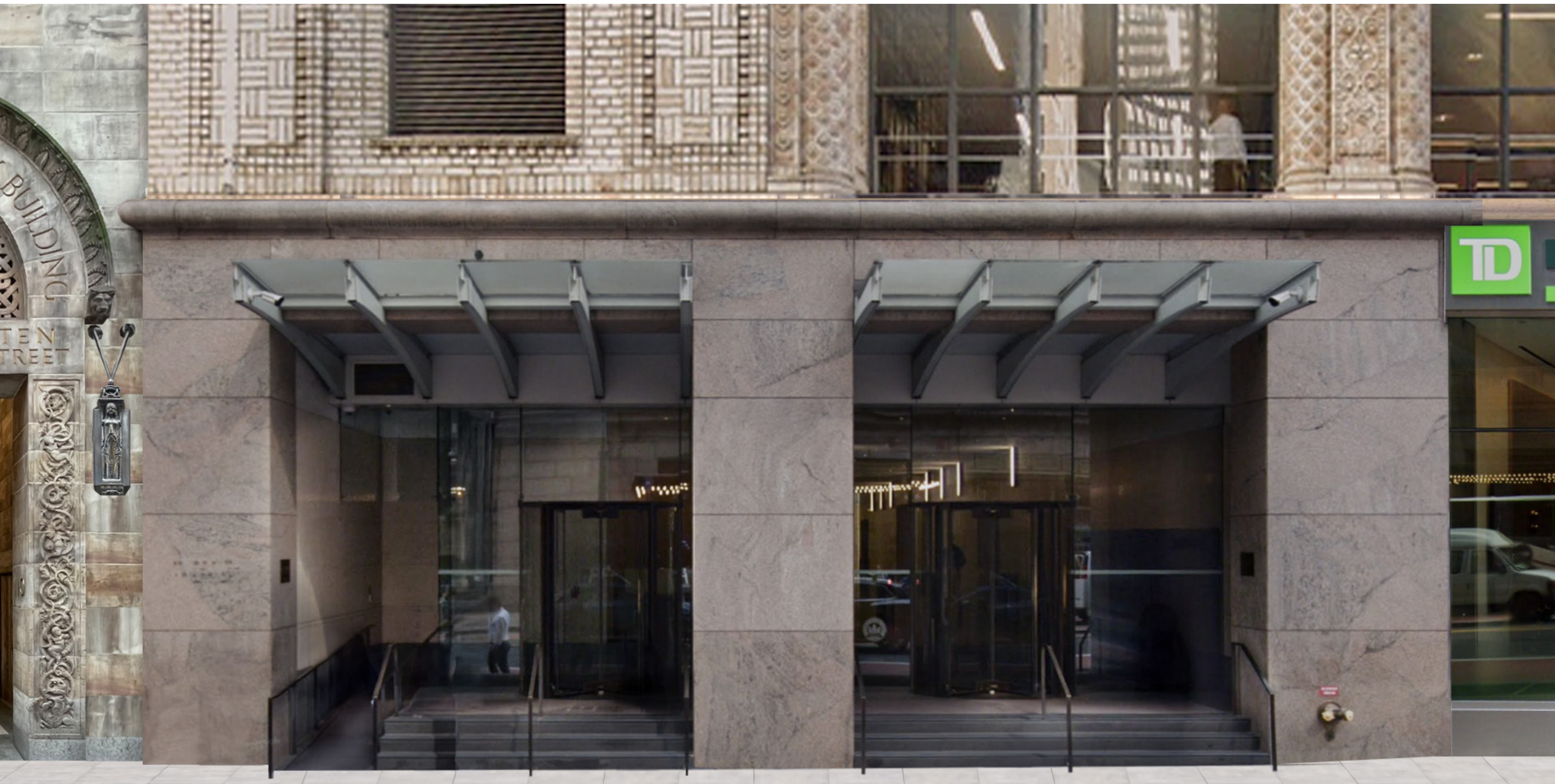
125 PARK AVENUE CURRENT ENTRY VIEW
