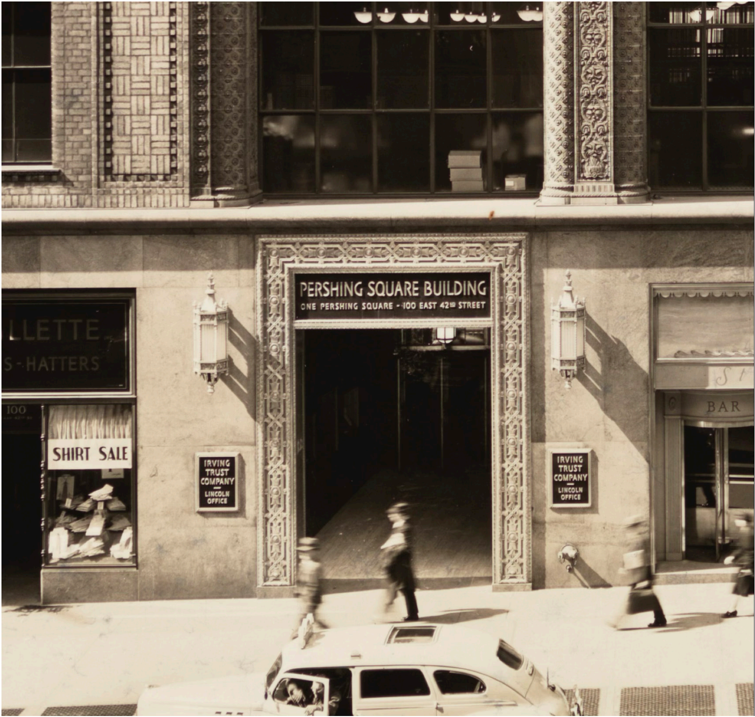
C. 1940 ENTRANCE DETAIL MCNY
