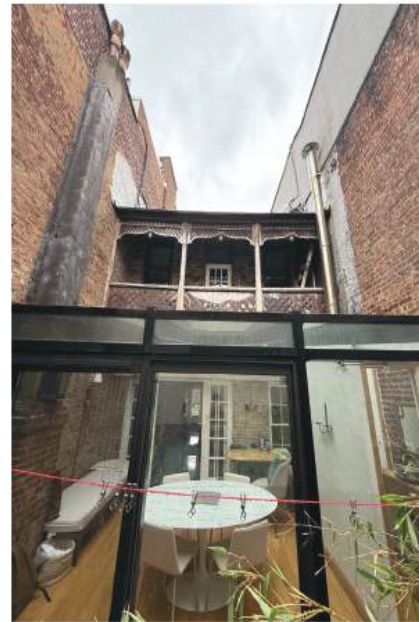
PHOTO 2: WEST VIEW (EXISTING REAR FACADE)
