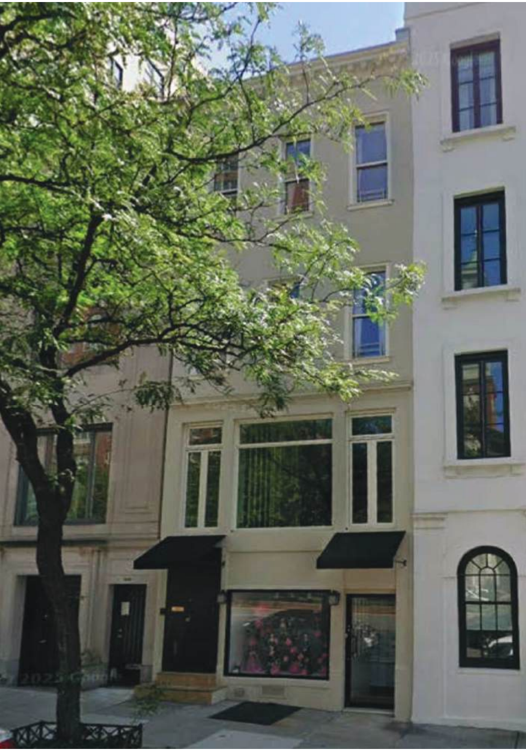
1143 PARK AVENUE CURRENT FRONT FACADE
