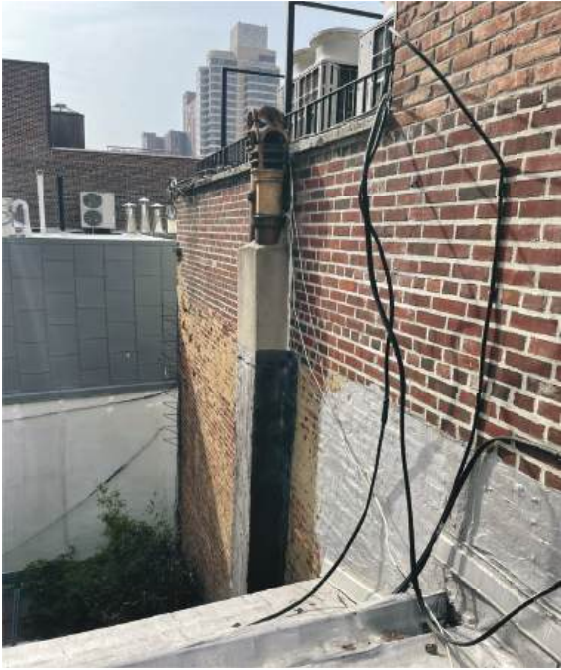
PHOTO 2: SOUTH EAST VIEW (REAR YARD)
