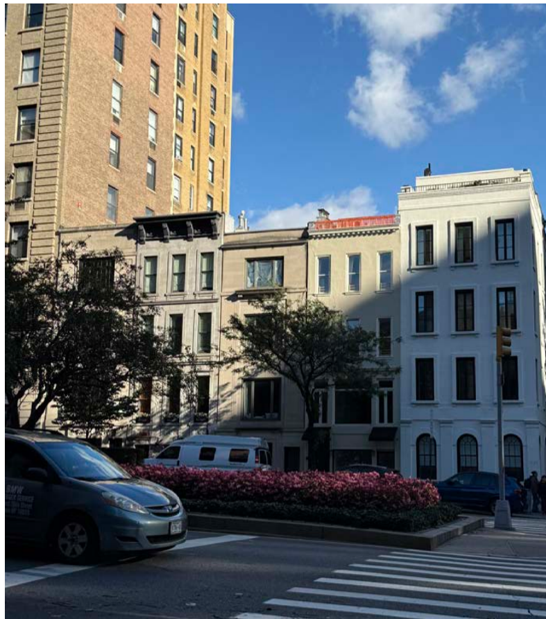
POINT 1: VIEW FROM NW CORNER OF 91ST & PARK
