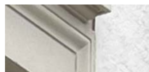
06 HISTORICAL DETAIL BLDG. PHOTO
