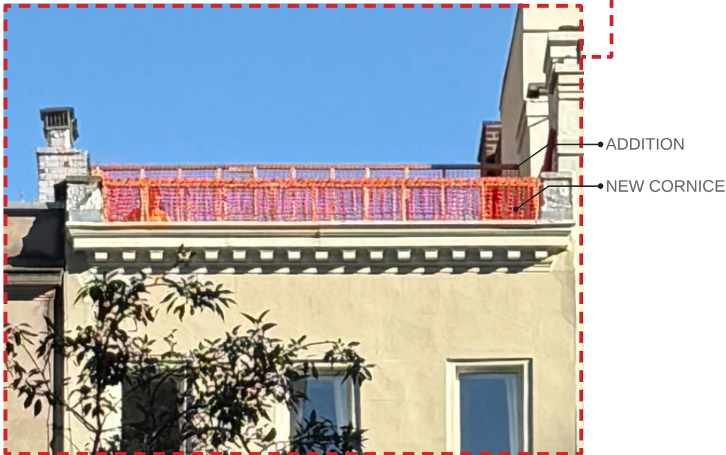
ENLARGED VIEW OF ROOF TOP ADDITION
