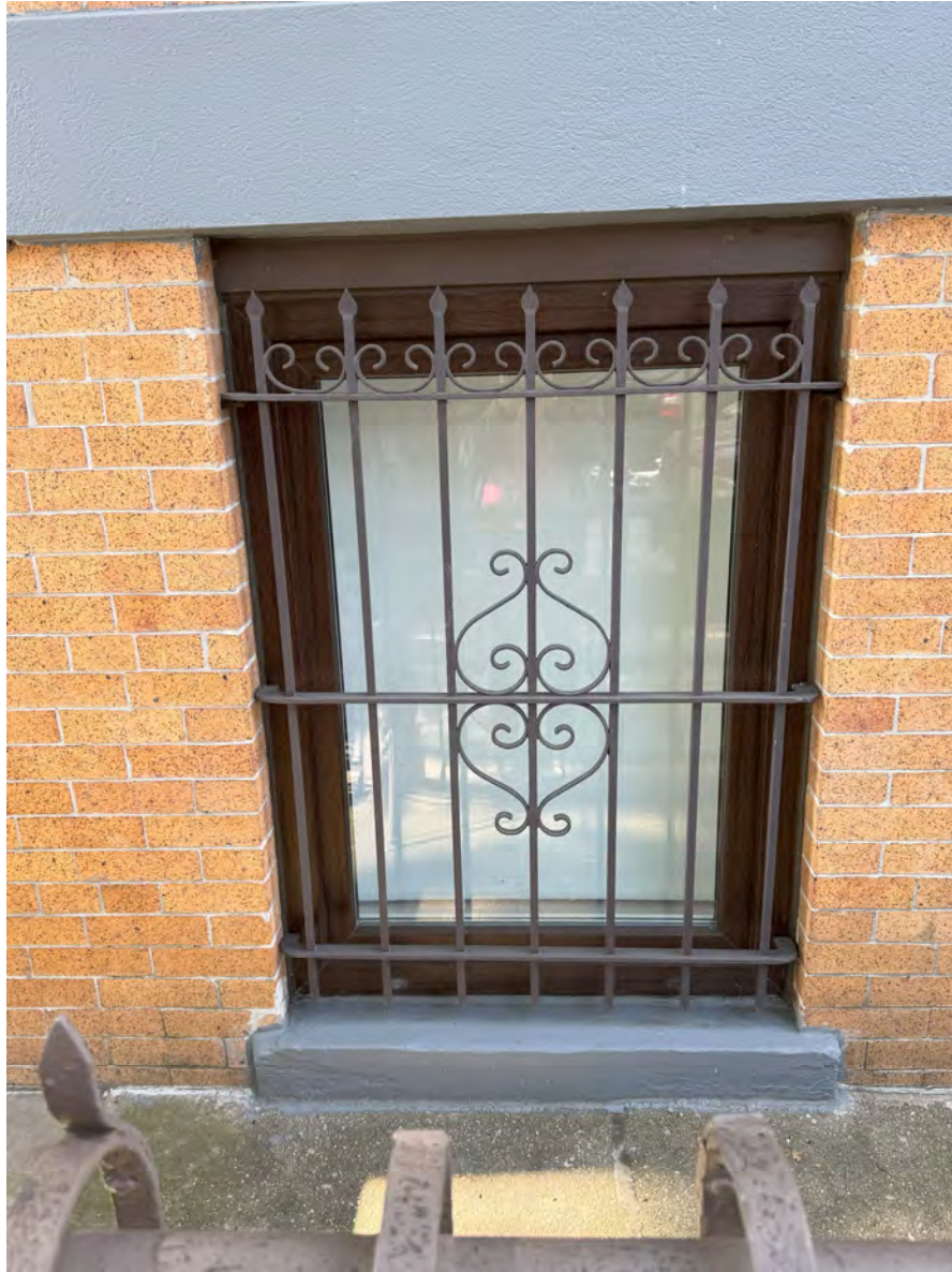
Detail view of original ironwork at new 60 th St. window (9/23/25)
