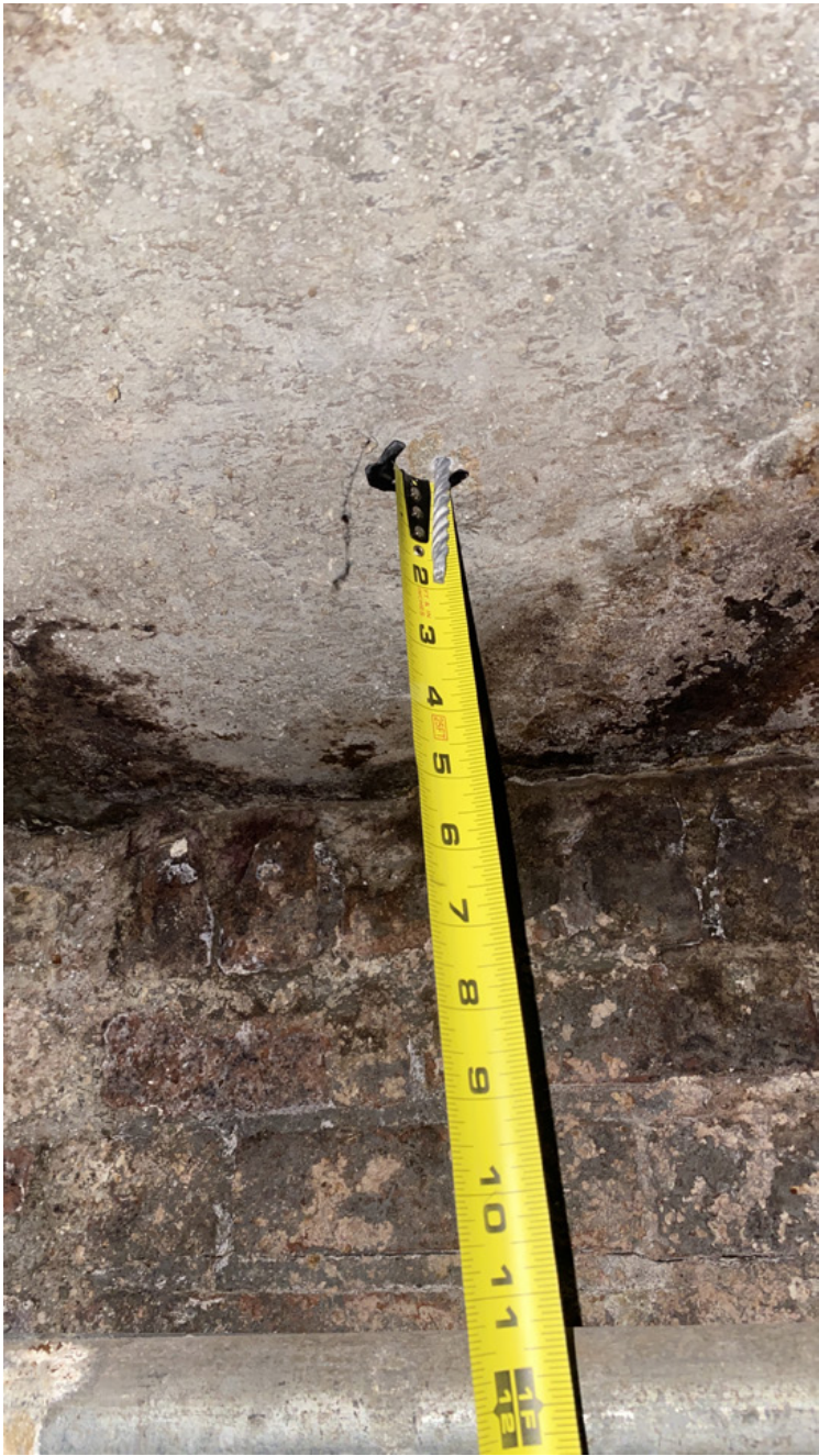
DEPTH PROBE No. 3 = 8" EAST VAULT
