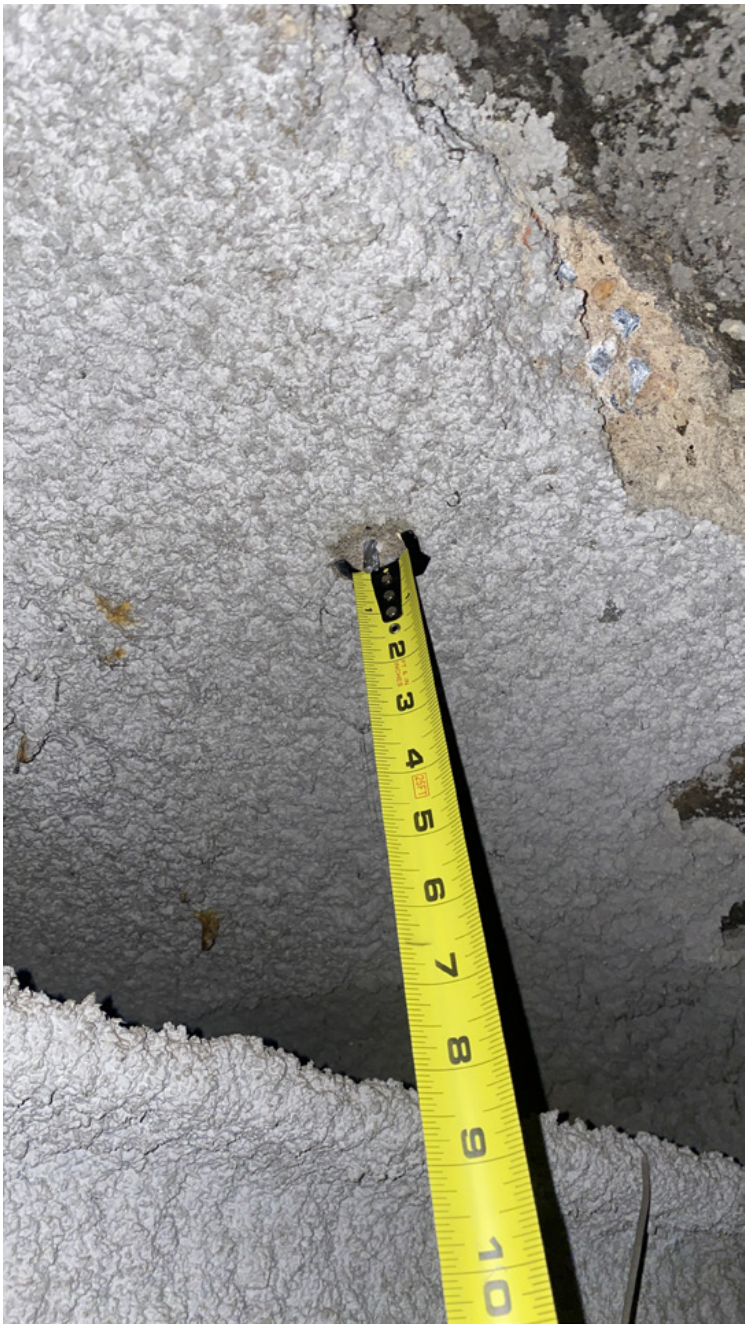
DEPTH PROBE No. 4 = 10" WEST VAULT
