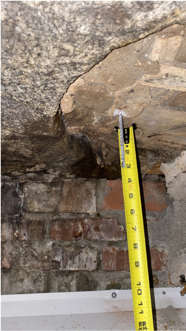
DEPTH PROBE No. 1 = 7.5" EAST VAULT
