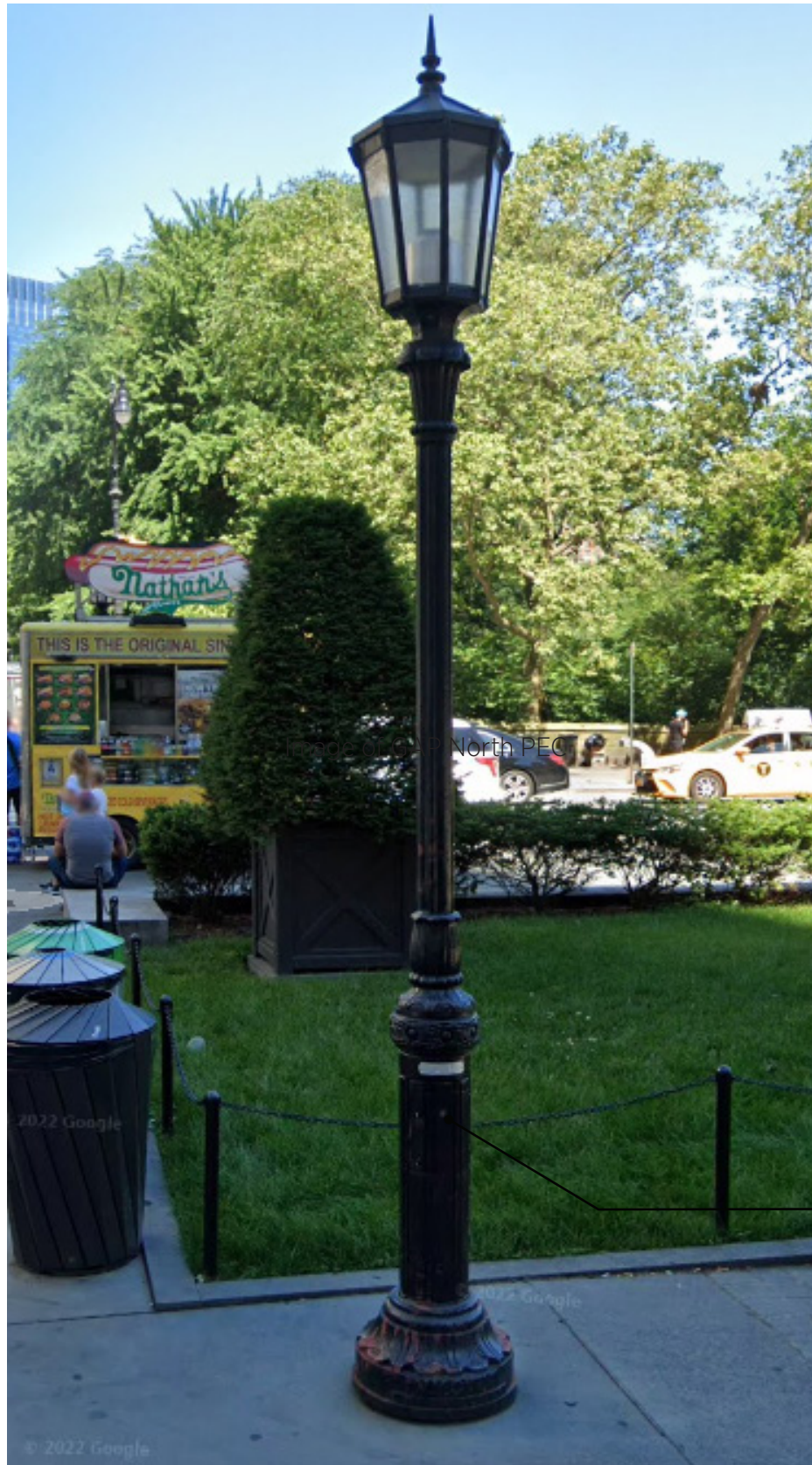
GAP North PEC, Button Photocell no longer acceptable installation
