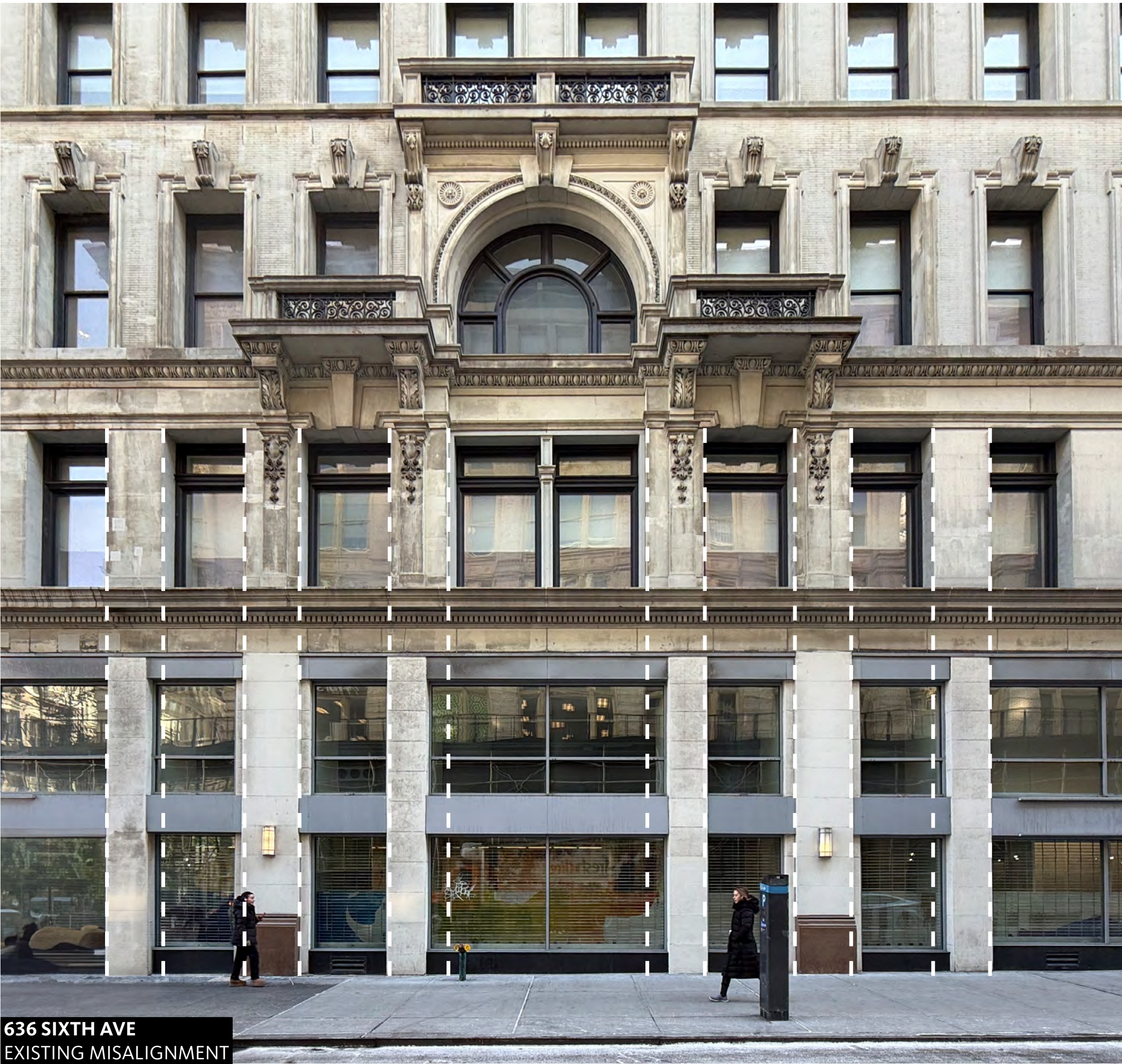
REFERENCING HISTORICAL INFLUENCE BY REALIGNING FLOOR 01 PIER PROPORTIONS TO UPPER LEVELS, INFILLING WITH FULL-HEIGHT STOREFRONT
