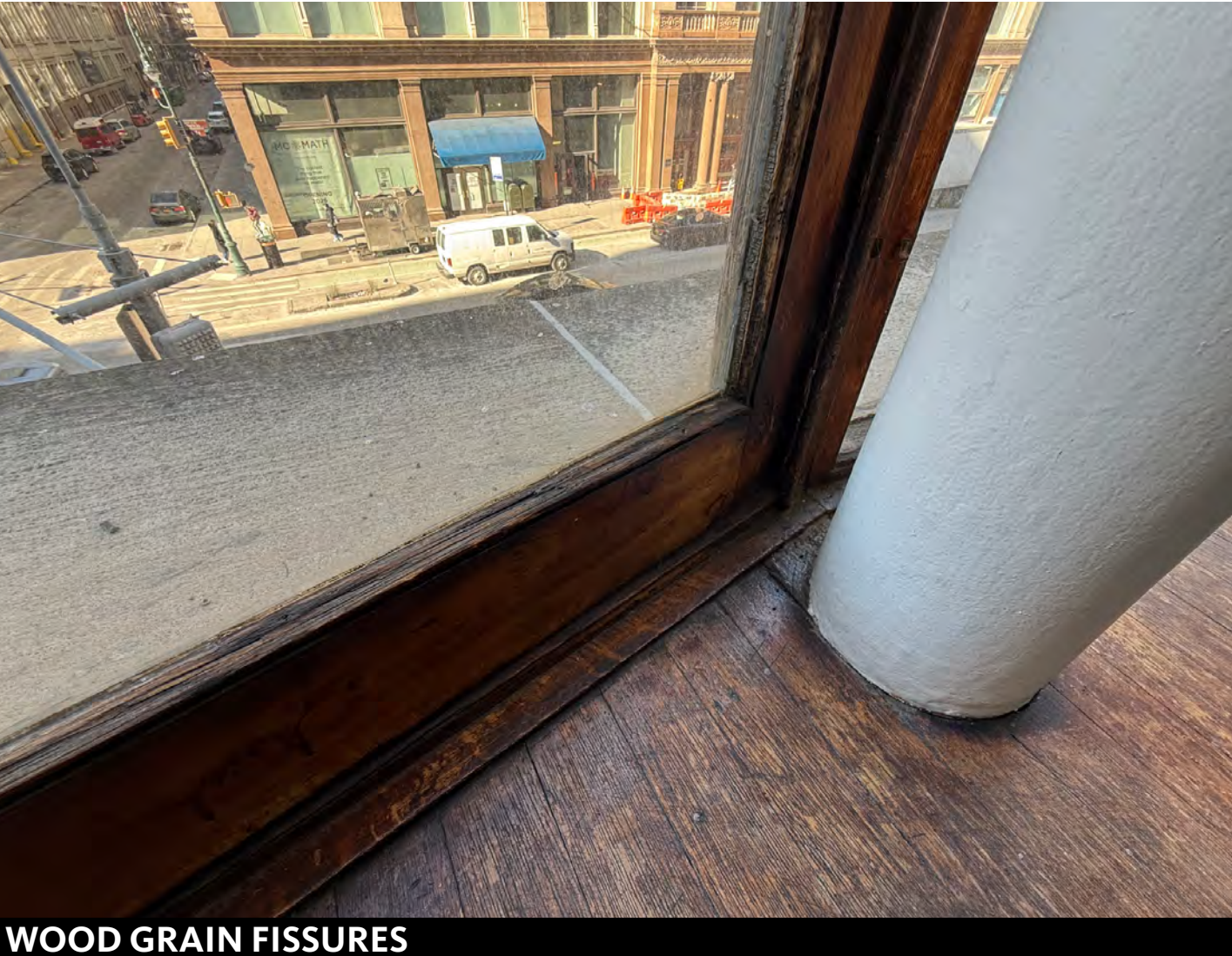
WOOD GRAIN FISSURES
