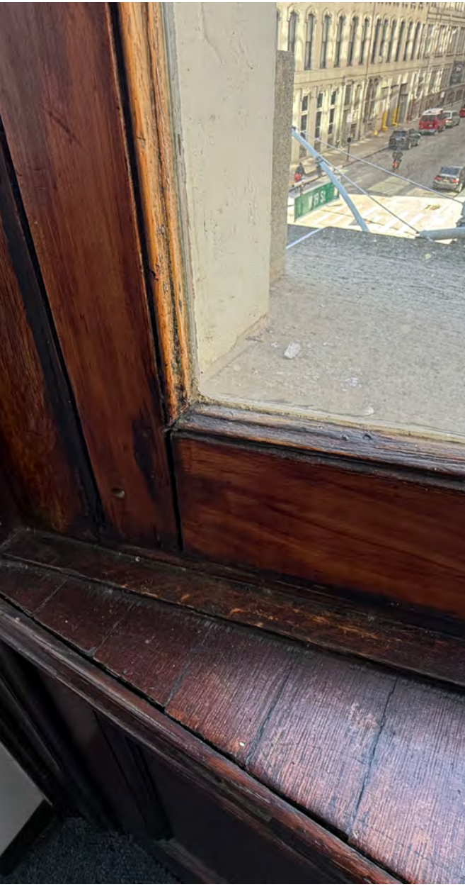
WOOD GRAIN FISSURES
