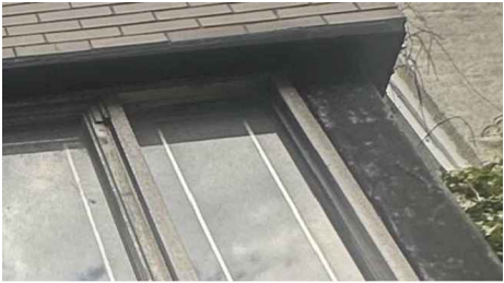
2 STEEL COLUMNS AND LINTELS EXPOSED LPC-05 Scale: N.T.S.
