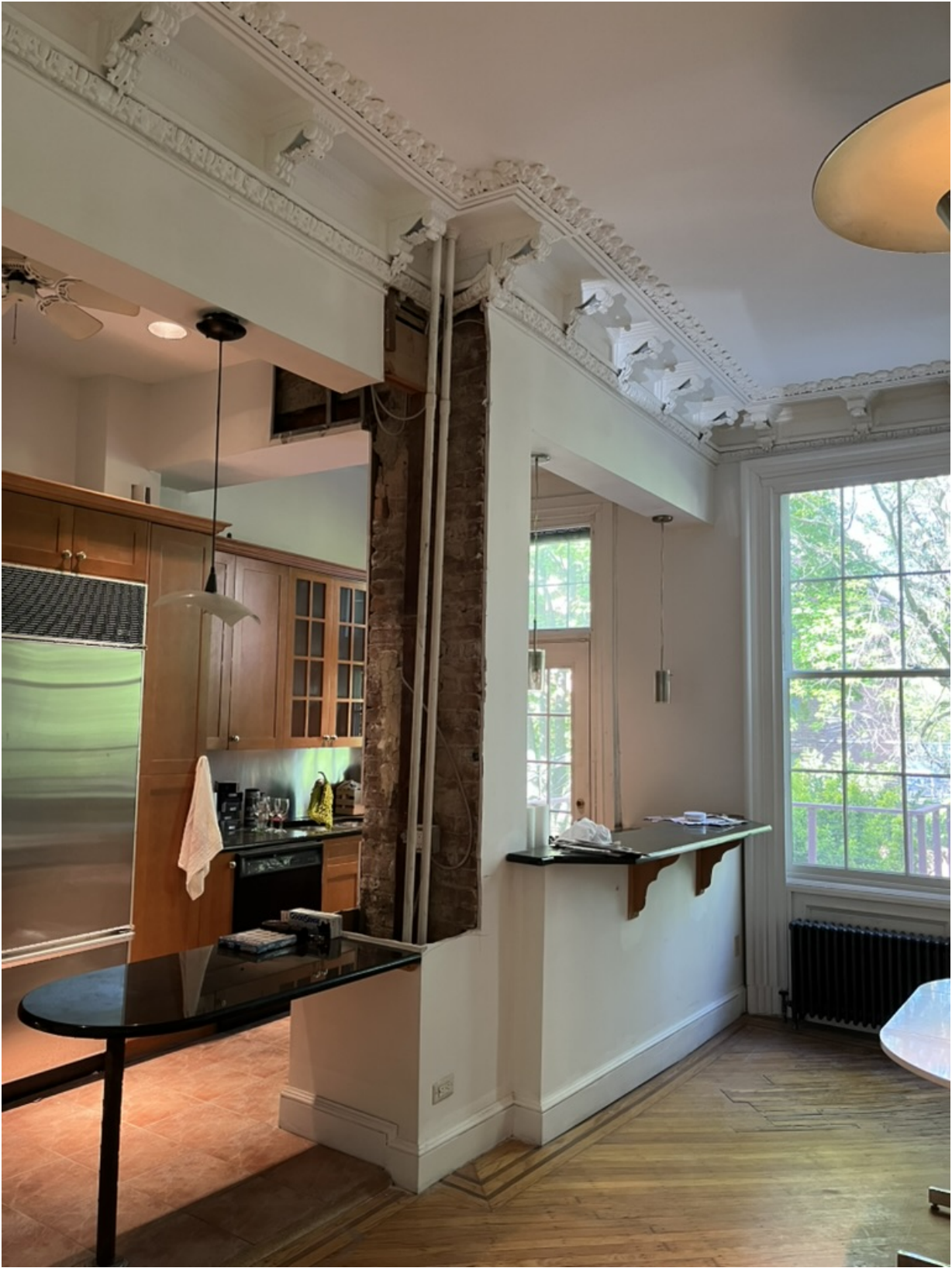
428 CLERMONT AVENUE - EXISTING FIRST FLOOR REAR KITCHEN & DINING EXISTING CONDITION DOCUMENTATION
