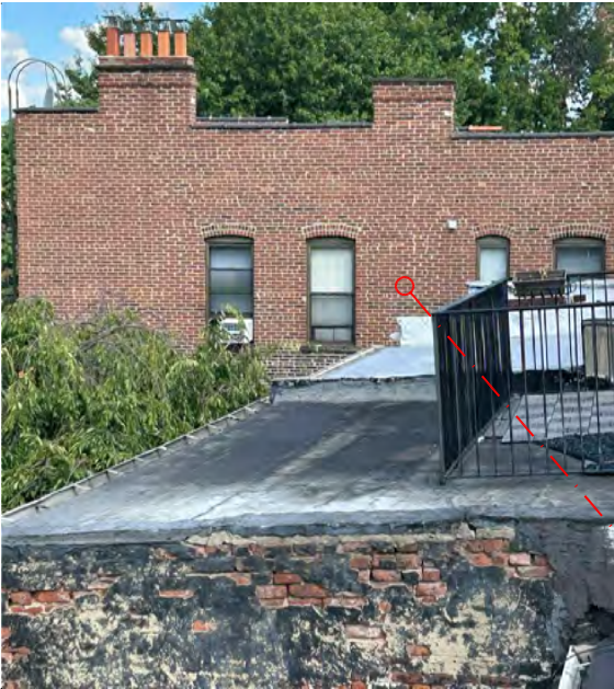
416 CLERMONT AVE REAR WINDOWS 7'-6" HIGH
