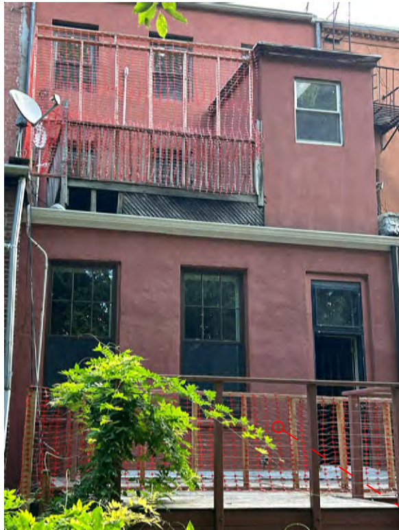
428 CLERMONT AVE REAR WINDOWS 7'-6" HIGH
