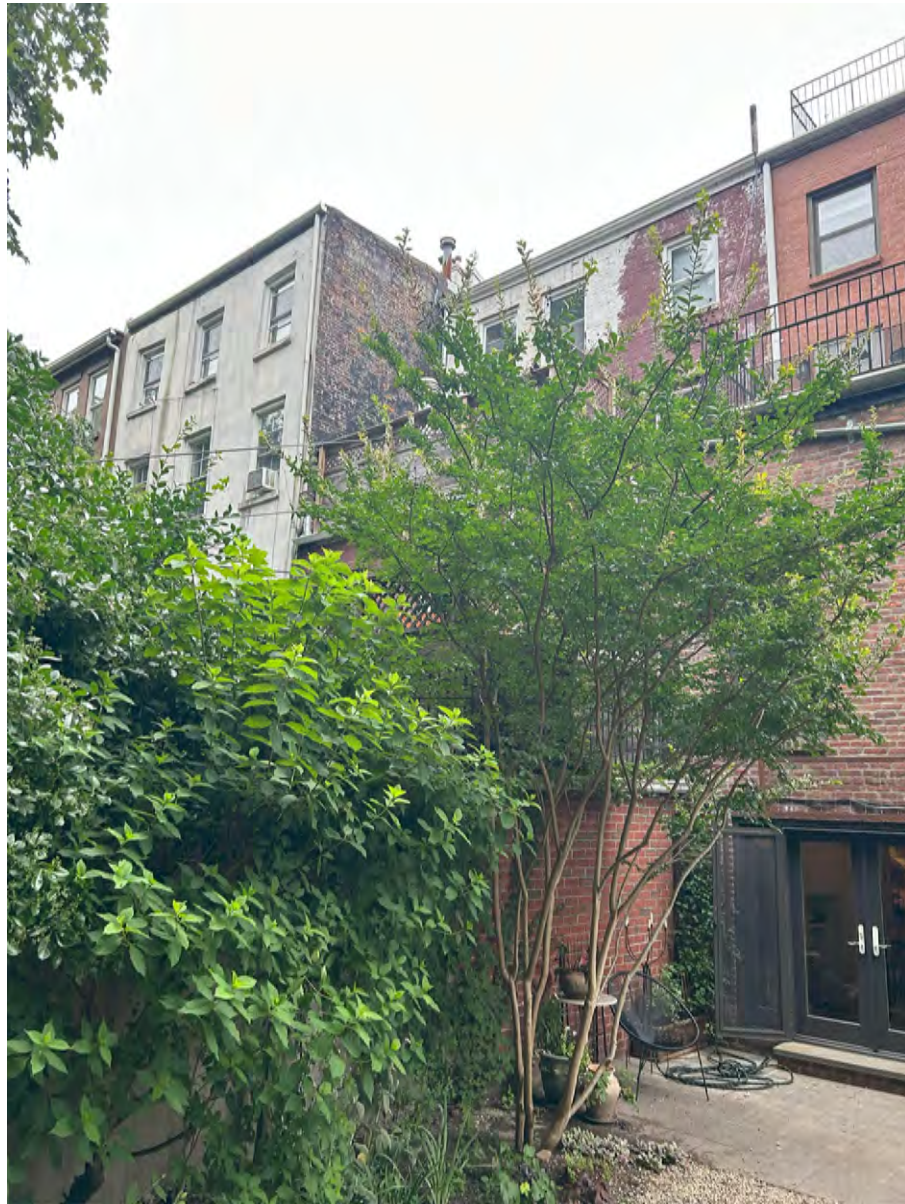
VIEW OF NEIGHBORS FROM REAR YARD (LOOKING NORTH) NTS 03
