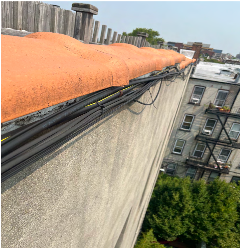
Existing Parapet Wall Conditions
