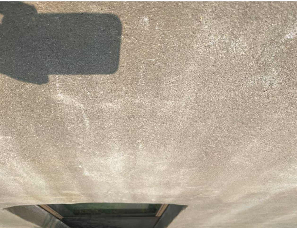
IMG.3._White lines are hairline cracks, which are normal for stucco but do allow rain to pass through to the original brick. The stucco installation is not furred out from the brick masonry wall nor is the lath felt-backed.
