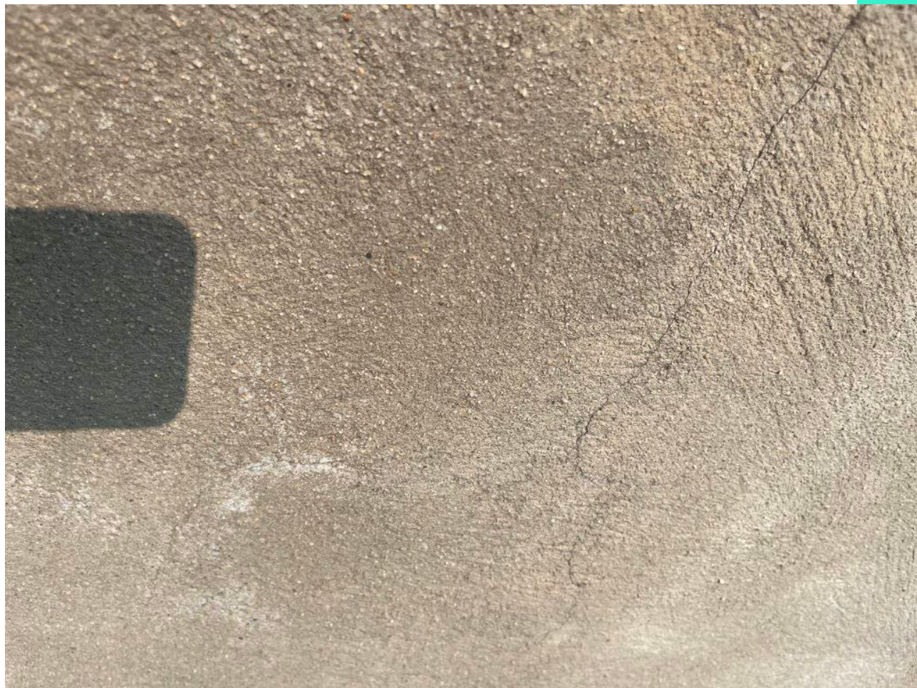
IMG.4._ Larger and smaller hairline cracks in stucco.
