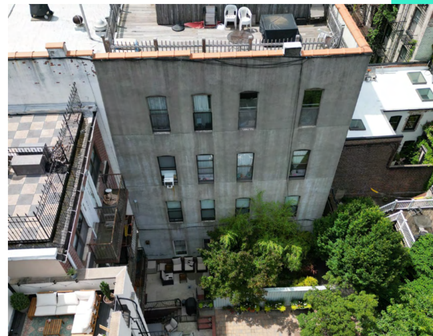
Existing Conditions - East Wall
