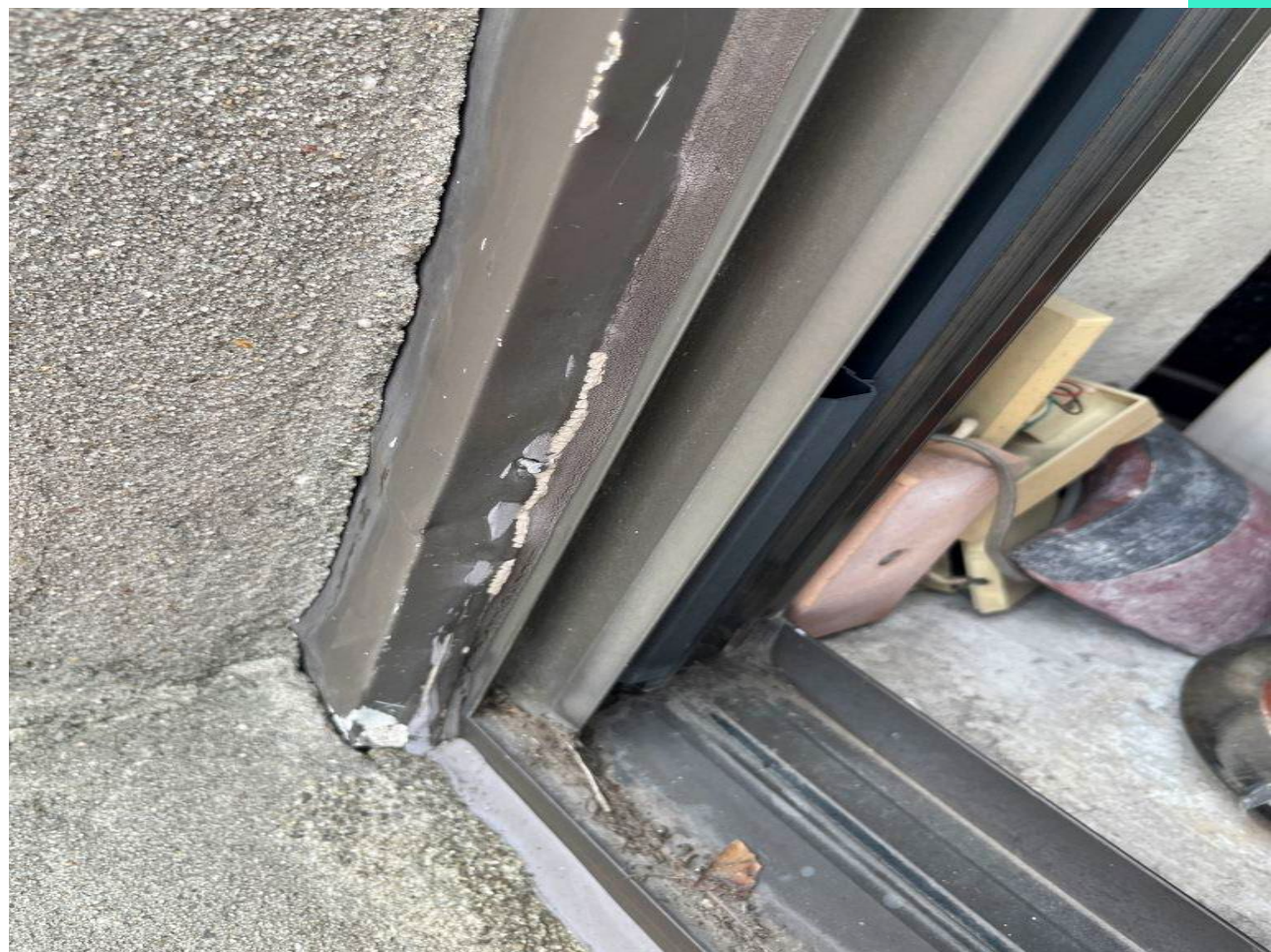
IMG.8._ Stucco is not sealed against the window frame. Stucco was applied after the windows and window panning was installed, probably as an attempt to address widespread weather leaks into the building.
