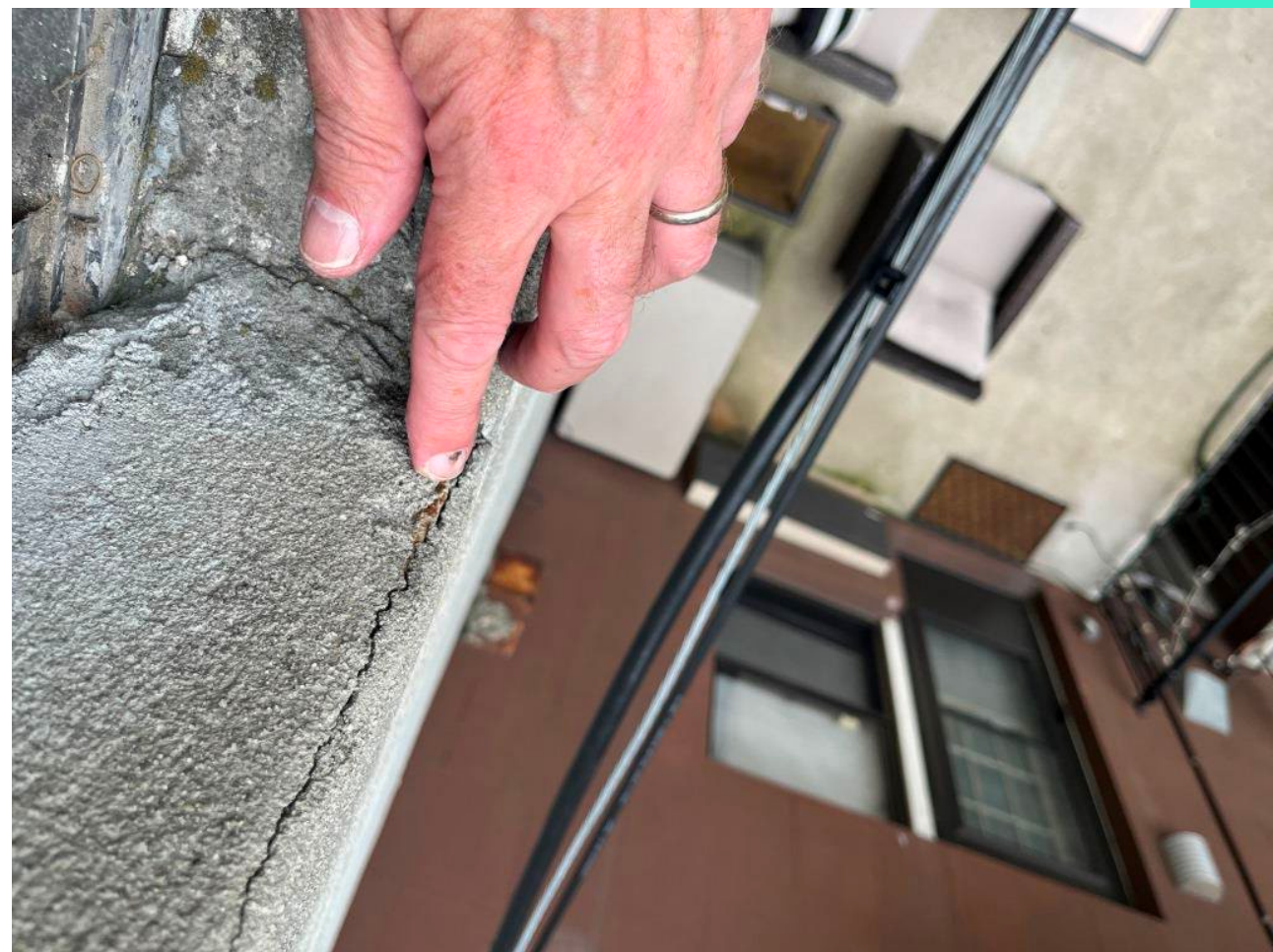
IMG.6._ Hairline stucco crack at the window opening. Finger is pointing to the jamb condition; orientation of the photo is looking down.
