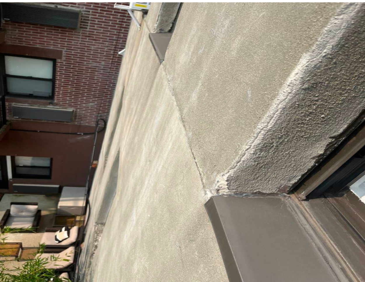
IMG.5._Hairline crack in stucco at window opening. Hairline cracks at this outside condition are common because the stucco lath ends at the perimeter of the masonry opening without turning in and returning to the window.
