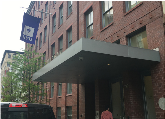
8. WILF HALL - 139 MACDOUGAL STREET
