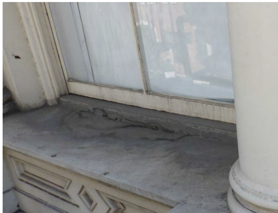
WATER TABLES ARE BACK-PITCHED RESULTING IN PONDING AND WATER INFILTRATION
