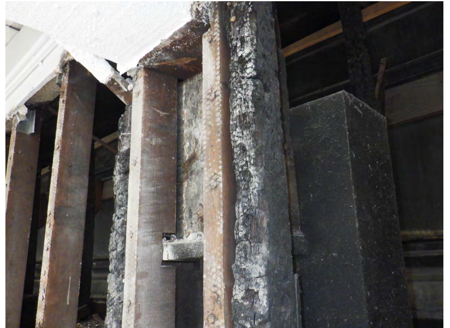
CHARRED STUD POSTS BEHIND EXISTING CORNICE
