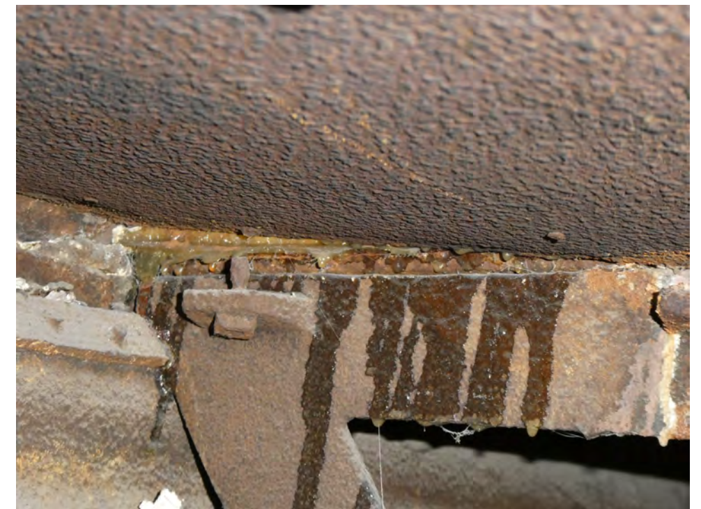
WATER TABLES ARE BACK-PITCHED RESULTING IN PONDING AND WATER INFILTRATION
