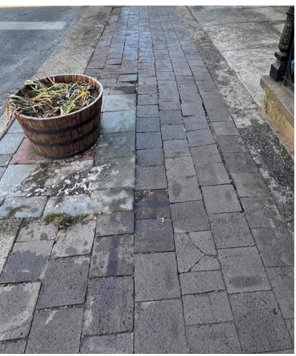
2 - St. Mark's - Original, Uneven, Cracked, Broken, Existing Pavers on St. Mark's (2025)
