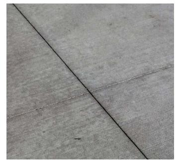
Sidewalk Pavement: Landmarks Gray Concrete w/ Sawn Joints - 24" Square Sawn Joint Pattern
