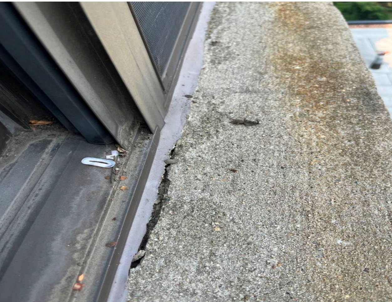
IMG.7._Stucco at windowsills is not sealed where it meets the window frame. Stucco is also reinforced where applied to the sills.
