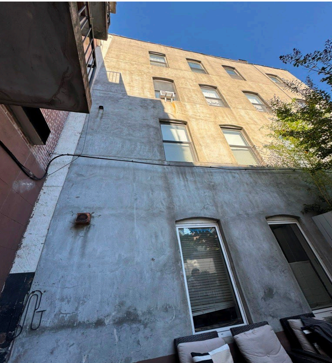
IMG.1._View of stucco cladding at east-facing wall. On the left is the rear elevation of the neighboring building.
