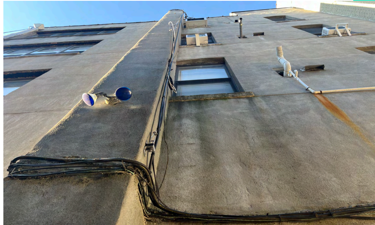
IMG.2._View of stucco cladding at north wall. Although stucco is reinforced with metal lath, it has developed non-structural hairline cracks, reducing the stucco's ability to prevent water penetration into the building's exterior masonry walls.
