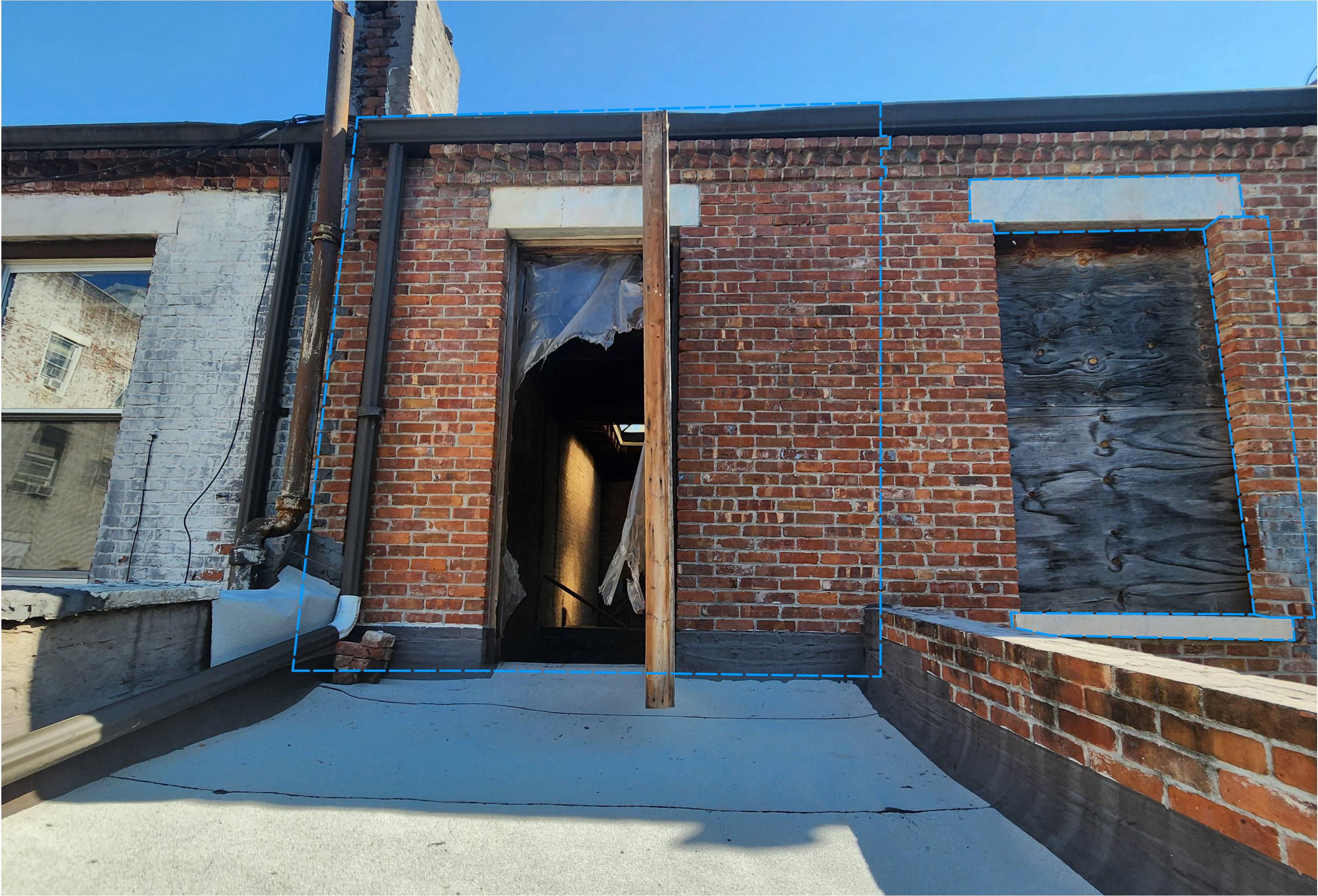
3. LOOKING FROM ROOFTOP OF THE ELL TO THE PORTION OF THE EXISTING CONDITIONS TO BE REMOVED TO ACCOMODATE FOR THE NEW EXTENSION - STONE LINTEL AND WINDOW SILL TO BE CAREFULLY REMOVED, SAVED AND REUSED FOR NEW OPENING AT NEW EXTENSION
